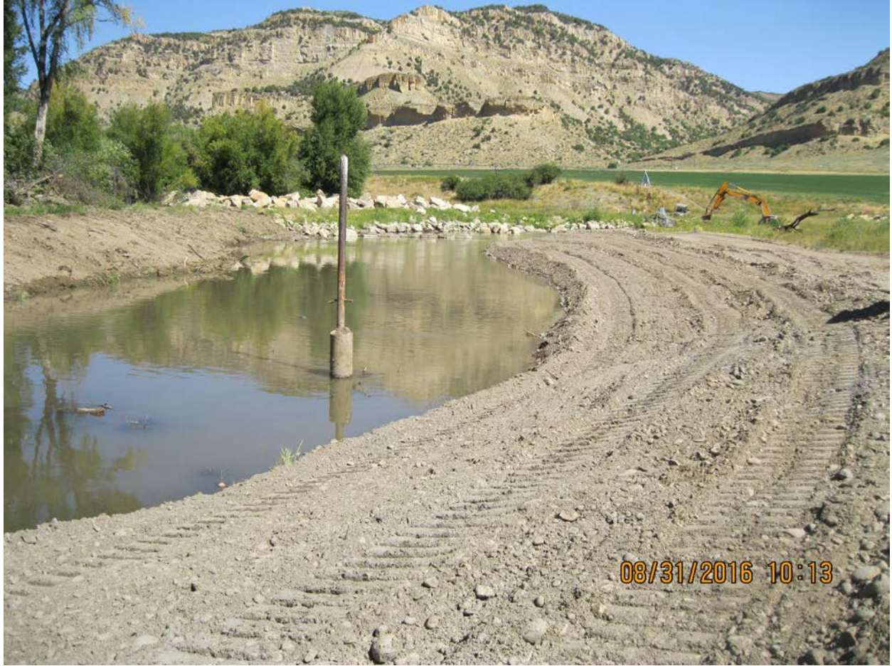
Looking north. Channel stabilization work being performed.
