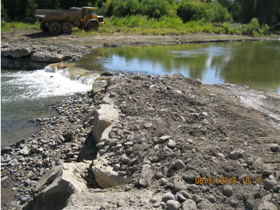
Low water crossing access to west side of river.
