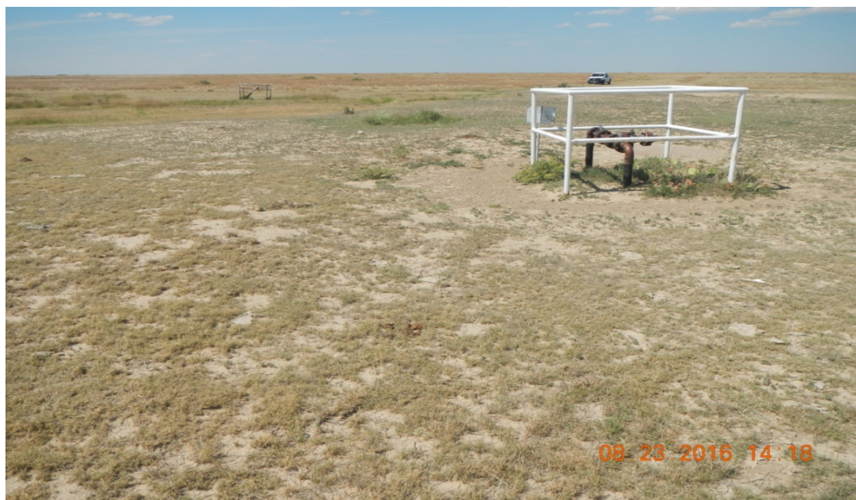
photo 4: South side of the location facing north. The pipe riser has not been removed.
