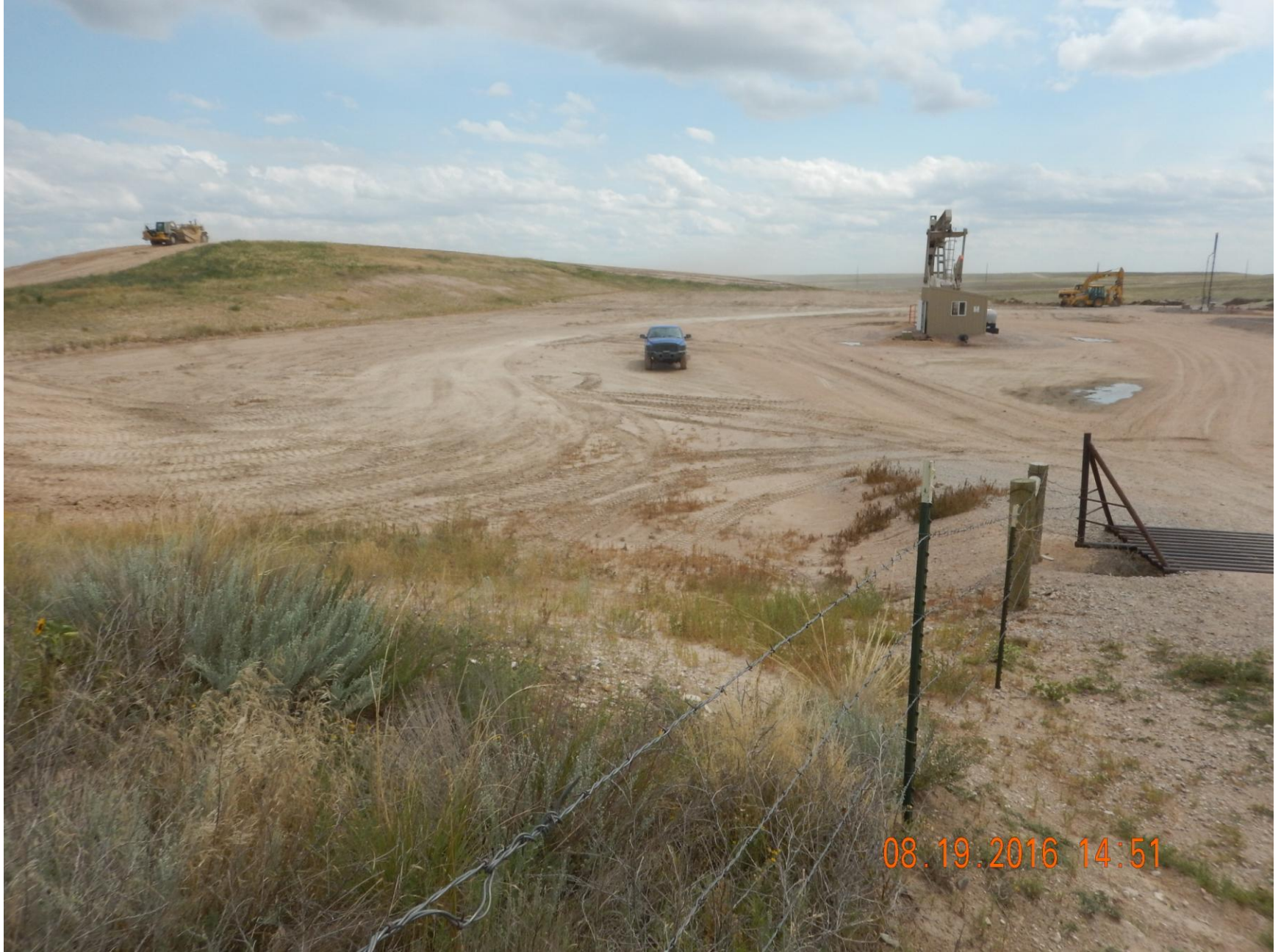
Figure 6: Photo taken from the north end of the location, facing south. Photo shows interim reclamation in process.
