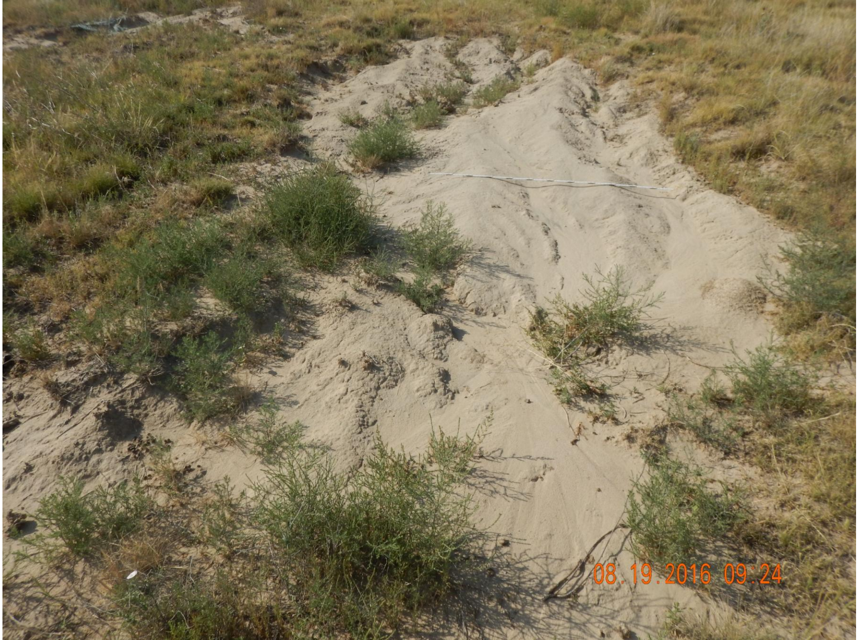
Figure 4: Photo taken from the location. Photo shows large bare areas on location where erosion is occurring. 6' measuring stick for reference.
