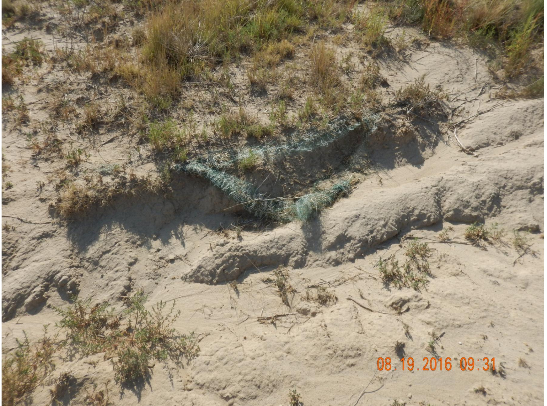
Figure 7: Photo taken from the location. Photo shows large bare areas on location where erosion is occurring. Photo also shows remnants of a sediment control blanket no longer in proper functioning condition, and is now debris.
