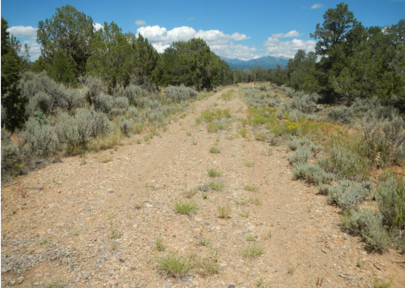
Photo 10. View of access road from near the access entrance facing northward.
