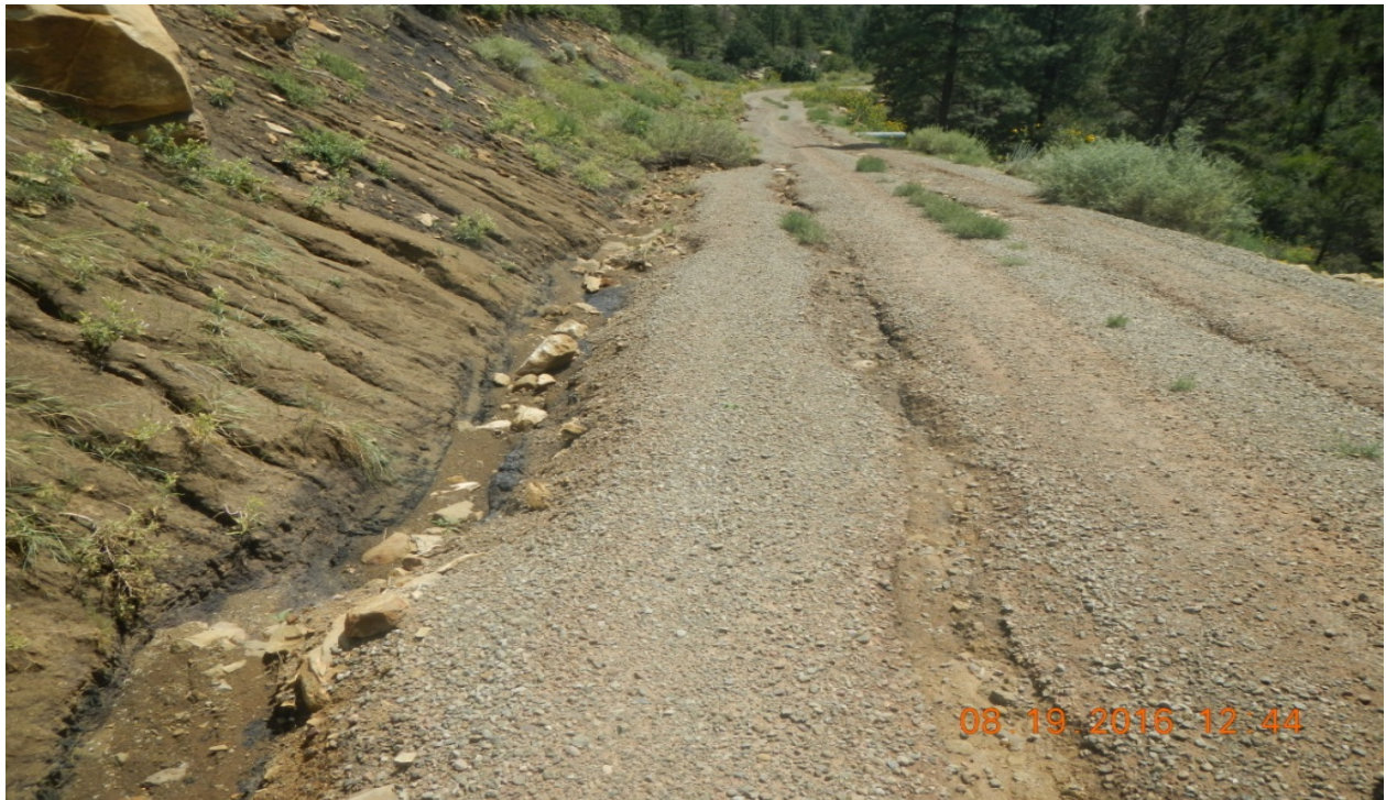
photo 2: Facing southwest along the main access road. Stormwater is being down the road causing erosion on the road. The cut slope is not stabilized and there are signs of erosion occurring.
