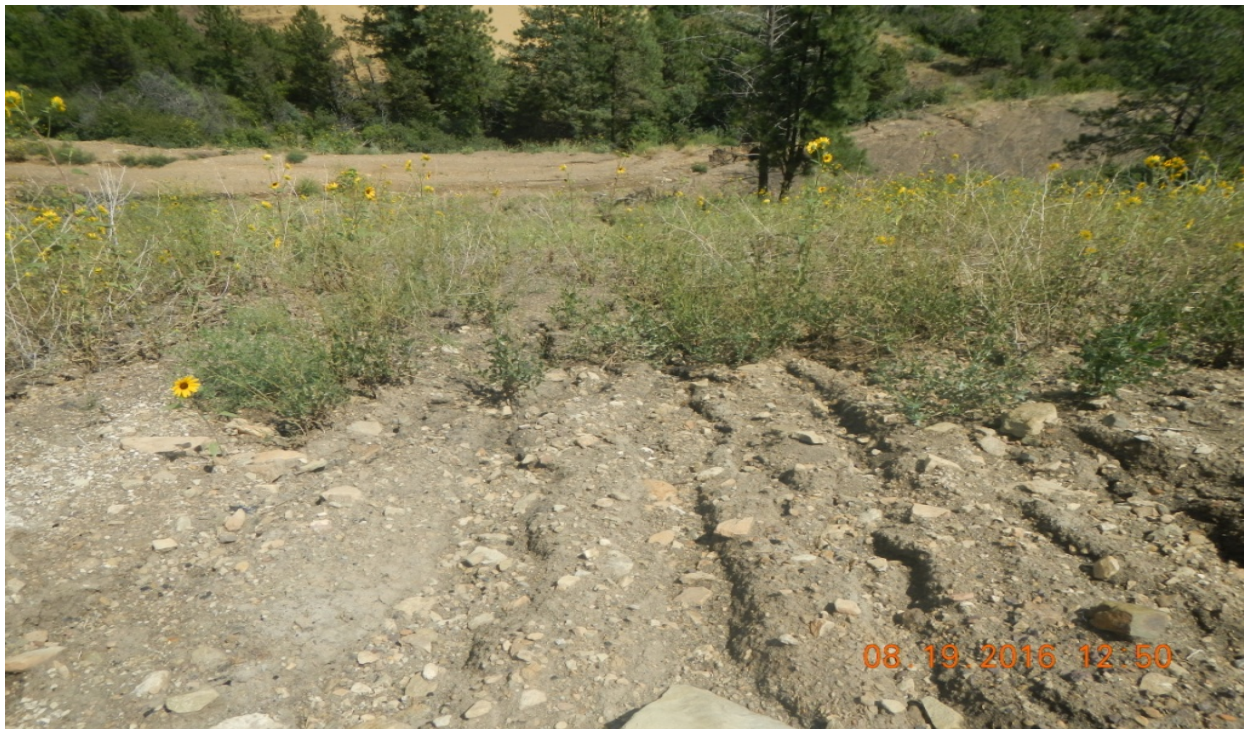
photo 10: Facing east off the fill slope. There is erosion occurring down off the slope.
