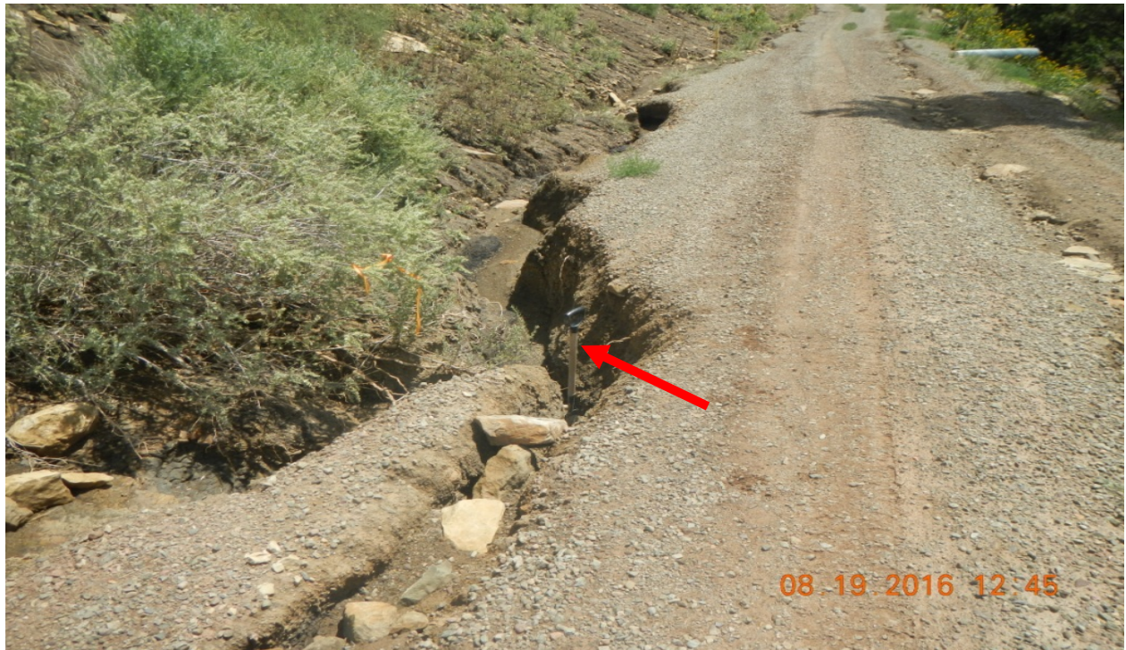
photo 3: Erosion occurring along the road has created a 3 ½ foot hole as indicated by the shovel which red arrow points to.
