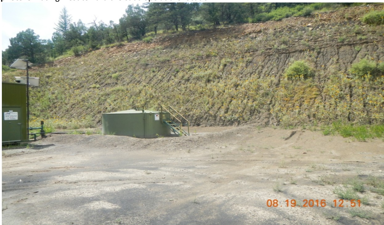
photo 6: Stormwater run-on is causing erosion along the cut slope.
