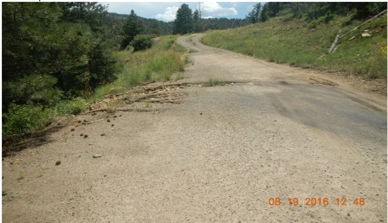
photo 4: Stormwater is flowing across the access road at this point causing erosion across and along the fill slope of the access road.
