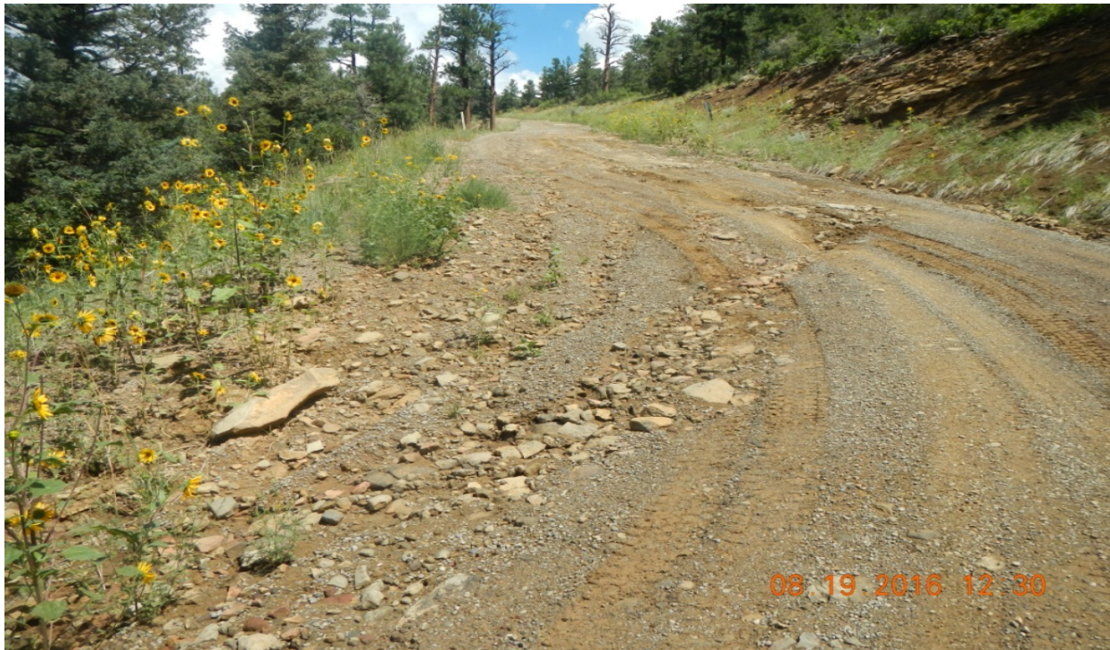
photo 5: The main road switches back to the northeast at this point. There are signs of erosion occurring on the road.
