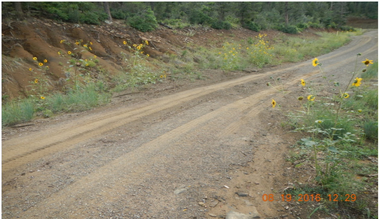
photo 4: Stormwater is flowing across the access road at this point causing erosion across and along the fill slope of the access road. There are erosion channels along the cut slope which is not stabilized.
