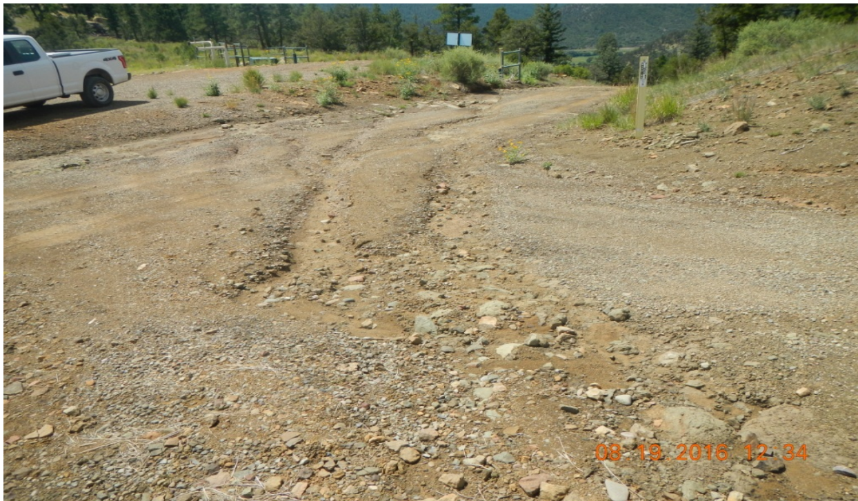
photo 8: Facing back toward the southwest along the main access road. There are signs of stormwater flow causing erosion down the road.
