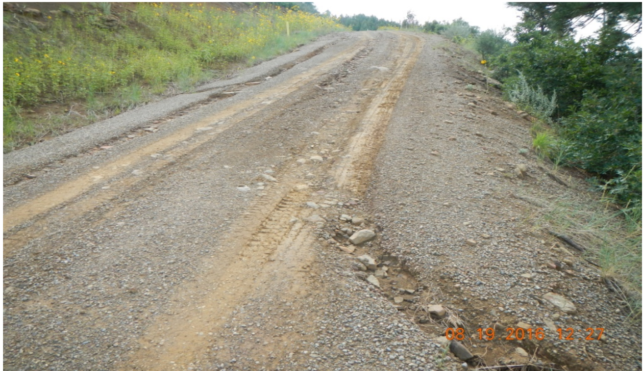
photo 1: Facing south along the main access road to the location. There are signs of erosion occurring along the road.
