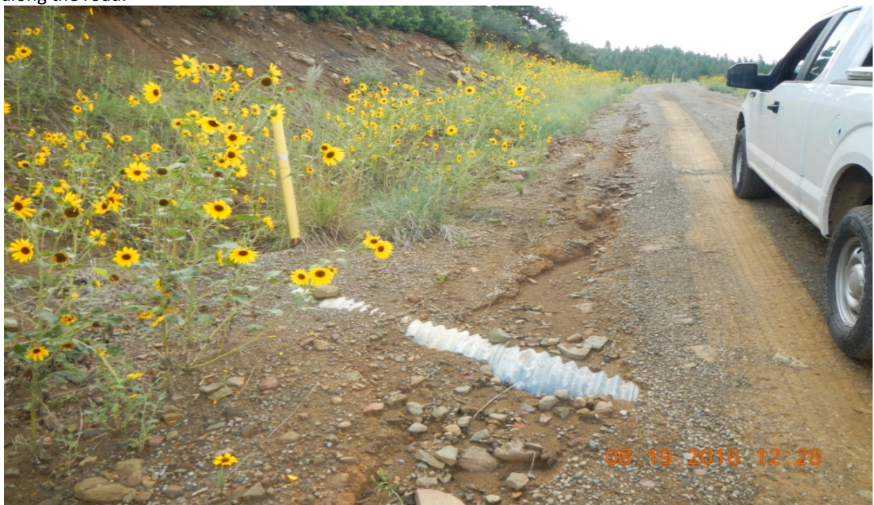
photo 2: Stormwater is not being diverted to the culvert and is running down the road causing erosion.
