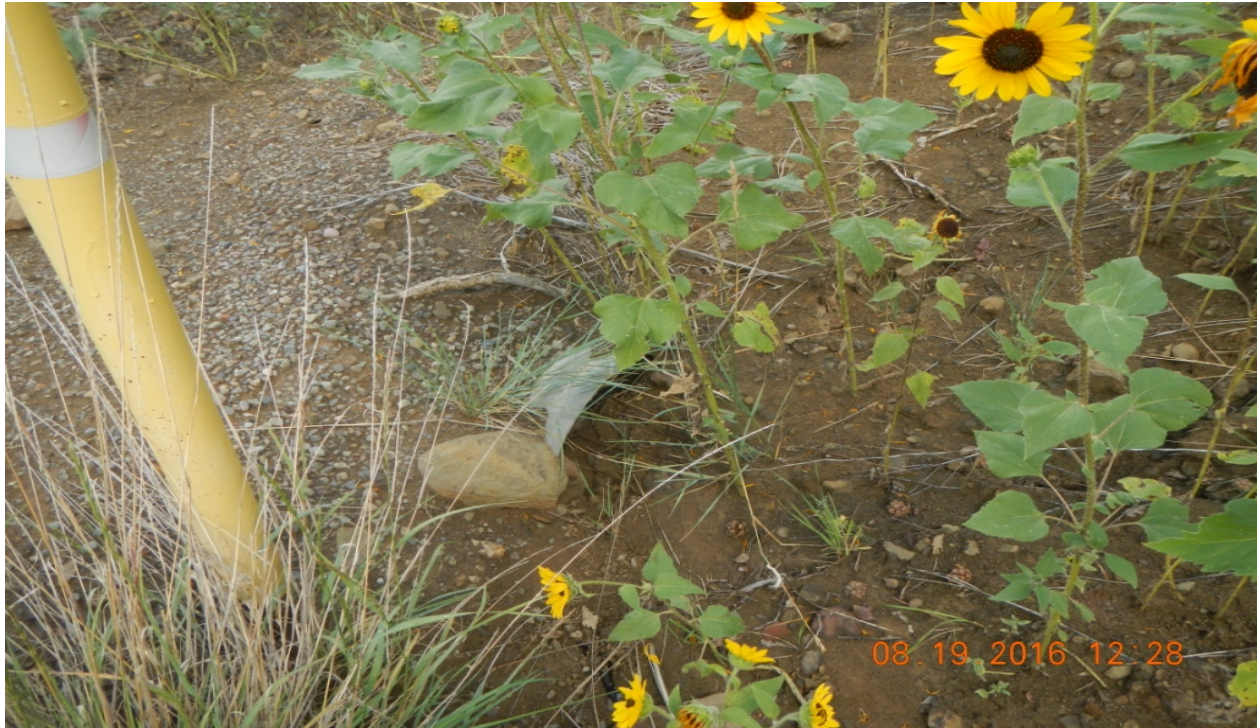
photo 3: The culvert along the road is filled in with sediment. Approximate Lat/Long:37.1637,-104.9130.
