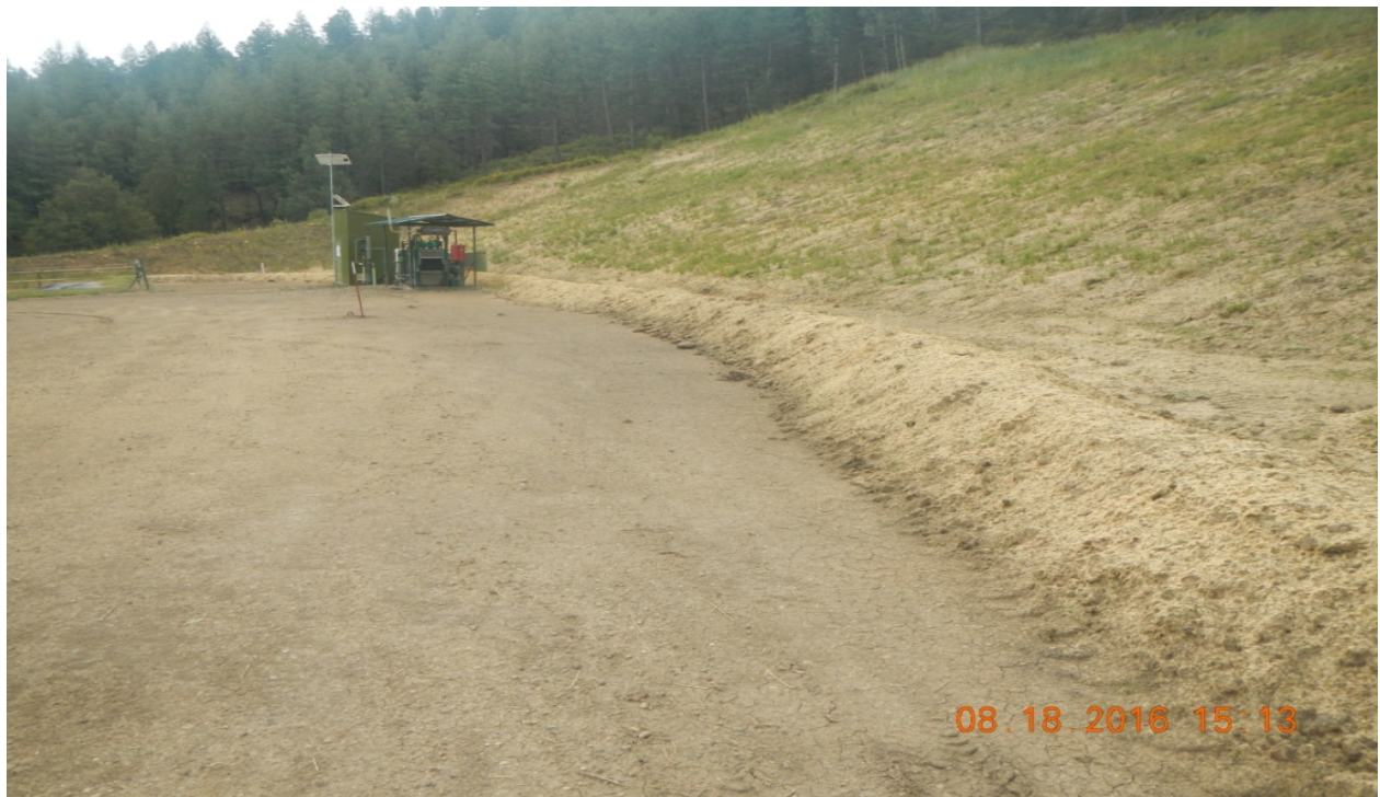
photo 4: The south slope has been hydro mulched/seeded and a berm has been installed.
