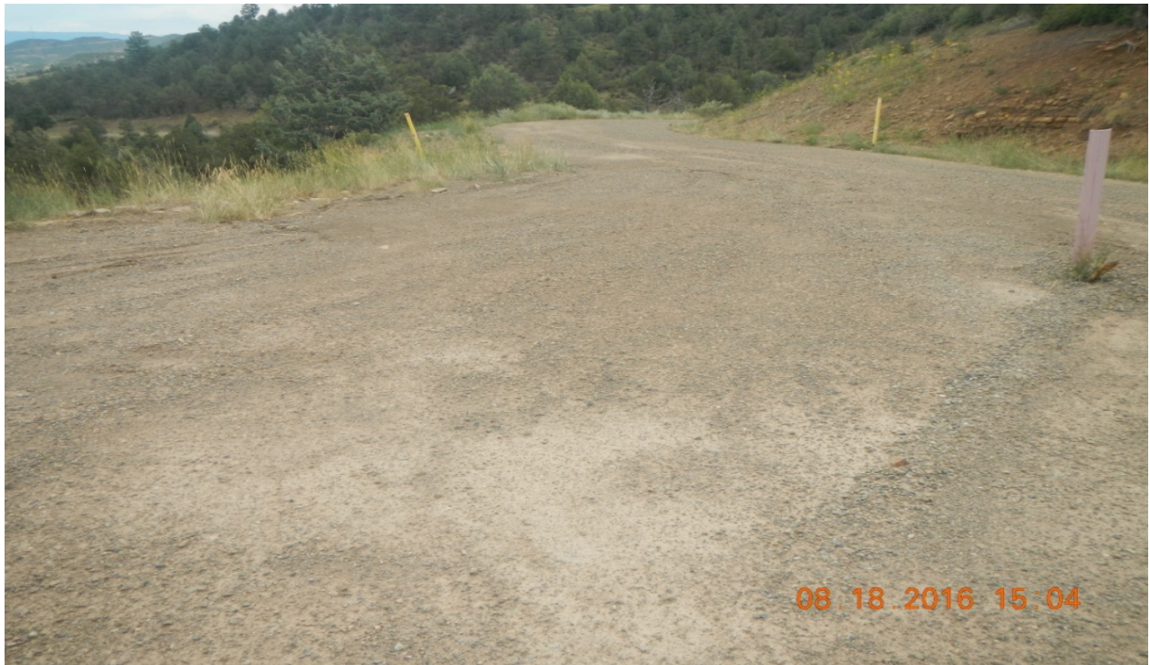
photo 3: Facing southeast at the location where erosion issues were repaired.
