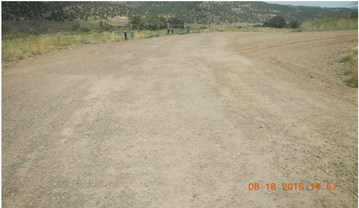
photo 1: Facing northeast along the access road where erosion issues were repaired.
