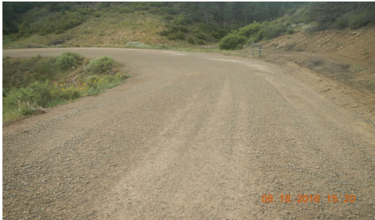
photo 6: Facing south along the access road where erosion issues were repaired.
