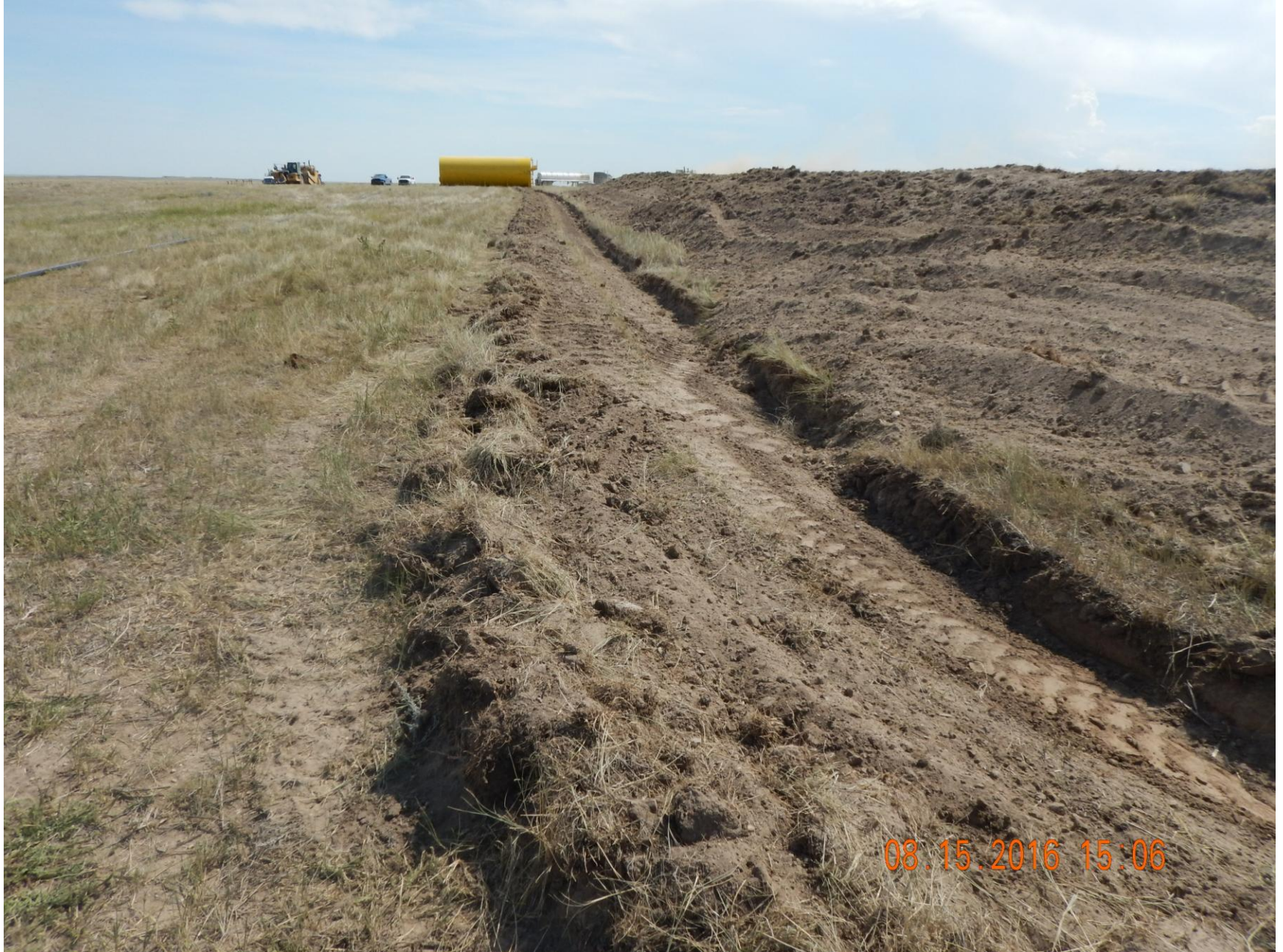
Figure 4: Photo taken from the northeast corner of the location, facing south. Photo shows stormwater and sediment control ditch BMP on the (partial) eastern perimeter of the location.
