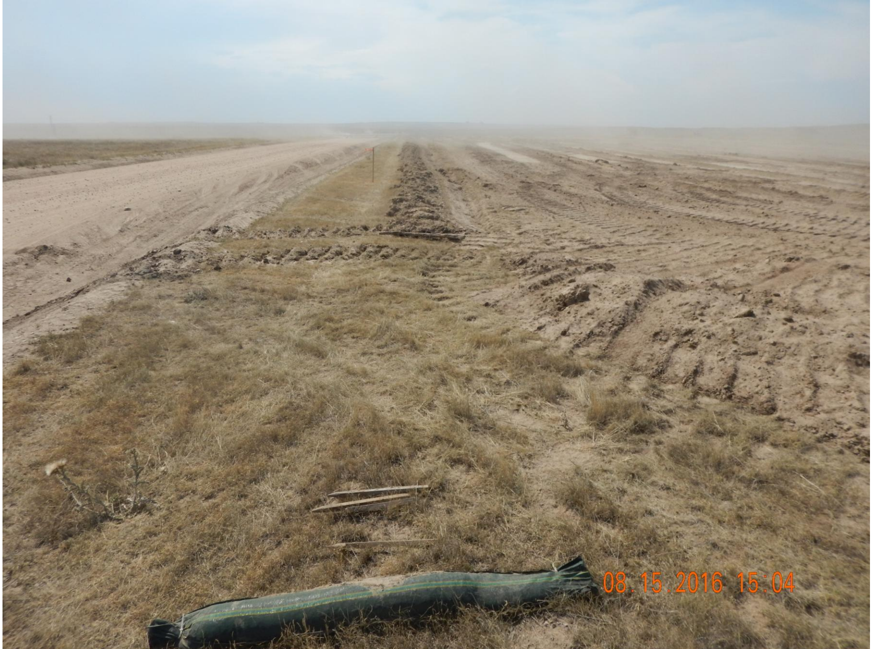
Figure 1: Photo taken from the southeast corner of the location, facing west. Photo shows stormwater and sediment control ditch BMP on the southern perimeter of the location.
