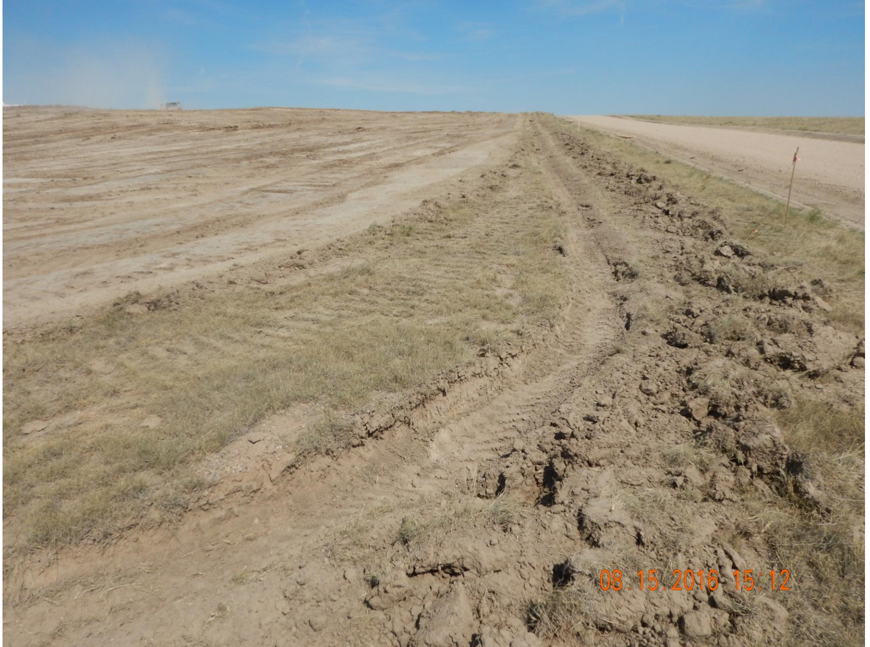
Figure 10: Photo taken from the southwest corner of the location, facing east. Photo shows stormwater and sediment control ditch BMP on the southern perimeter of the location.
