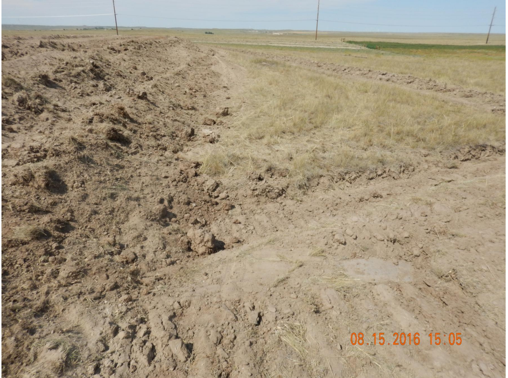
Figure 3: Photo taken from the east end of the location, facing north. Photo shows stormwater and sediment control ditch BMP only partially on the eastern perimeter of the location.
