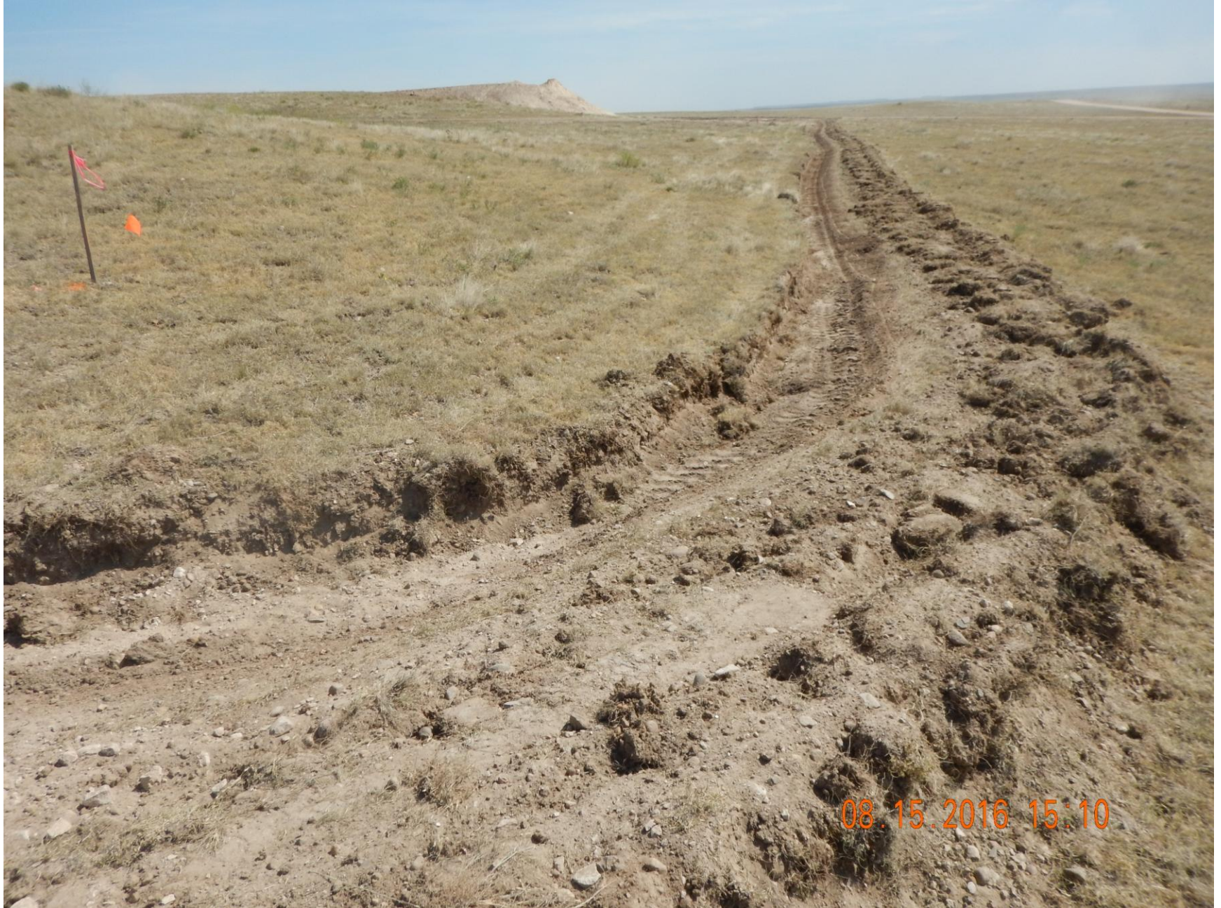
Figure 8: Photo taken from the northwest corner of the location, facing south. Photo shows stormwater and sediment control ditch BMP on the western perimeter of the location.
