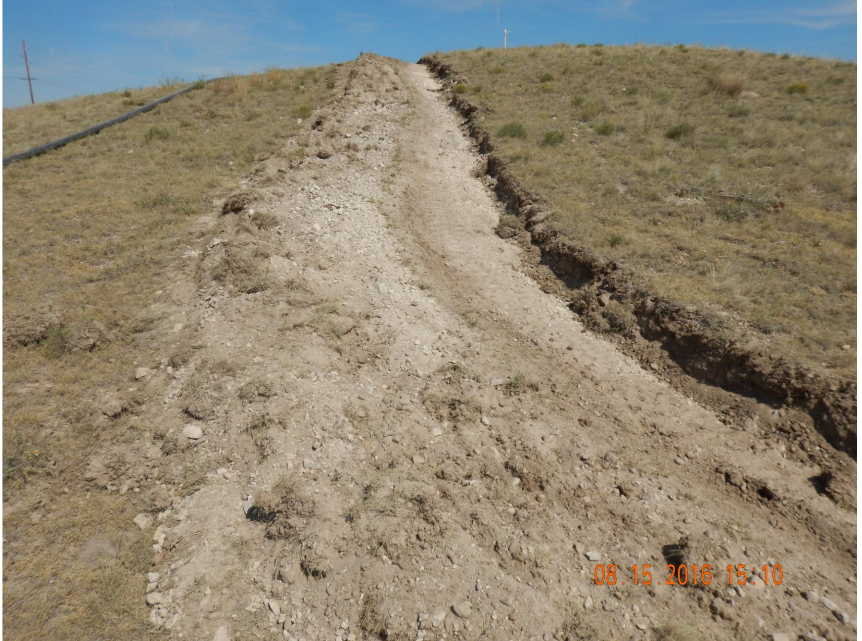
Figure 9: Photo taken from the northwest corner of the location, facing east. Photo shows stormwater and sediment control ditch BMP on the northern perimeter of the location.
