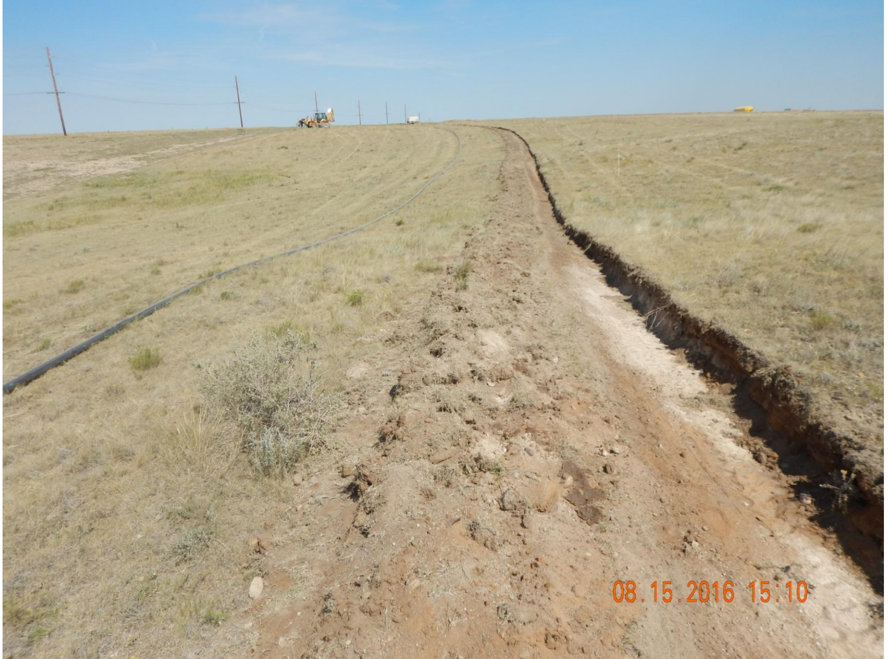
Figure 6: Photo taken from the northwest corner of the location, facing east. Photo shows stormwater and sediment control ditch BMP on the northern perimeter of the location.
