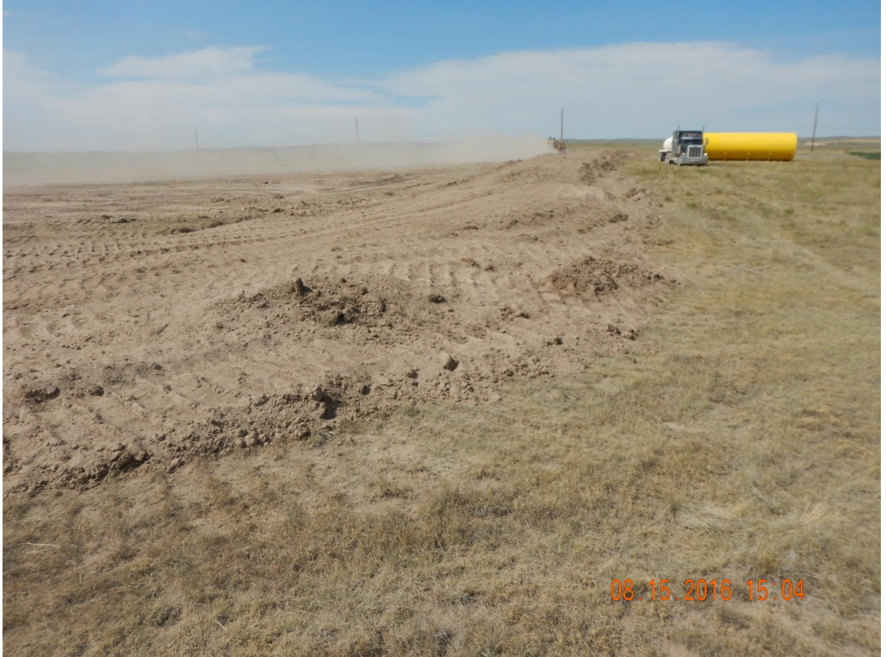
Figure 2: Photo taken from the southeast corner of the location, facing north. Photo shows stormwater and sediment control BMPs missing partially on the eastern perimeter of the location and topsoil stockpile.
