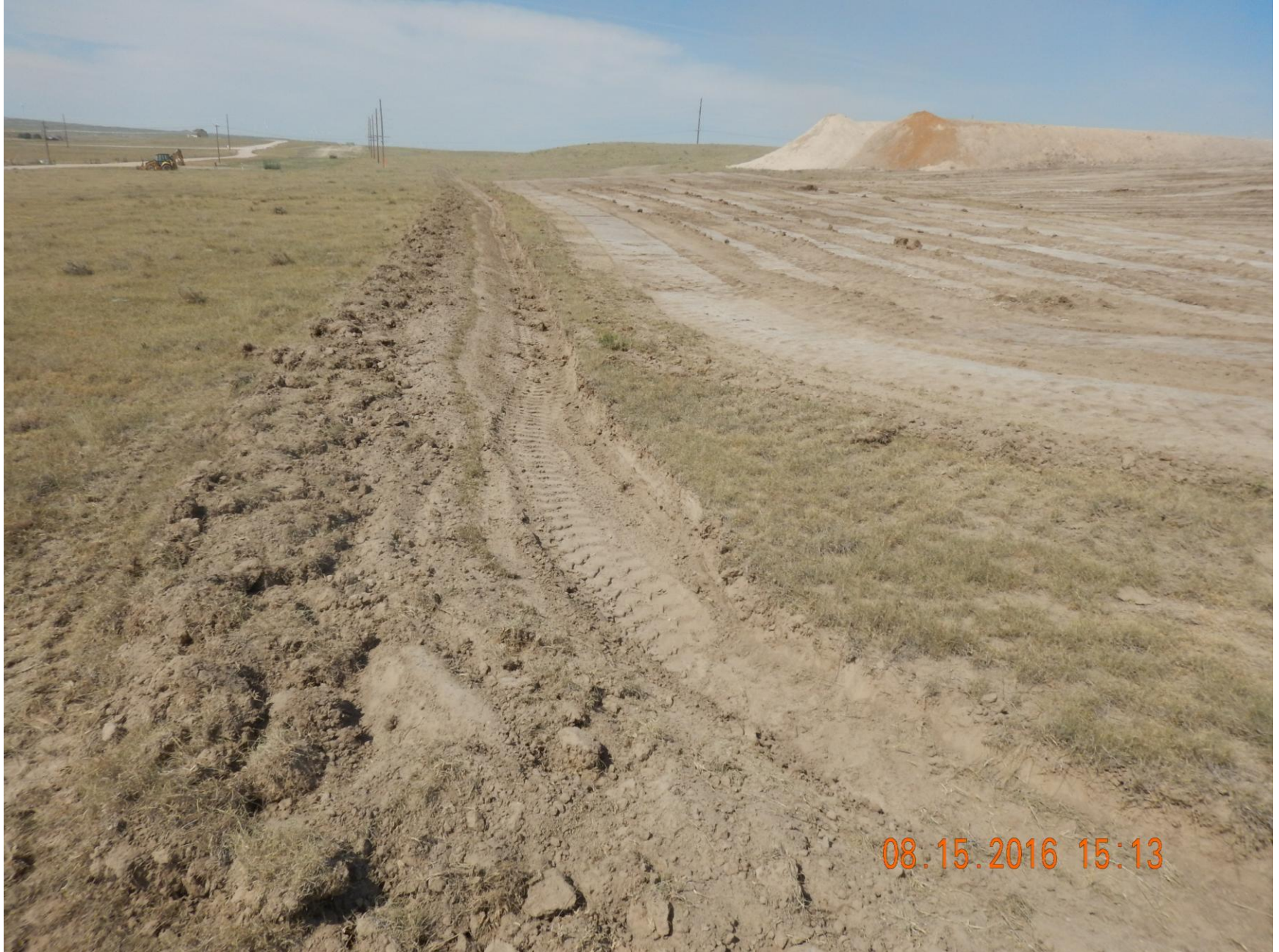
Figure 11: Photo taken from the southwest corner of the location, facing north. Photo shows stormwater and sediment control ditch BMP on the western perimeter of the location.
