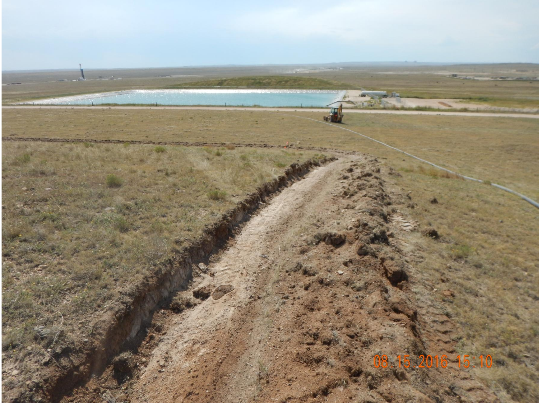
Figure 7: Photo taken from the northwest corner of the location, facing west. Photo shows stormwater and sediment control ditch BMP on the northern perimeter of the location.
