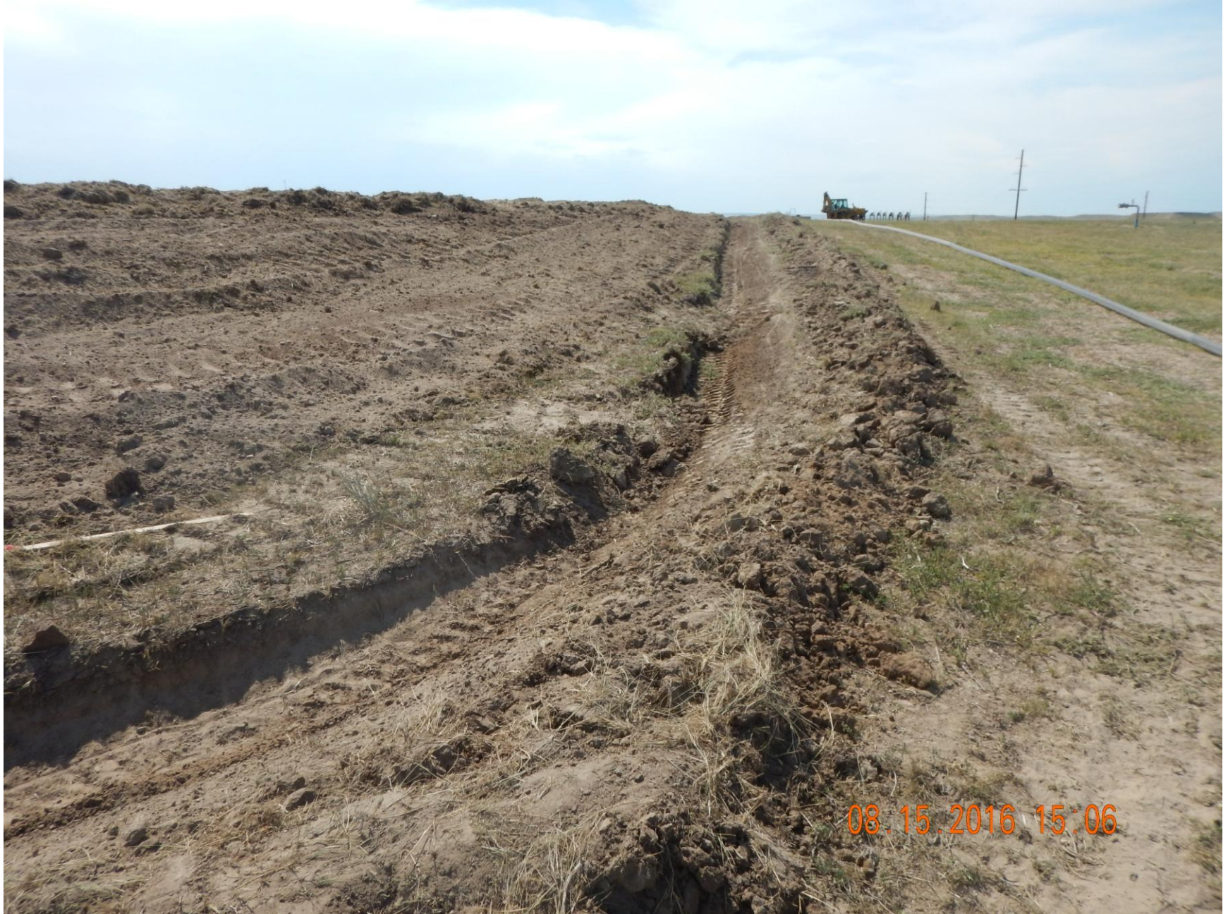
Figure 5: Photo taken from the northeast corner of the location, facing west. Photo shows stormwater and sediment control ditch BMP on the northern perimeter of the location.
