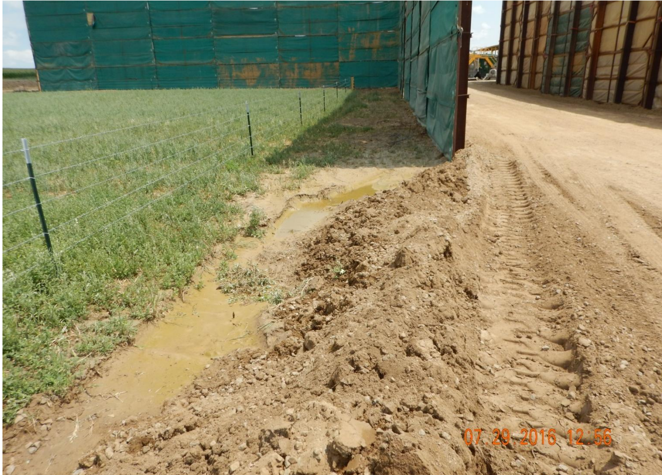
Photo 7. Photo taken from entrance of location, facing East. Flood irrigated water is running onto location from adjacent lands. Need to control run-on so that sediment is controlled and not leaving location.
