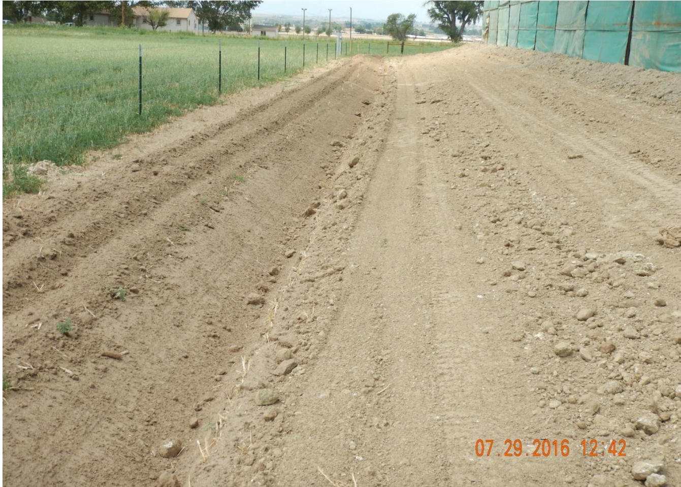
Photo 1. Photo taken from southern location, facing West. BMP installed in center of the photo.
