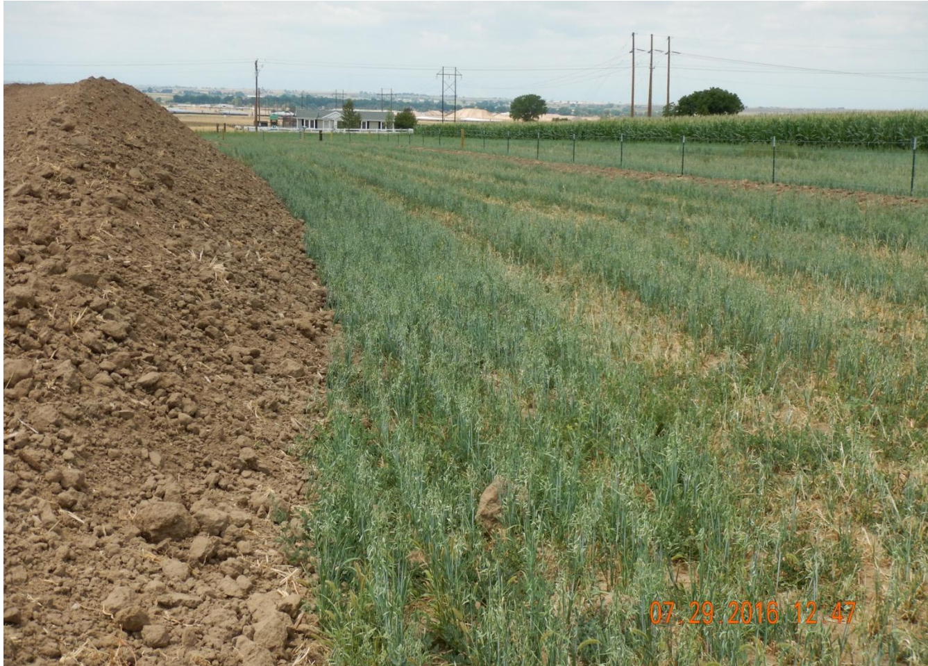
Photo 5. Photo taken from northern location, facing West, towards the north-facing topsoil stockpile. Topsoil stockpile, north-facing and south-facing, sides are steep and could pose erosion issues in the future. In the future, spread out the topsoil stockpile to eliminate the chance of erosion. There appears to be sufficient space to spread this topsoil pile out to reduce the steep side slopes.
