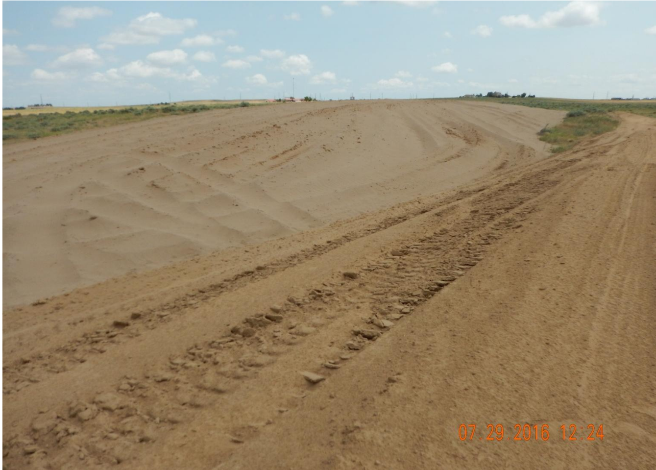
Photo 1. Photo taken from northern location, facing East, towards topsoil stockpile. BMPs should be used to stabilize this topsoil stockpile from wind erosion due to the predominately sandy soil.
