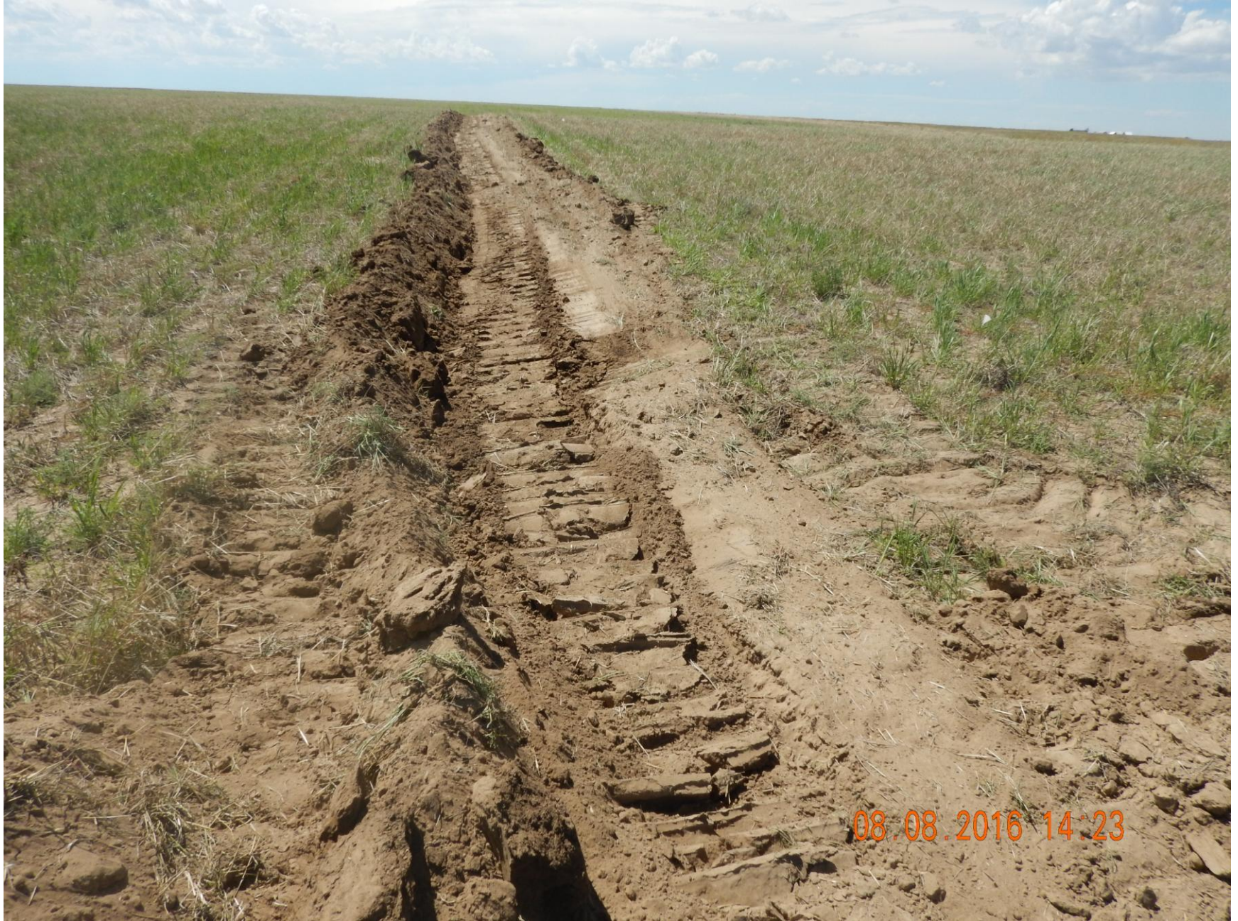
Figure 4: Photo taken from the southeast corner of the location, facing west. Photo shows stormwater and sediment control ditch on the southern perimeter.
