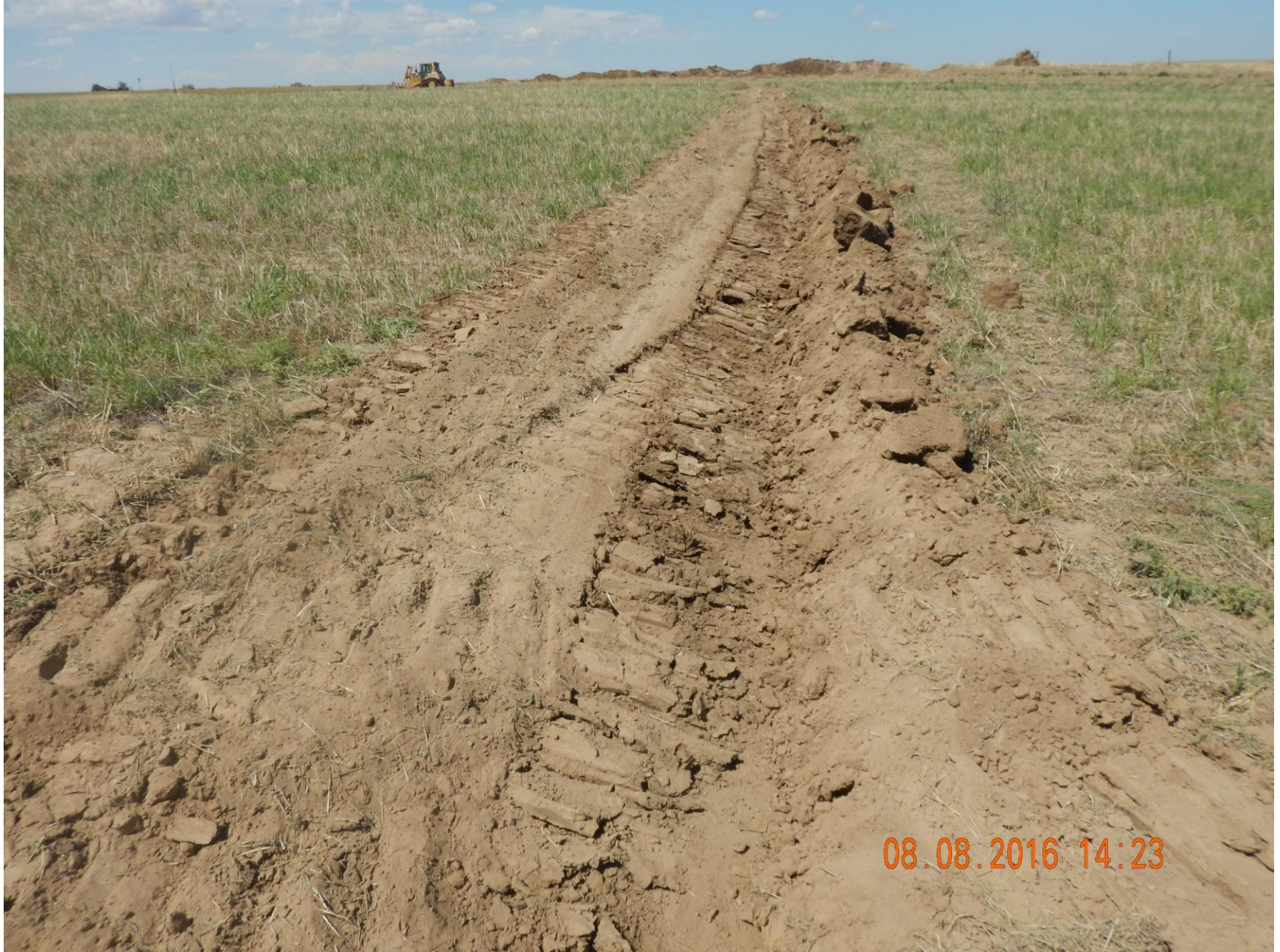
Figure 5: Photo taken from the southeast corner of the location, facing north. Photo shows stormwater and sediment control ditch on the eastern perimeter..
