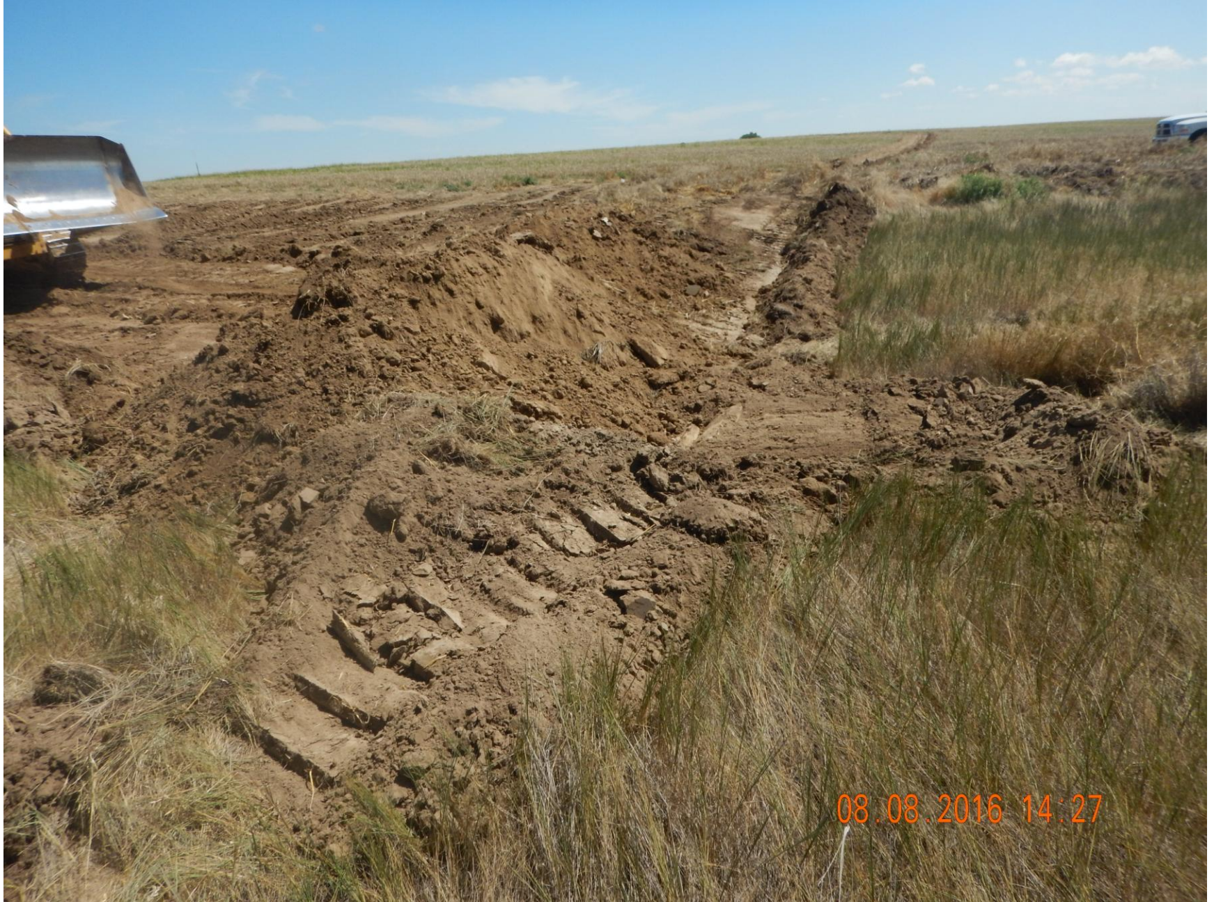
Figure 11: Photo taken from the northwest corner of the location, facing south. Photo shows stormwater and sediment control BMP incomplete on the western perimeter.
