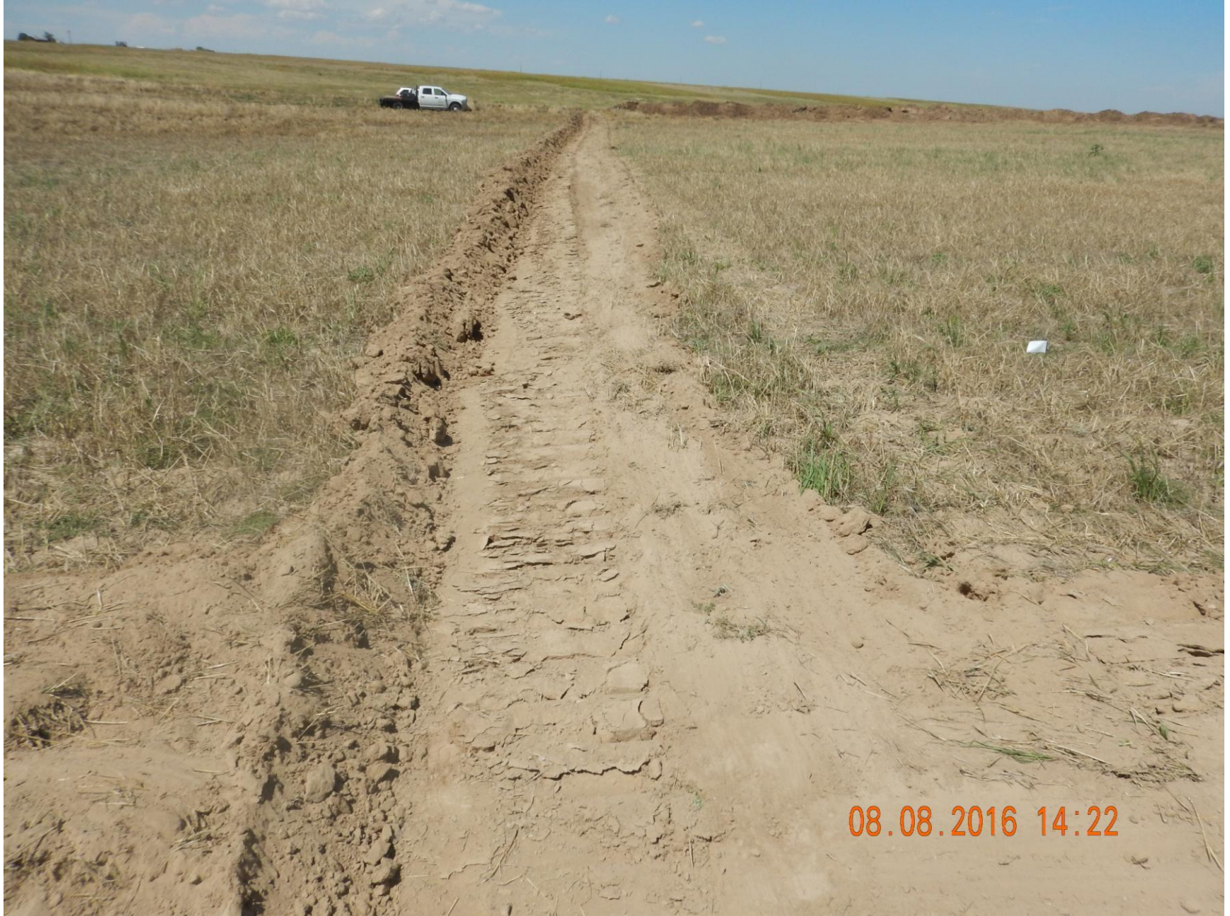
Figure 2: Photo taken from the southwest corner of the location, facing north. Photo shows stormwater and sediment control ditch on the western perimeter.
