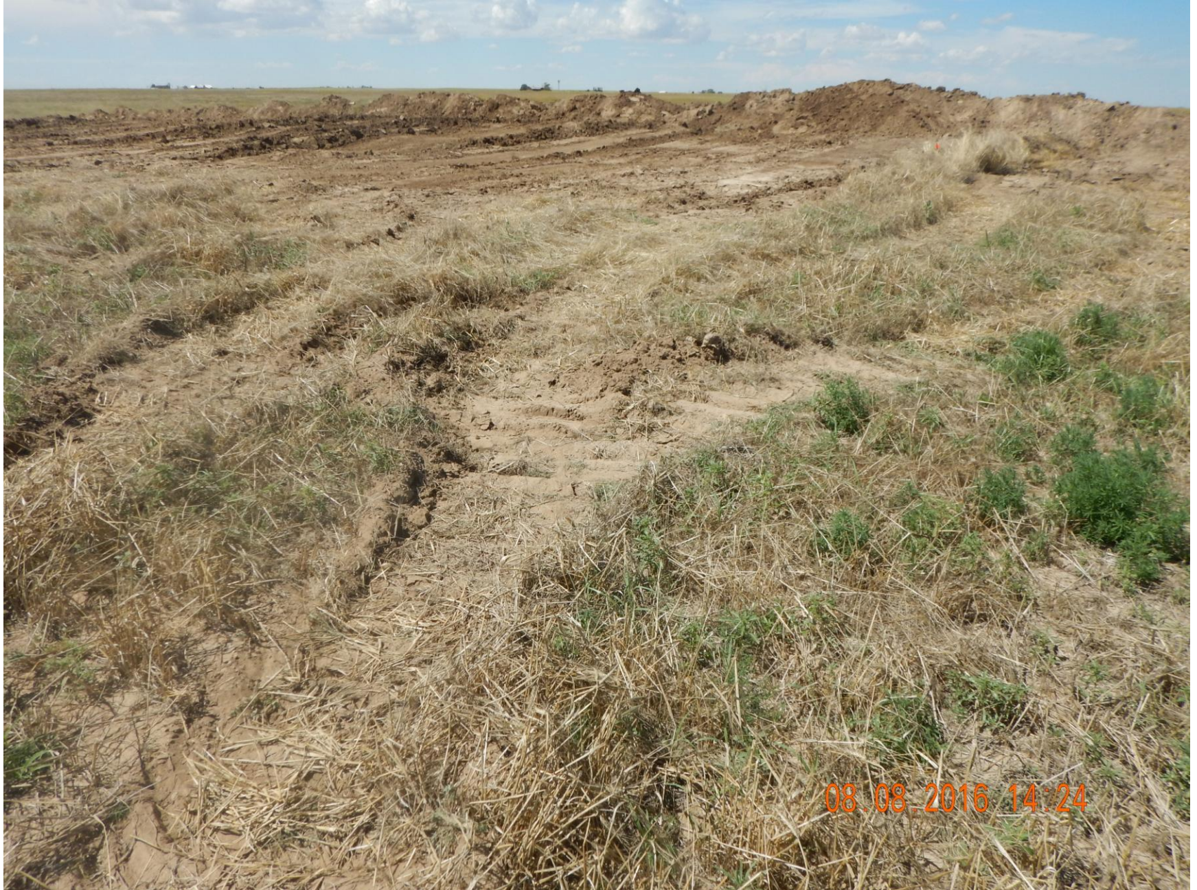
Figure 7: Photo taken from the east end of the location, facing northwest. Photo shows stormwater and sediment control BMPs absent from the northeast end of the location.
