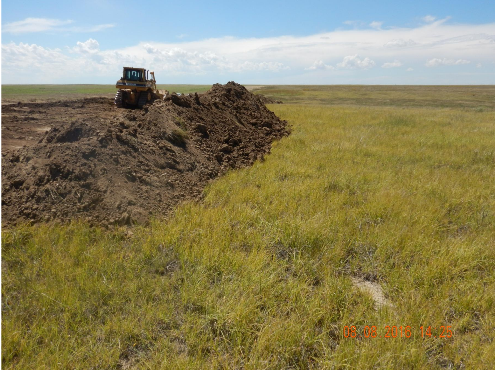
Figure 9: Photo taken from the northeast corner of the location, facing west. Photo shows stormwater and sediment control BMPs absent from north end of the location.
