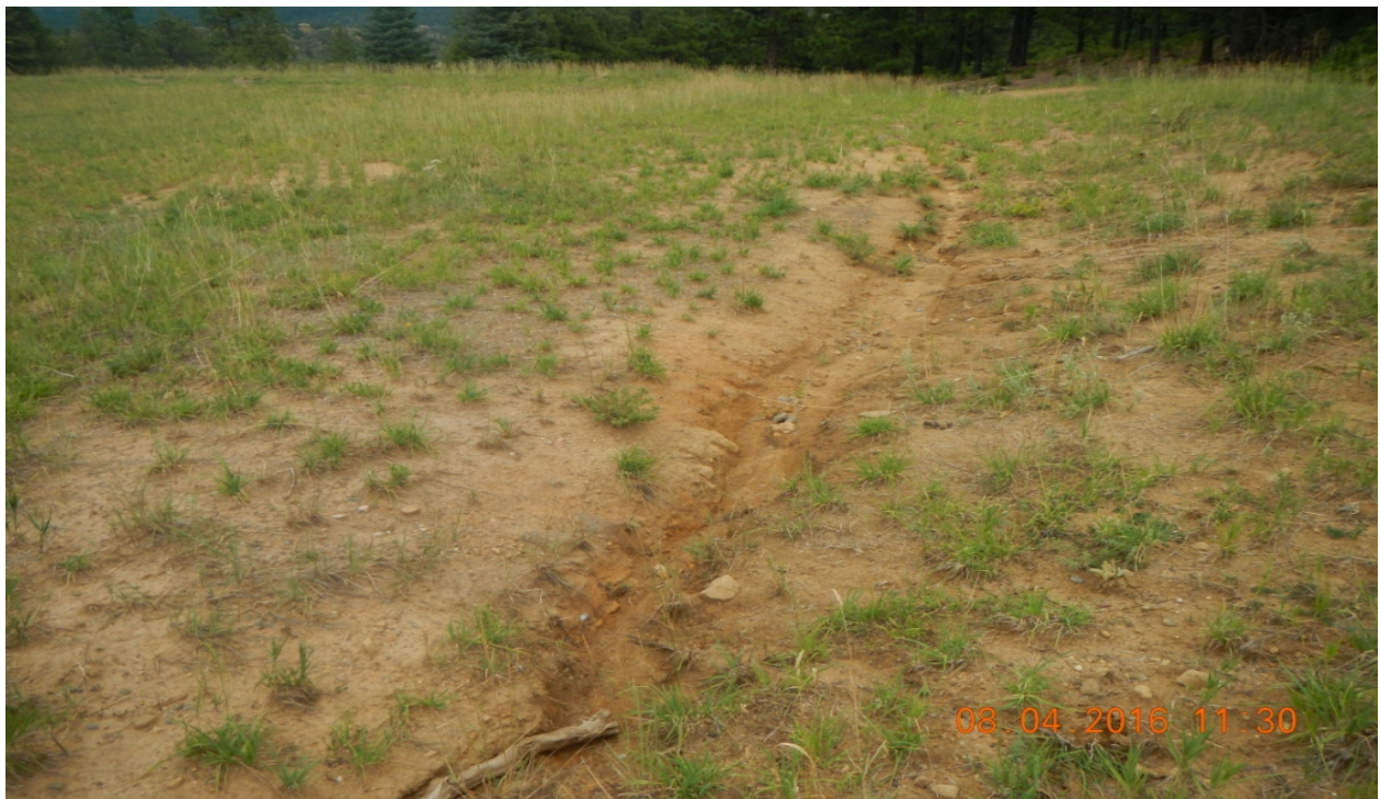
photo 6: There is an erosion channel at the southeast side of the location from stormwater directed from the access road.
