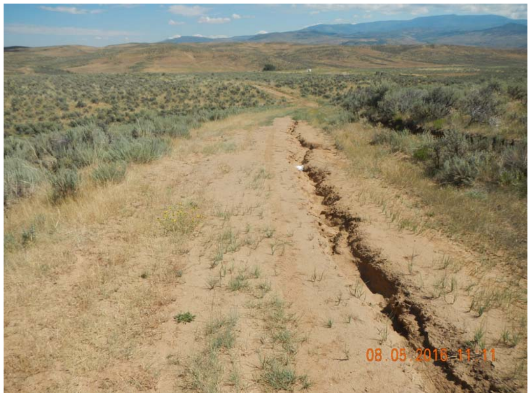
Ruts in access road. Hard hat for scale. Drainage crossing in background.
