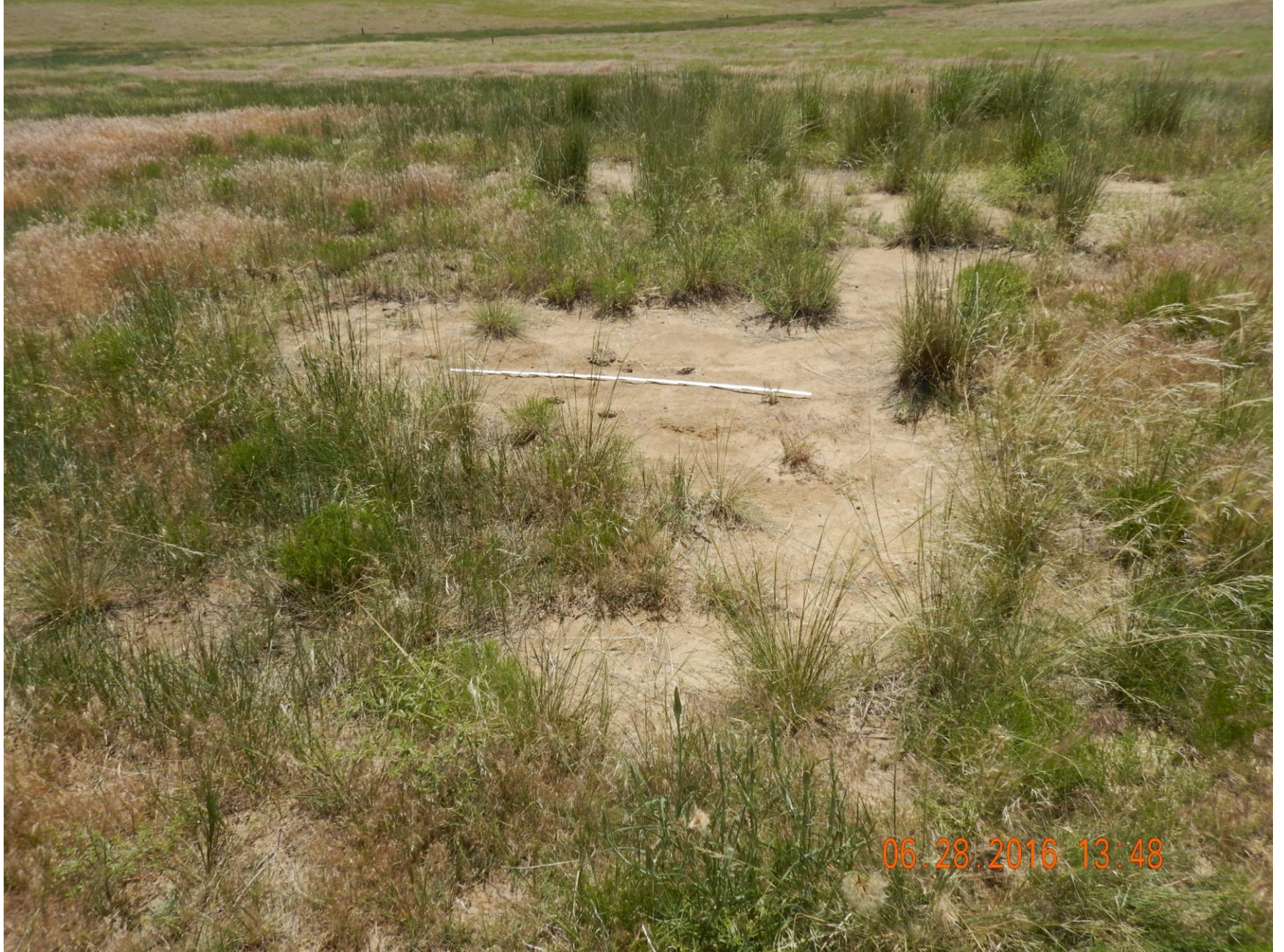
Figure 3: Photo taken from the well location, facing south. Photo shows well location has not achieved uniform vegetative cover. 6' measuring stick for reference.
