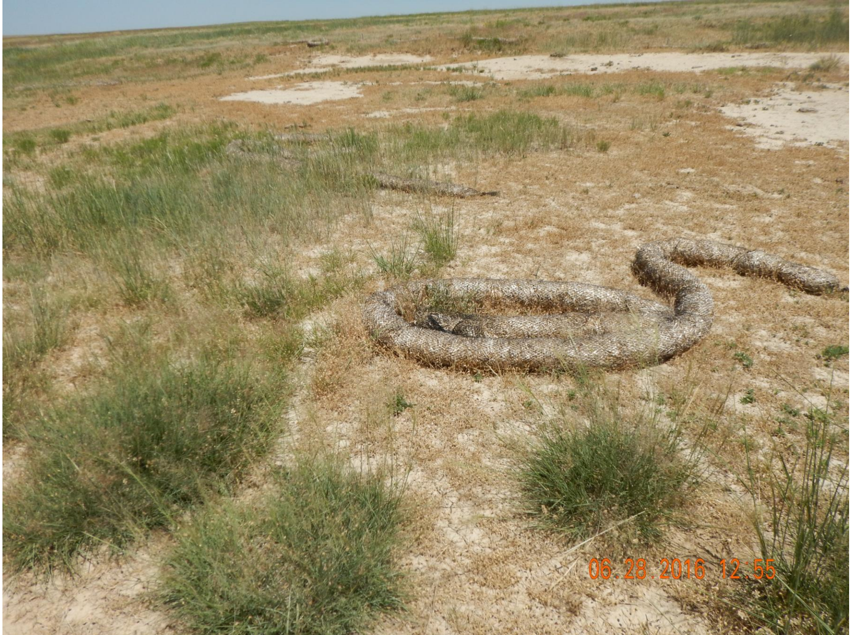
Figure 18: Photo taken from the Northern DA, facing north. Photo shows stormwater control wattles in disrepair.
