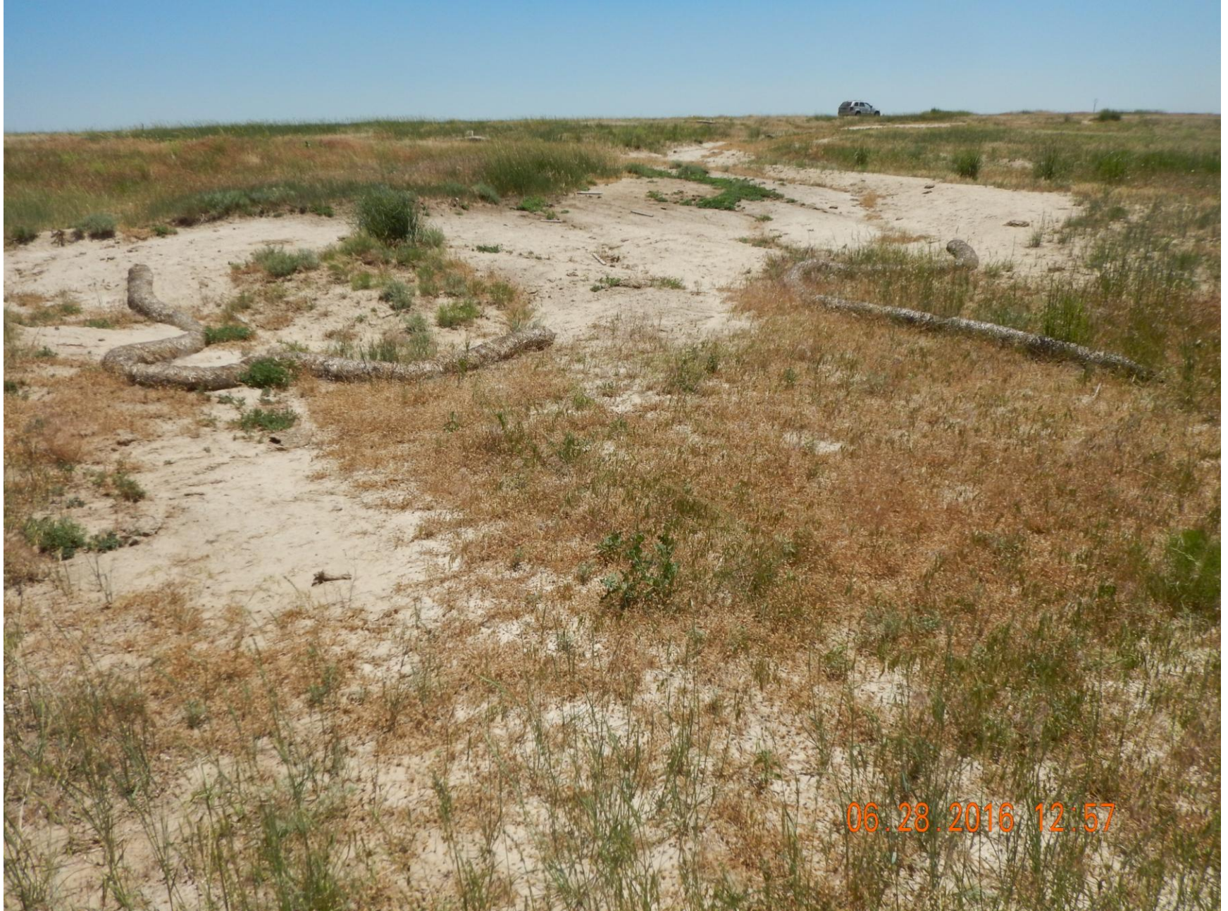
Figure 24: Photo taken from the Northern DA, facing southeast. Photo shows degradation and stormwater control wattles in disrepair.
