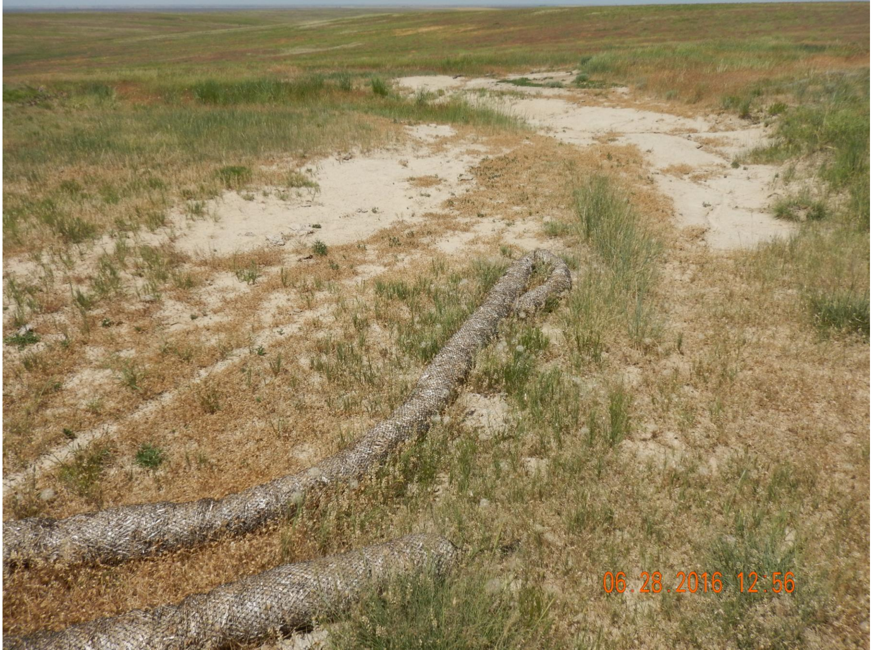
Figure 22: Photo taken from the Northern DA, facing northwest. Photo shows stormwater control wattles in disrepair.
