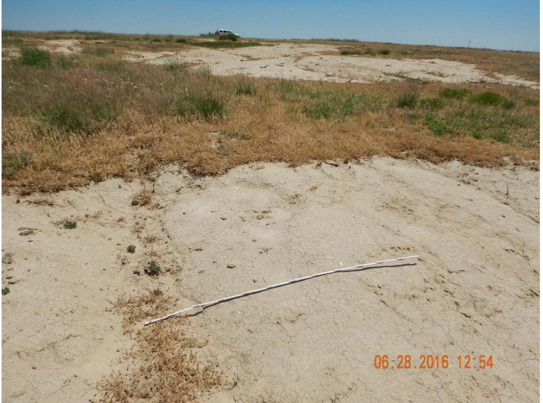
Figure 15: Photo taken from the NORTHERN DA, facing east towards the access road. Photo shows large unvegetated areas, and degradation due to erosion. 6' measuring stick for reference.
