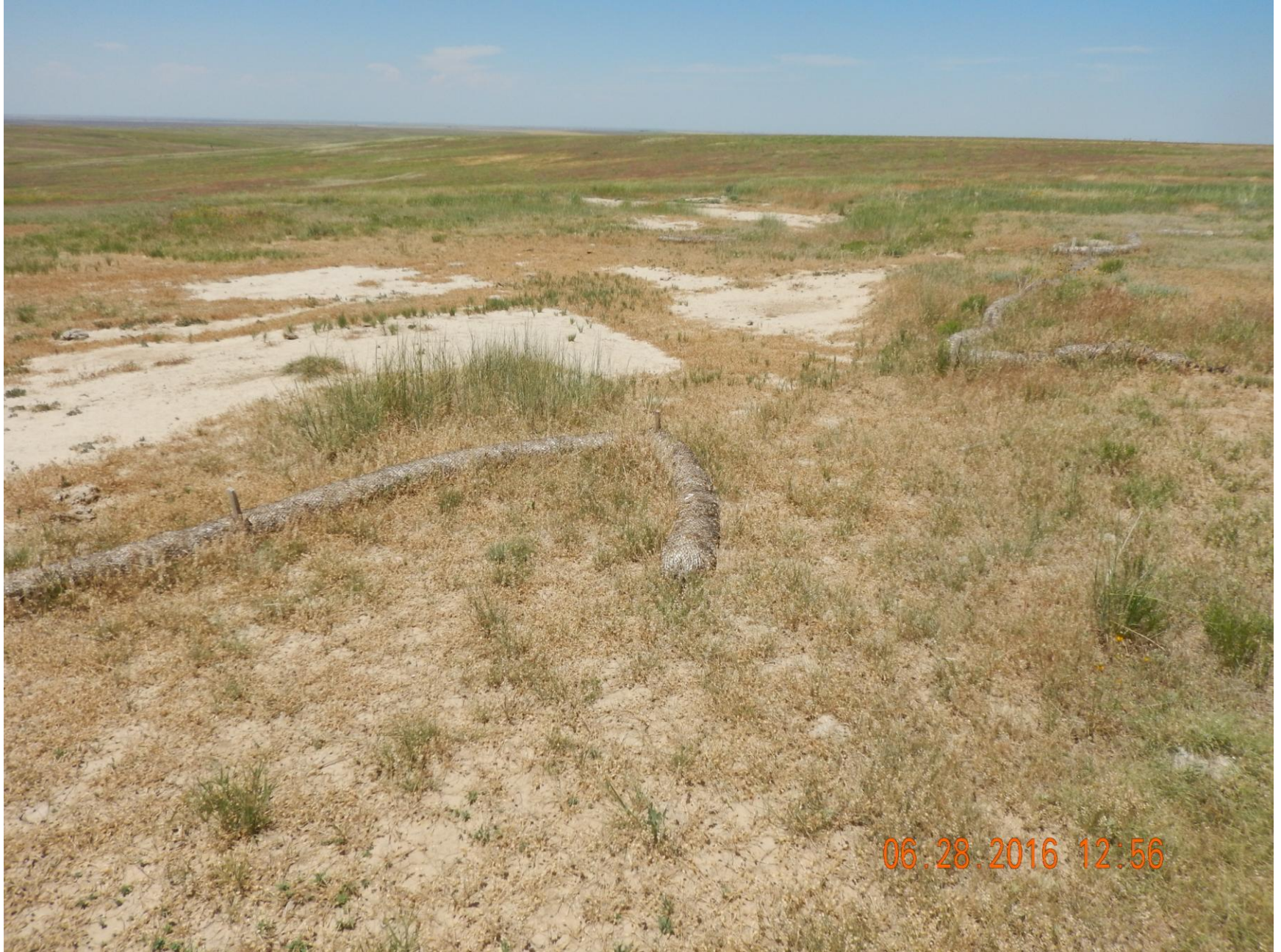
Figure 21: Photo taken from the Northern DA, facing northwest. Photo shows stormwater control wattles in disrepair.
