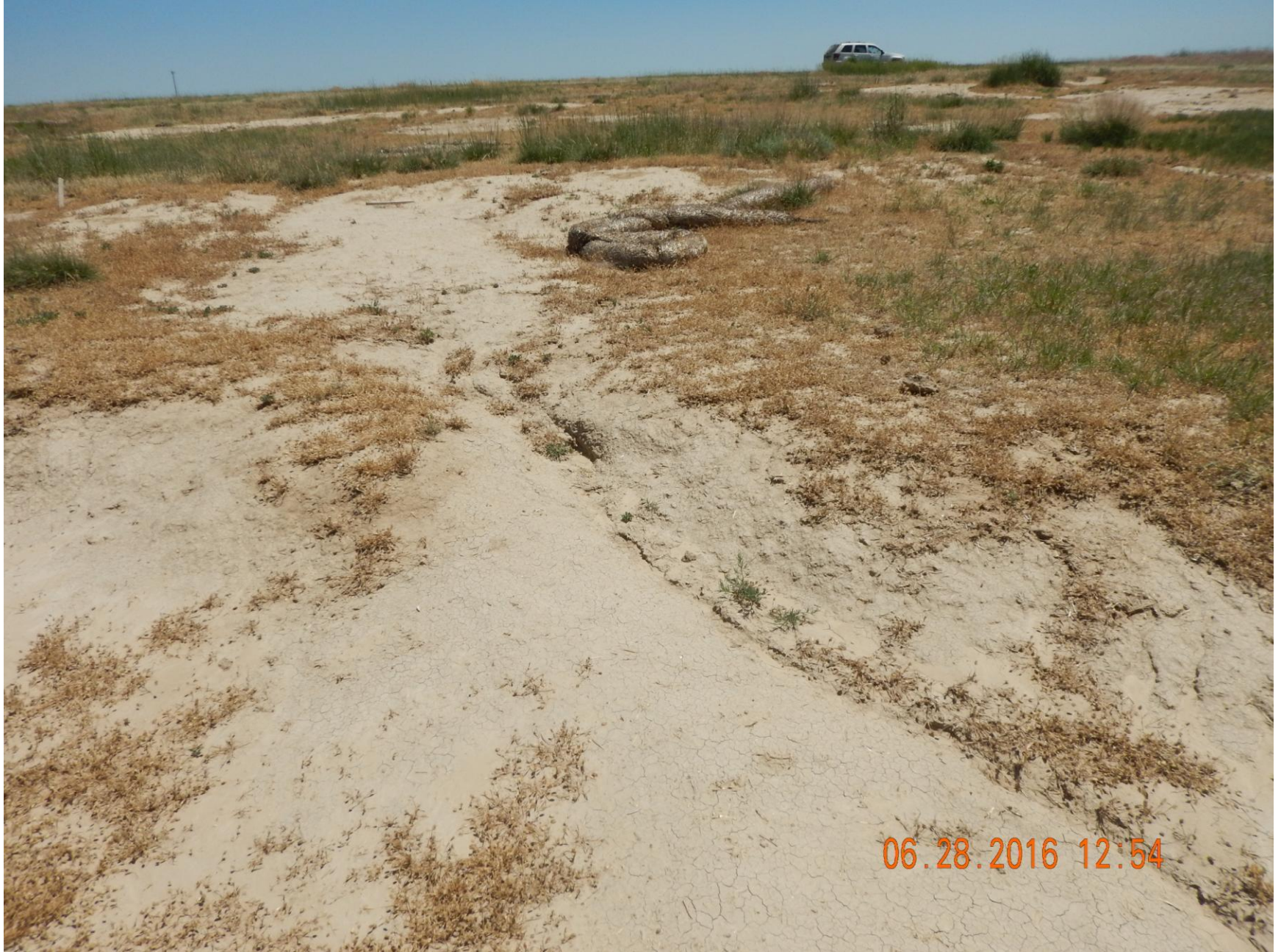
Figure 17: Photo taken from the Northern DA, facing east towards the access road. Photo shows stormwater control wattles in disrepair.
