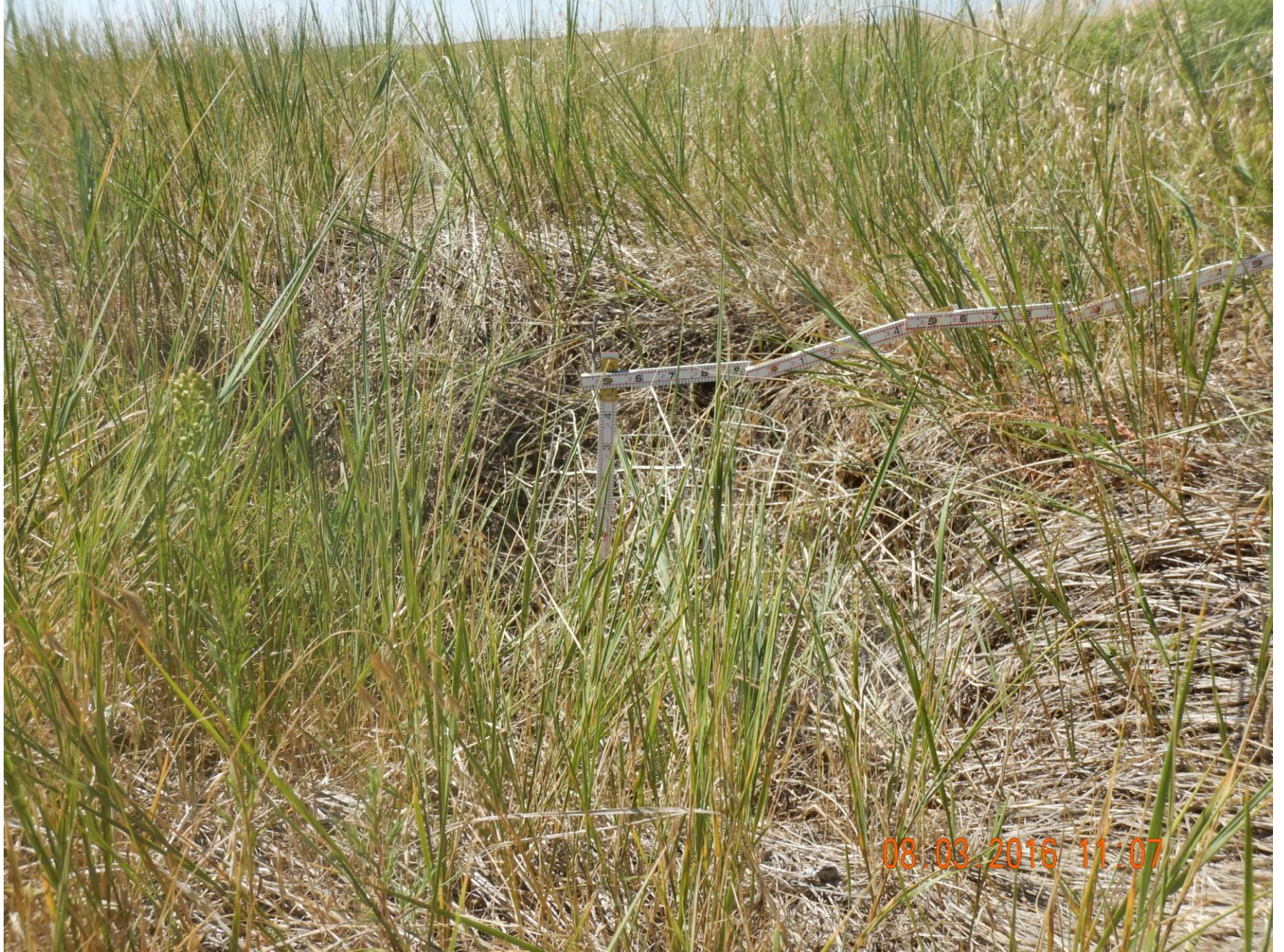
Figure 4: Photo shows large hole found on location is approximately 2 feet deep.
