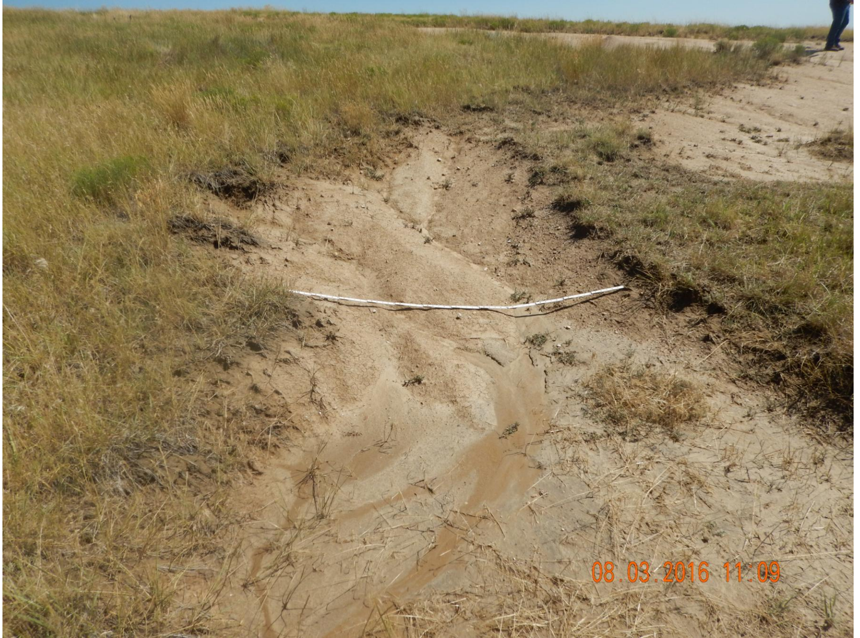
Figure 12: Photo taken from the south end of the spill area, facing north. Photo shows degradation caused by stormwater erosion over spill area.
