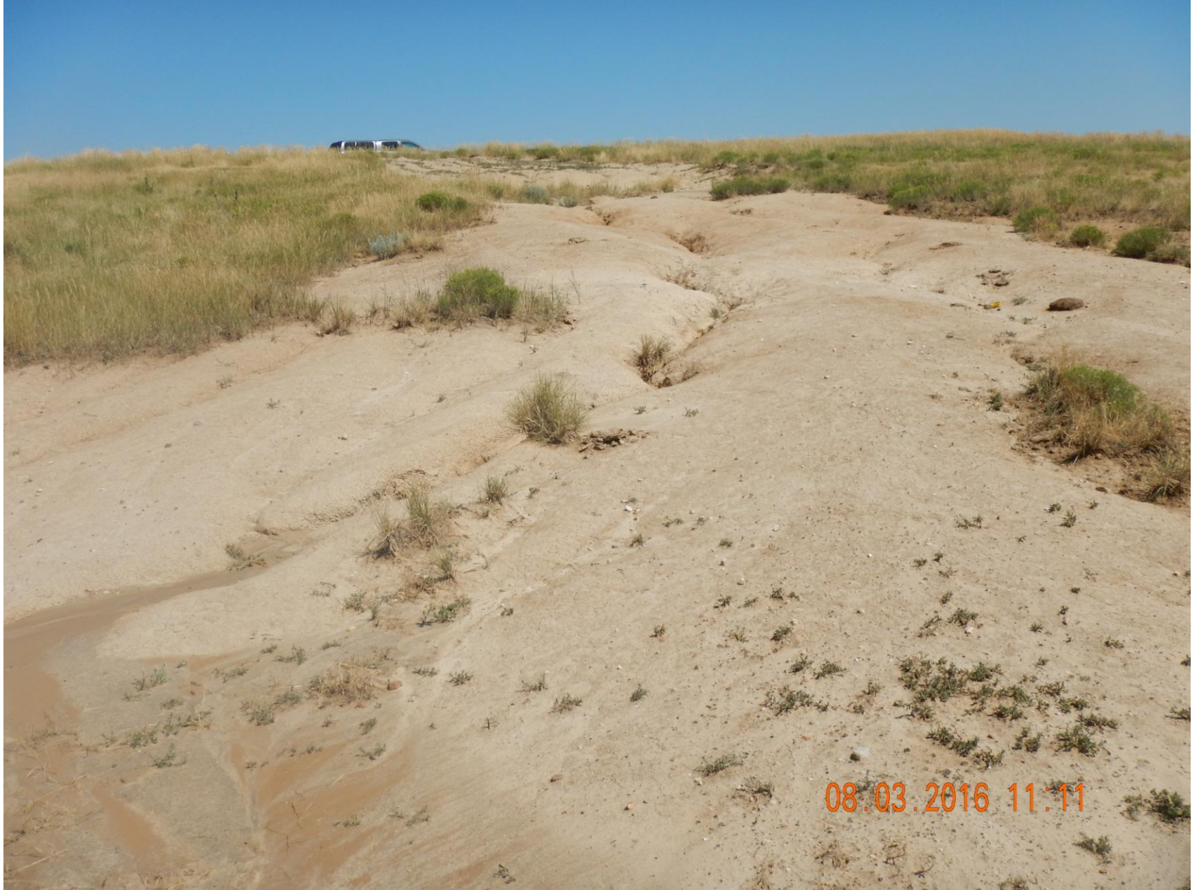
Figure 14: Photo taken from the south end of the spill area, facing north. Photo shows degradation caused by stormwater erosion over spill area.
