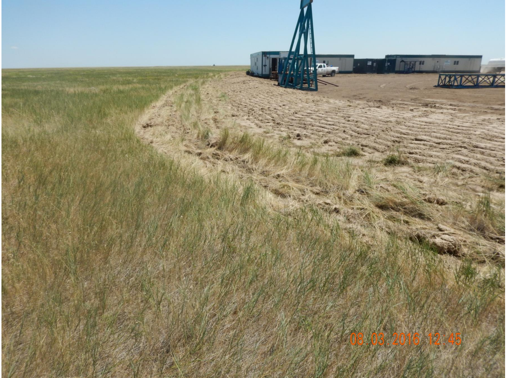
Figure 4: Photo taken from the north end of the location, facing east. Photo shows berms adequately built and tracked, and surface roughening used in conjunction.
