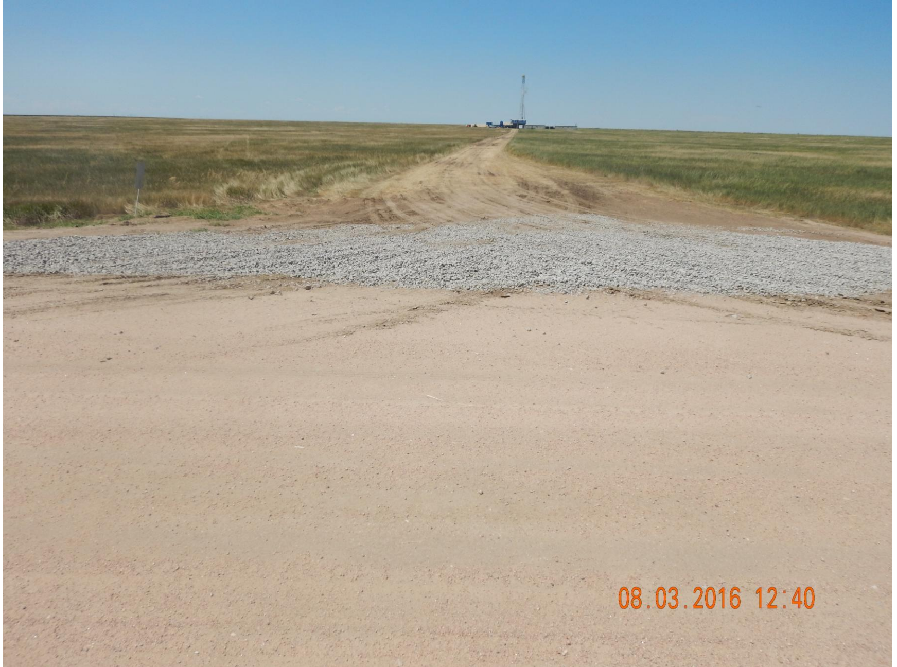
Figure 1: Photo taken from access road entrance, facing west towards location. Photo shows vehicle tracking BMP at access road.
