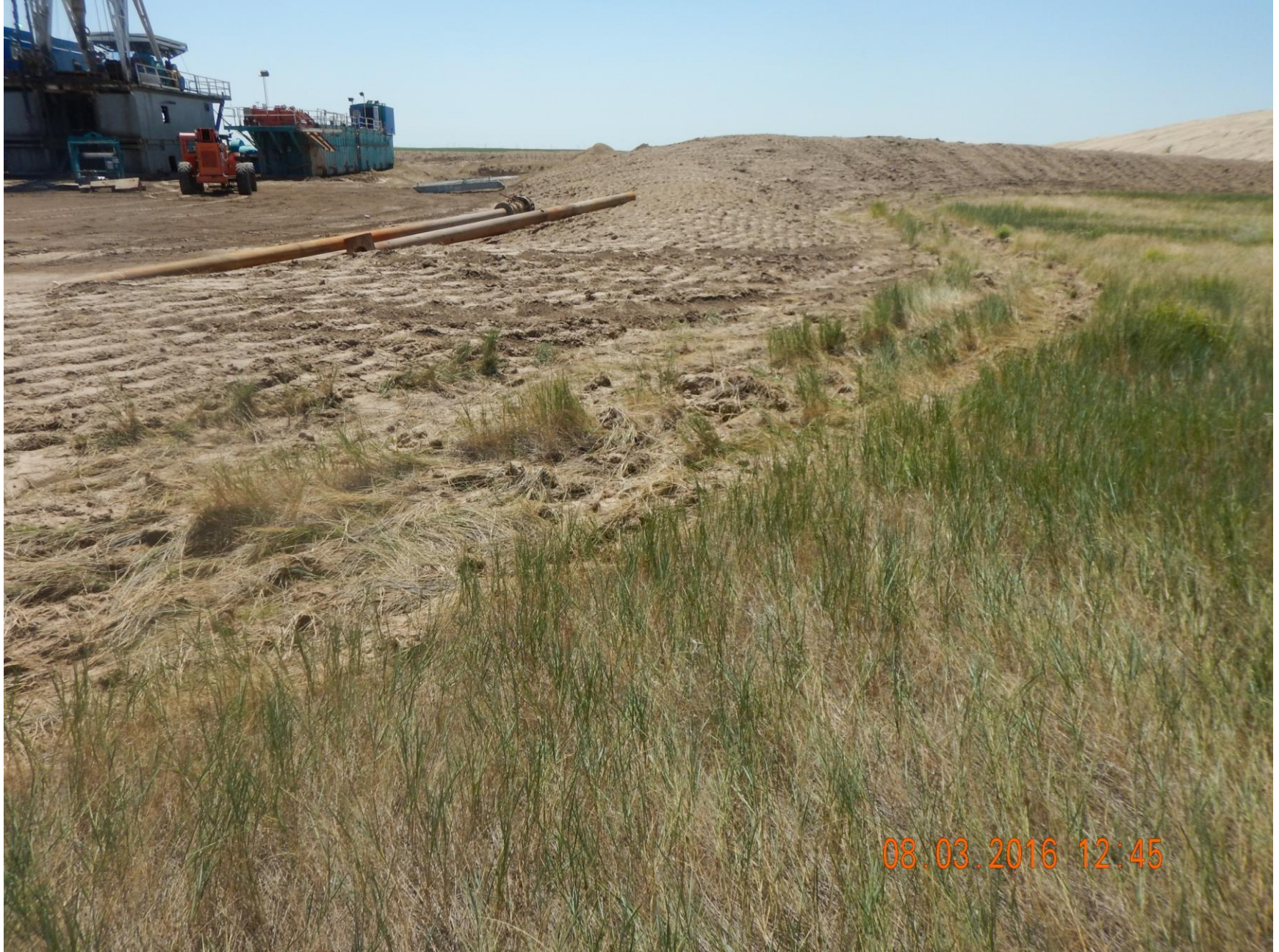
Figure 5: Photo taken from the north end of the location, facing south. Photo shows berms adequately built and tracked, and surface roughening used in conjunction.
