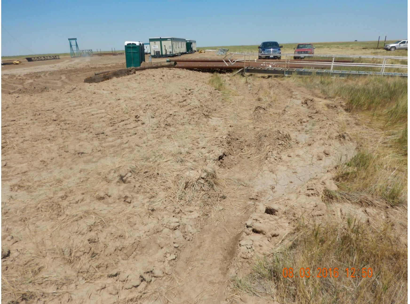
Figure 11: Photo taken from the southeast corner of the location, facing north. surface roughening appears to have been traveled over. Vehicle traffic may re-compact the surface roughening, and prevent the BMP from properly functioning
