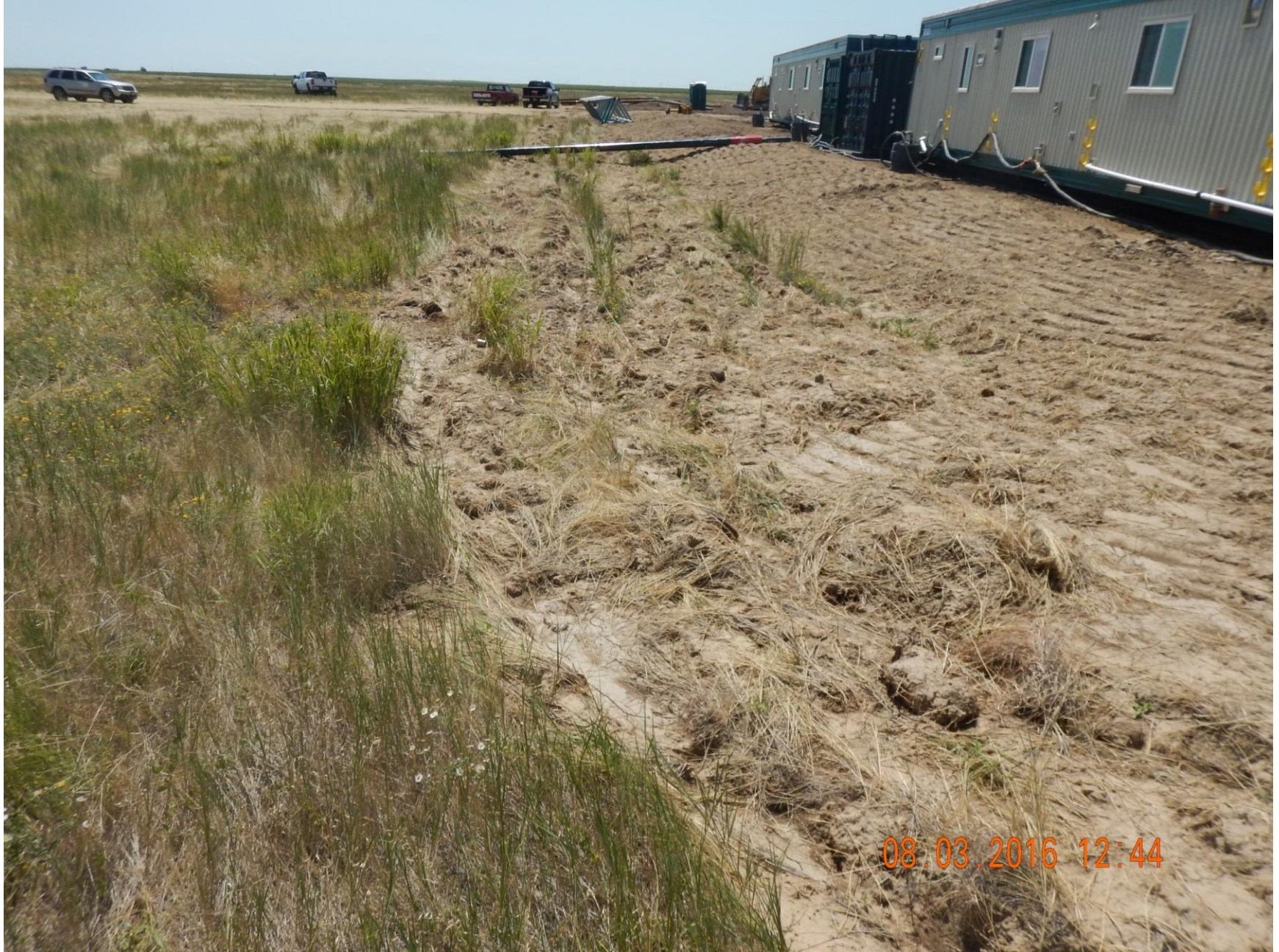
Figure 2: Photo taken from the northeast corner of the location, facing south. Photo shows berms adequately built and tracked, and surface roughening used in conjunction.
