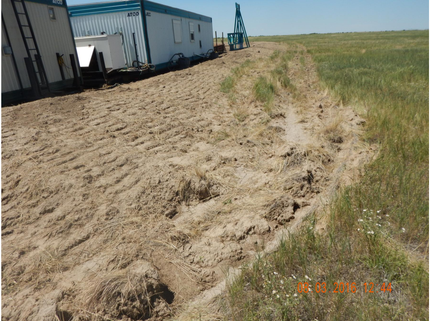
Figure 3: Photo taken from the northeast corner of the location, facing west. Photo shows berms adequately built and tracked, and surface roughening used in conjunction.
