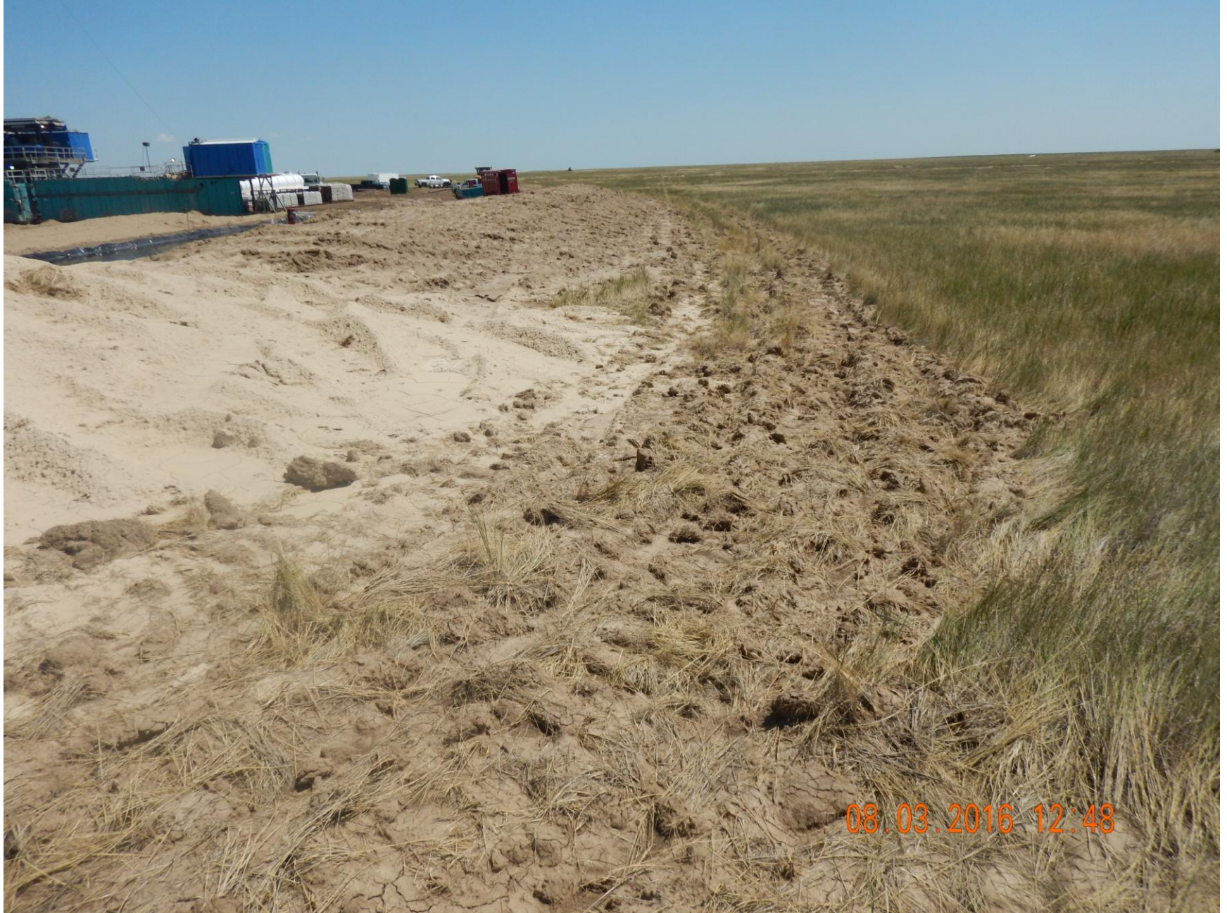
Figure 10: Photo taken from the southwest corner of the location, facing east. Photo shows berms adequately built and tracked, and surface roughening used in conjunction.
