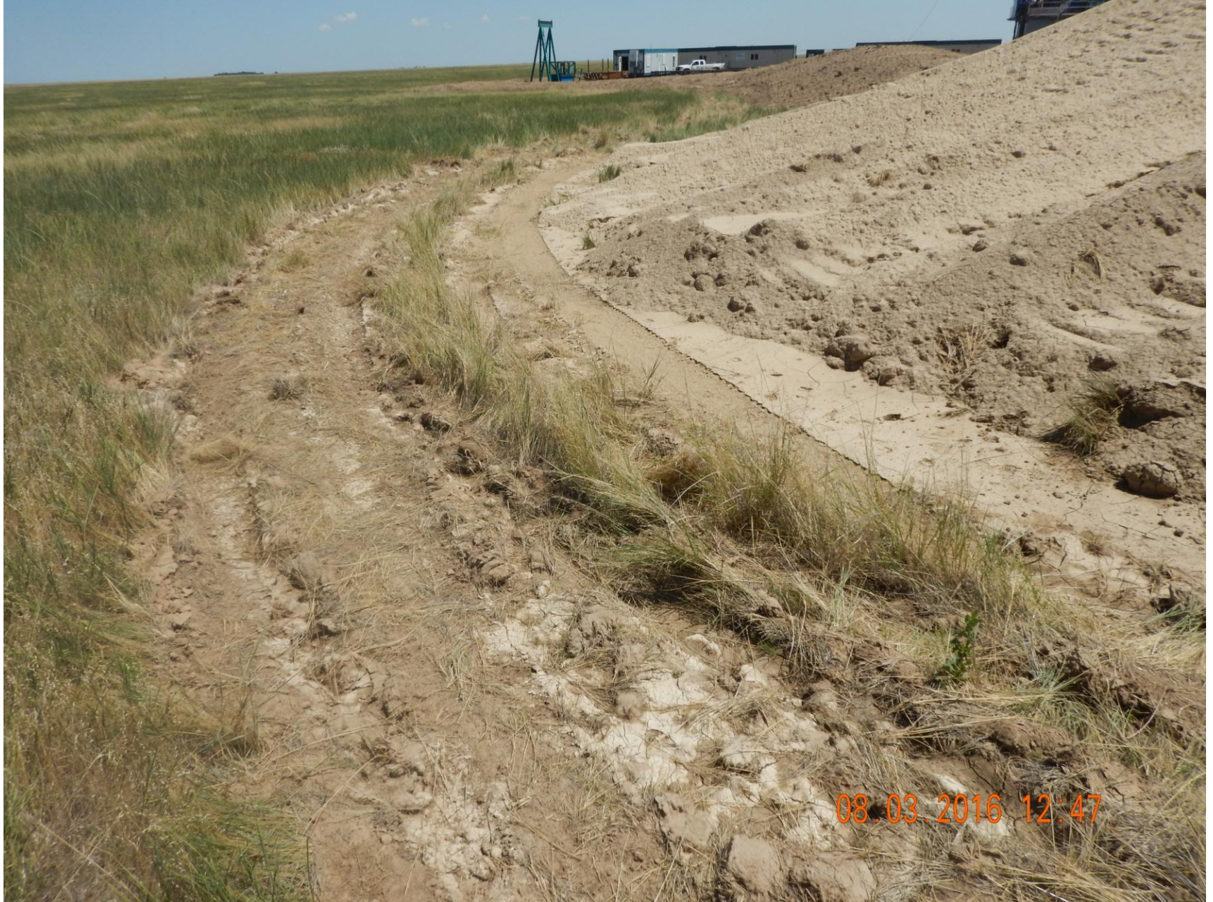
Figure 7: Photo taken from the northwest corner of the location, facing east. Photo shows surface roughening appears to have been traveled over. Vehicle traffic may re-compact the surface roughening, and prevent the BMP from properly functioning
