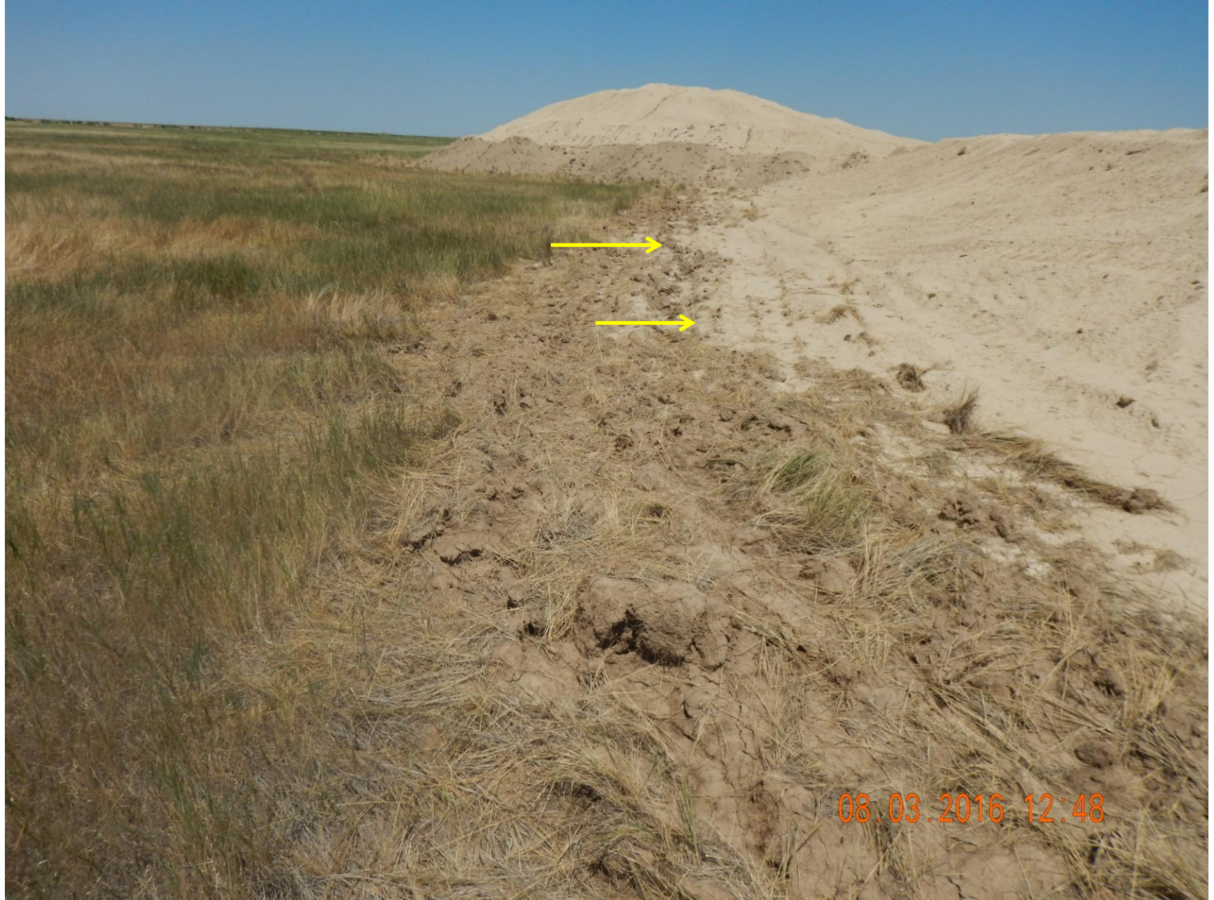
Figure 9: Photo taken from the northwest corner of the location, facing east. Photo shows surface roughening. Note sediment build up to right that was caught by BMP. These areas will need to be monitored, if sediment continues to fill BMP, maintenance will be required.
