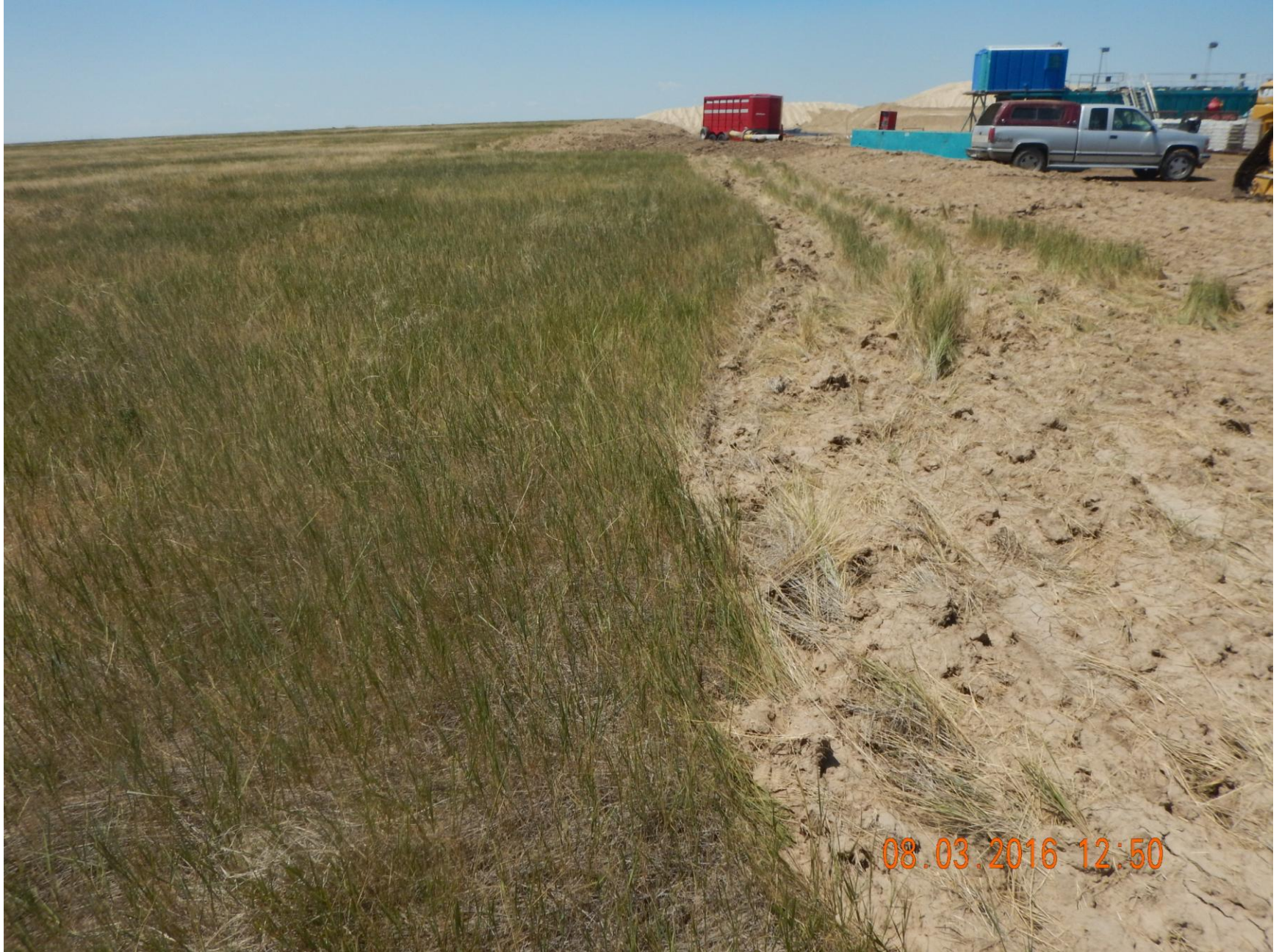
Figure 12: Photo taken from the southeast corner of the location, facing west. Photo shows berms adequately built and tracked, and surface roughening used in conjunction.
