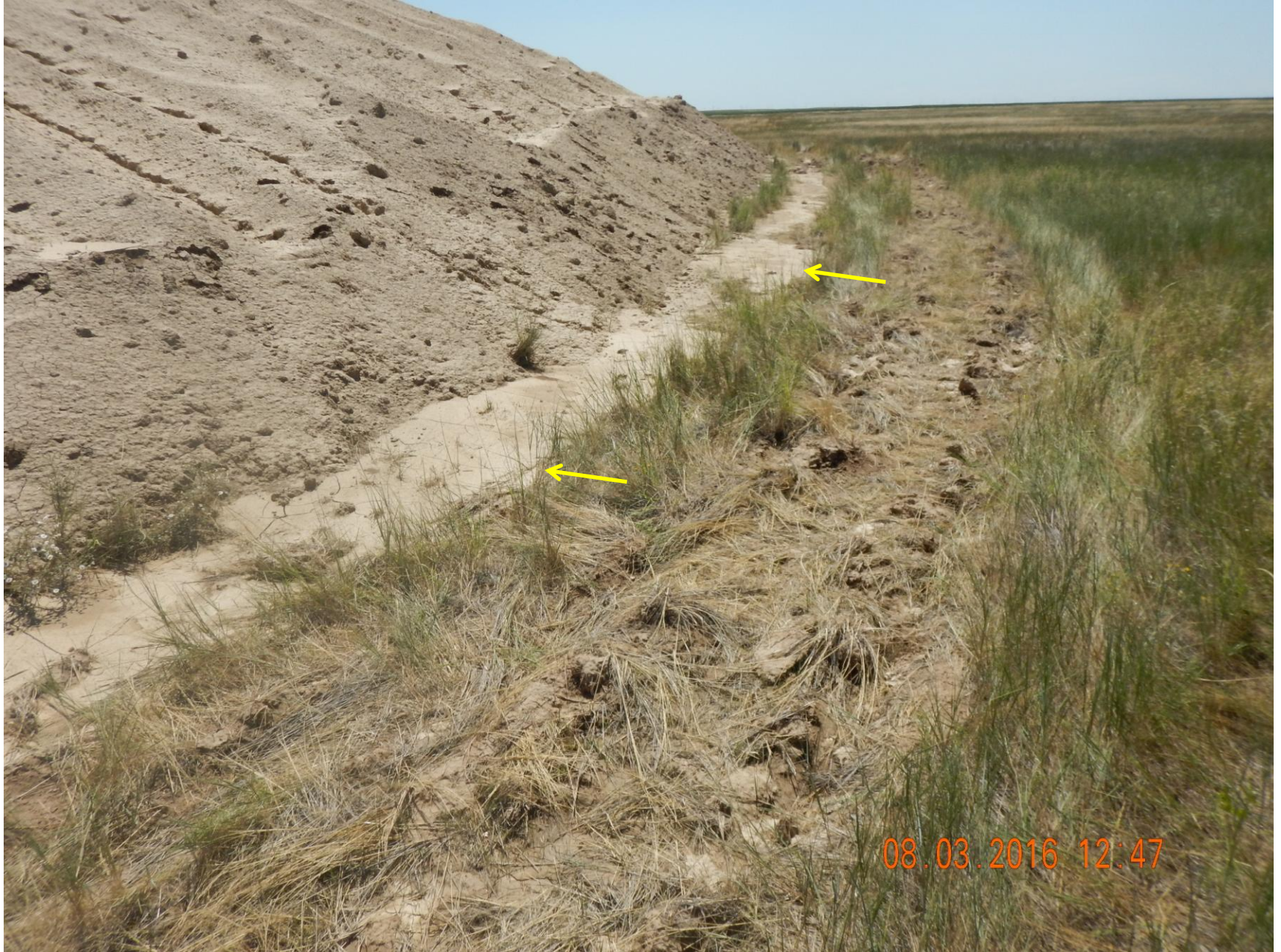
Figure 8: Photo taken from the northwest corner of the location, facing east. Photo shows surface roughening. Note sediment build up to left that was caught by BMP. These areas will need to be monitored, if sediment continues to fill BMP, maintenance will be required.
