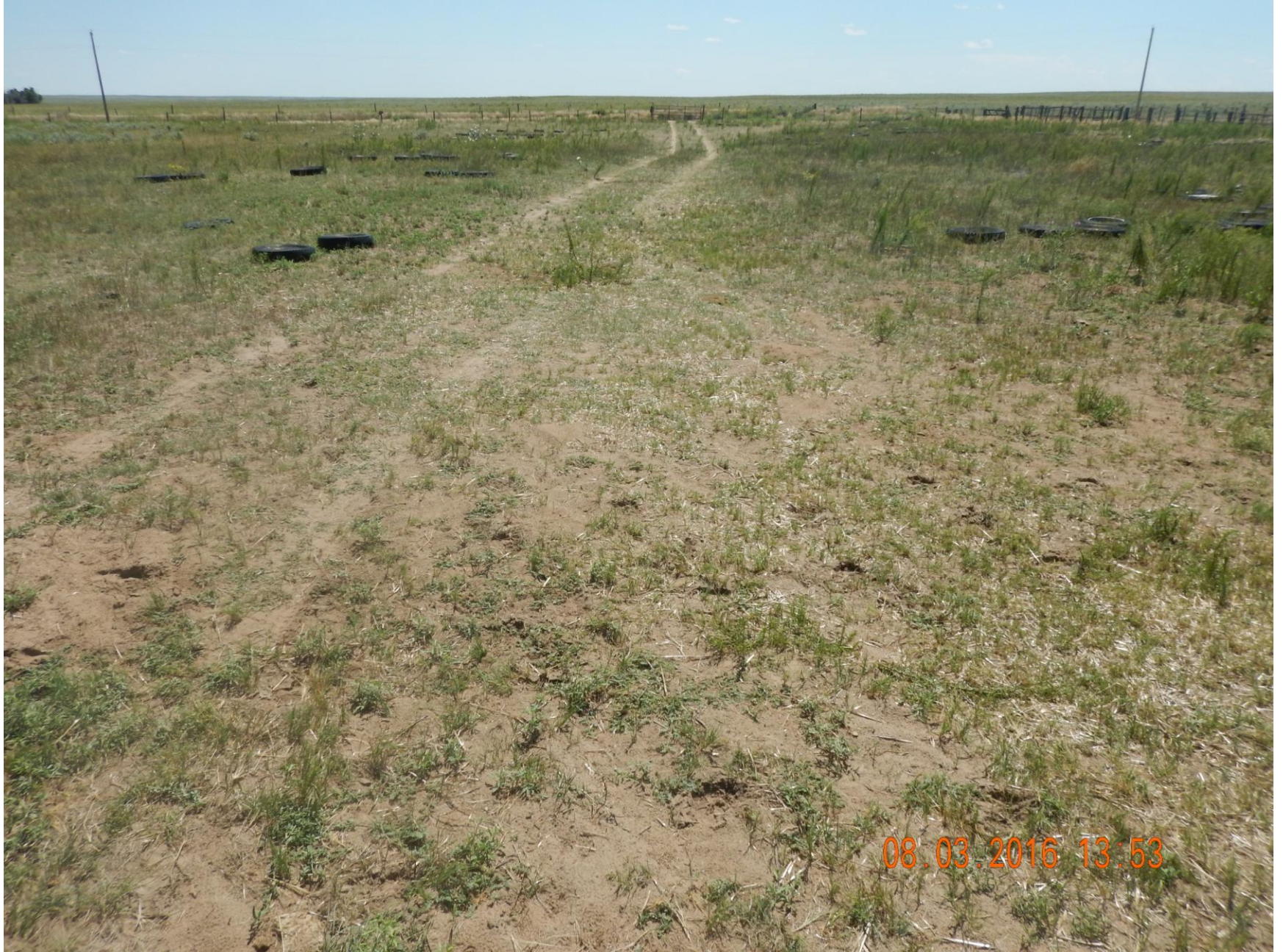
Figure 2: Photo taken from ranch two-track just north of the access gate on County Road F, facing south. Straw crimped into soil appears to be holding.
