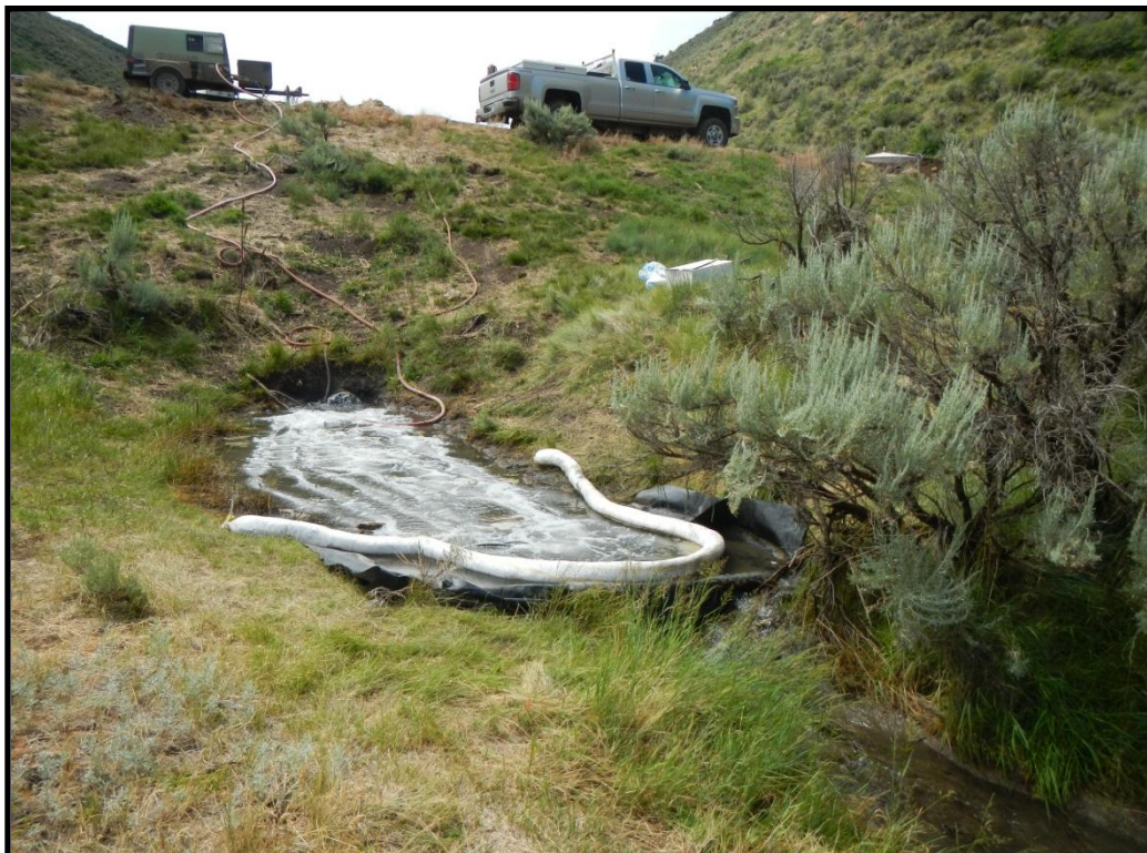
Aeration system installed to remove VOCs.
