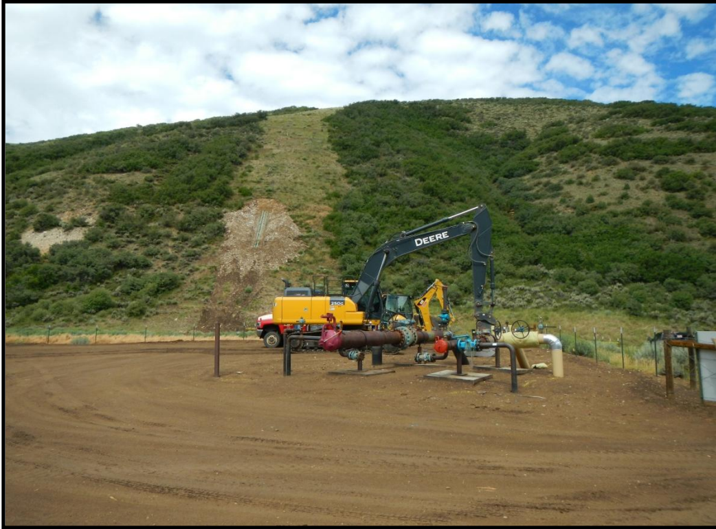
From A27 CDP looking west. Pipeline leak identified at the bottom of exposed pipeline
