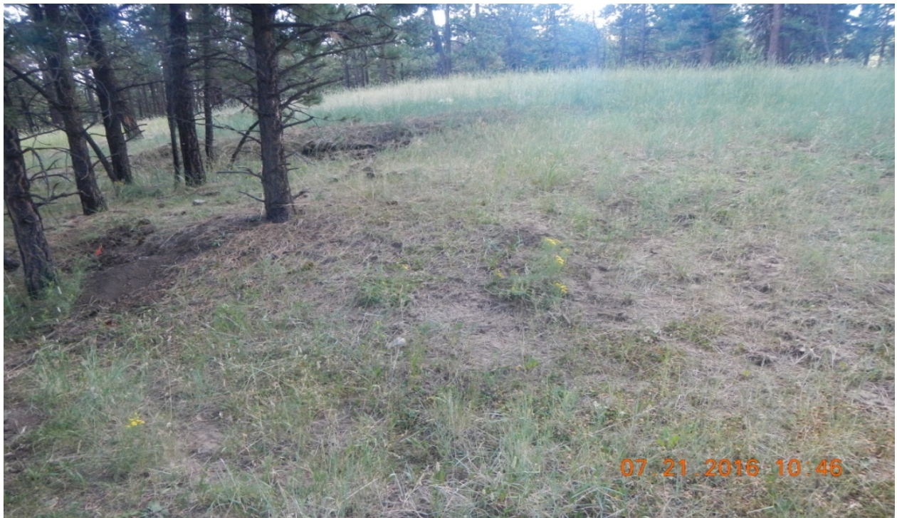
photo 10: North side of the location facing southeast along the fill slope.
