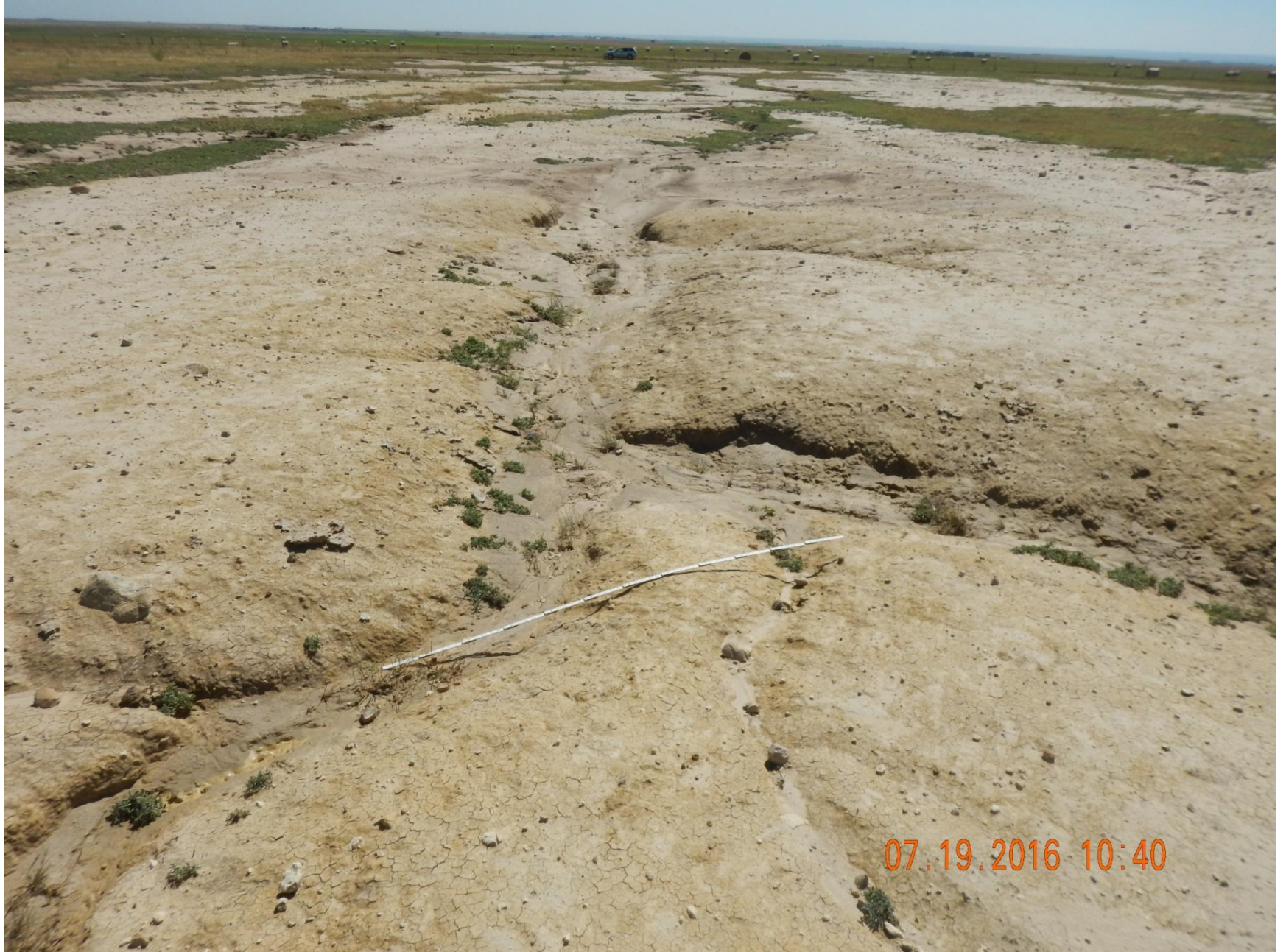
Figure 13: Photo taken from the west end of the location, facing east. Photo shows areas of degradation due to stormwater erosion and possible salt kill from the location. 6' measuring stick for reference
