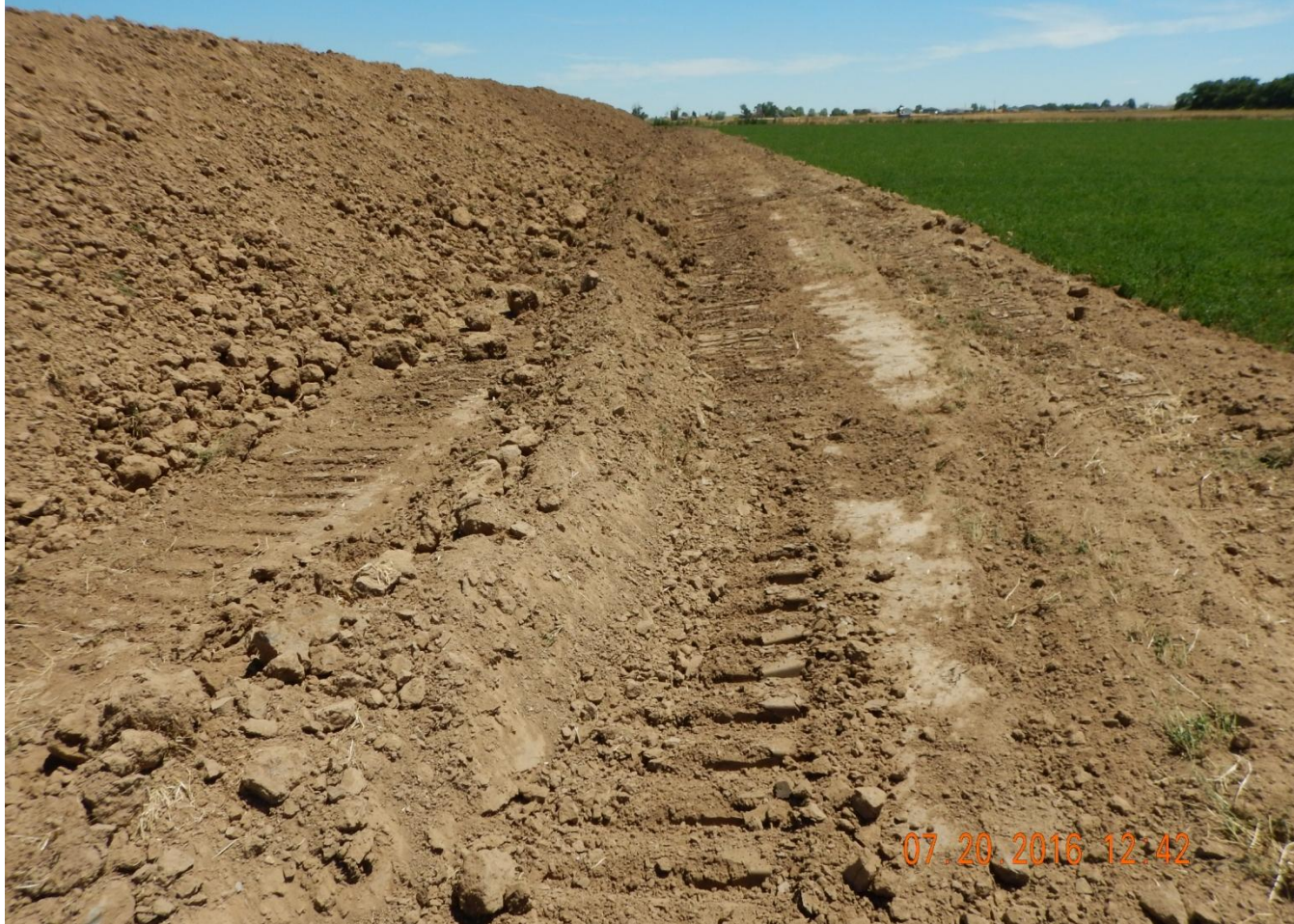
Photo 2. Photo taken from southwest location, facing East. Need to stabilize topsoil stockpile upon completion of salvage operations. Unconsolidated berms along perimeter of location need to be compacted.
