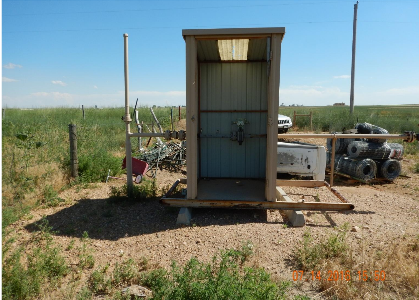
Photo 2. Photo taken of equipment which needs to be removed and reclaimed per Rule 1004.
