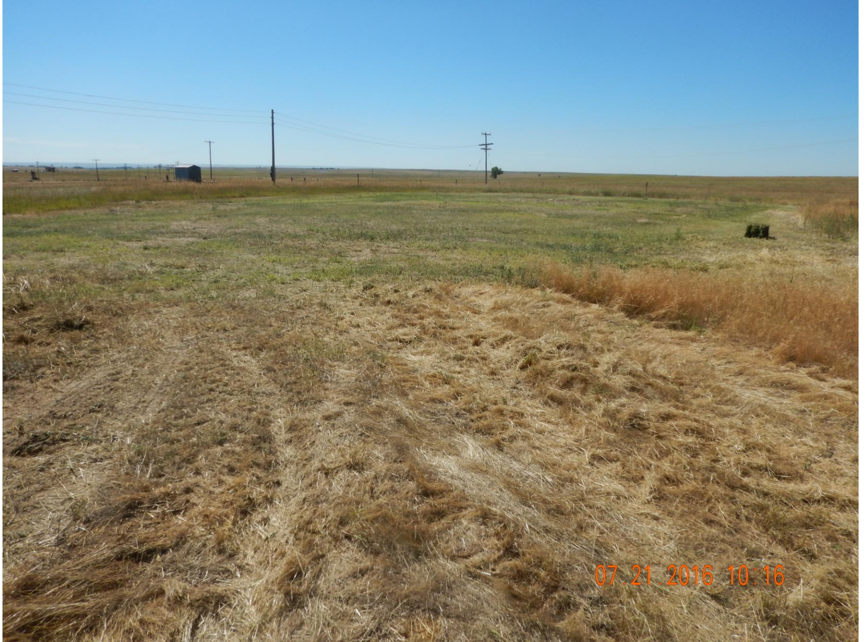
Figure 3: Photo taken from the location, facing south. Photo shows areas around battery have been mowed/weed-wacked and debris has been baled.
