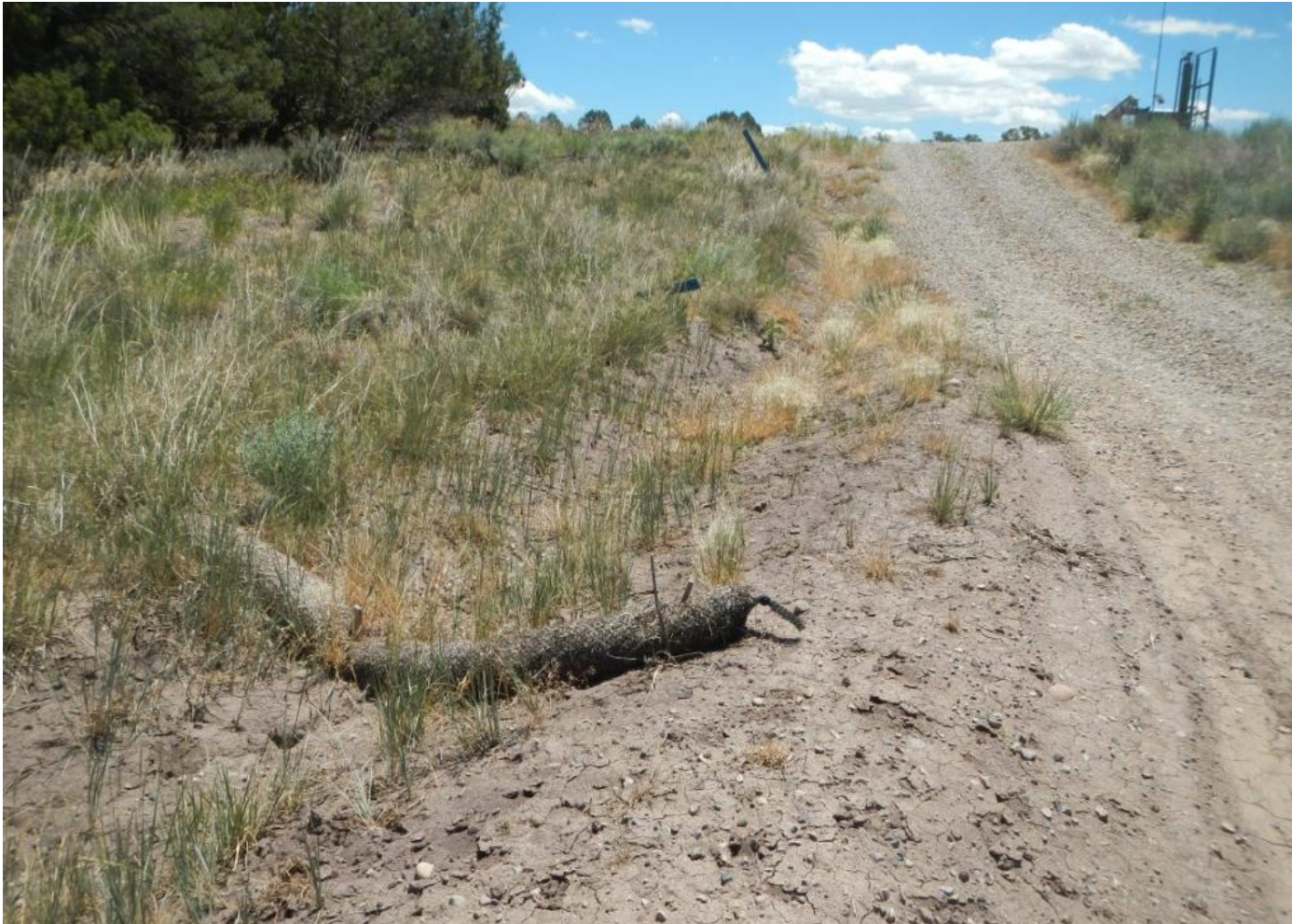
Photo 1. View of the access road to the well pad facing upslope from the well pad entrance. Revegetation appears to be helping to stabilize slope. Wattles here are in acceptable condition.
