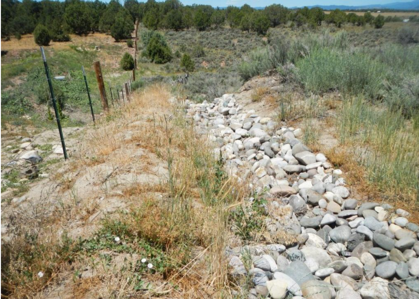
Photo 4. View of cobble run-down in the western portion of the project area appears to be functioning.
