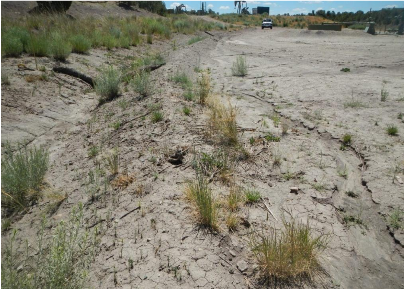
Photo 6. View of eastern edge of the well pad working area from the northeastern corner facing southward. Stormwater flows on the well pad surface is resulting in channeling on the well pad (right hand side of photo).
