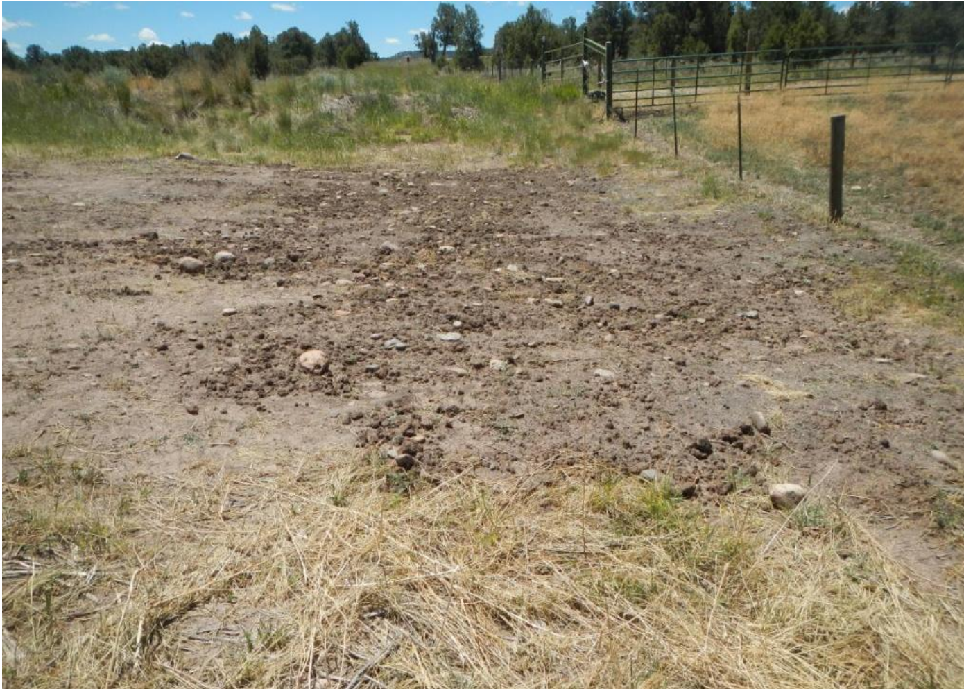
Photo 2. View of area of recent flowline disturbance. This needs to be seeded mulched.
