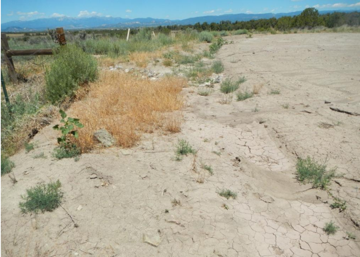
Photo 3. View of the western edge of the project area. Diversion ditch is full of sediment and needs to be cleaned. Erosion from well pad surface is depositing sediment in diversion, as evidenced by erosional channels on the well pad surface and sediment plumes where it settles in diversion channel. Well pad surface needs erosion controls such as gravelling.
