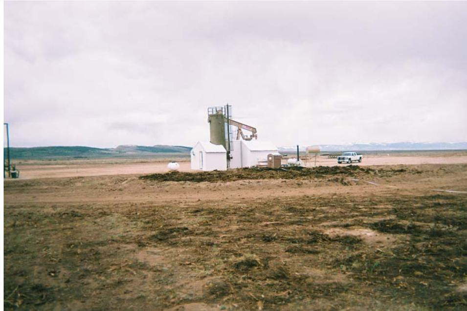
**Subject:** A top valve seal on the vertical separator failed resulting in the January 29, 2012 condensate release. Impacted vegetation and soils were scraped up using a loader and placed within secondary containment to the east of the separator. Stained soils and vegetation are shown in the foreground.
