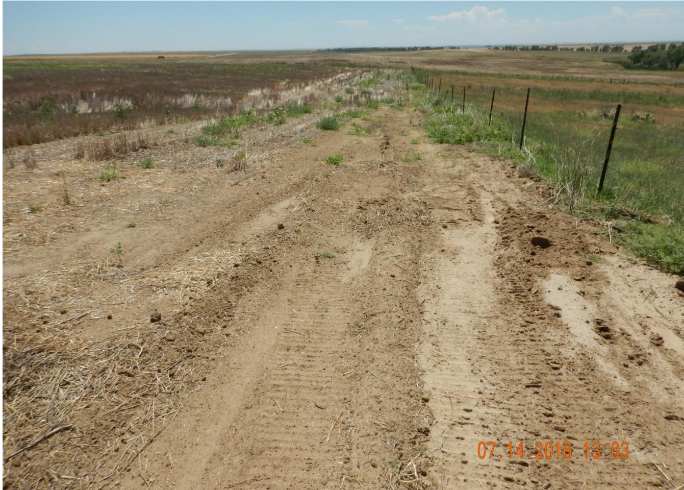
Photo 6. Photo taken from southwest of well location, facing South. Gully from erosion has been filled in.
