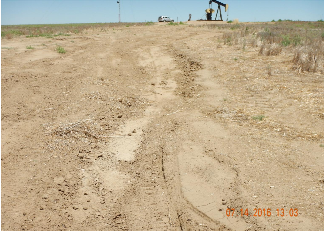
Photo 5. Photo taken from southwest of well location, facing North. Gully from erosion has been filled in.
