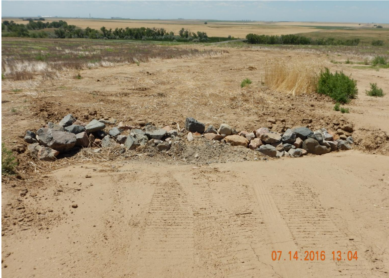
Photo 3. Photo taken from the southern well location, facing West, toward the first BMP. Two stormwater BMPs installed along the southern location to control stormwater and transport of sediment.
