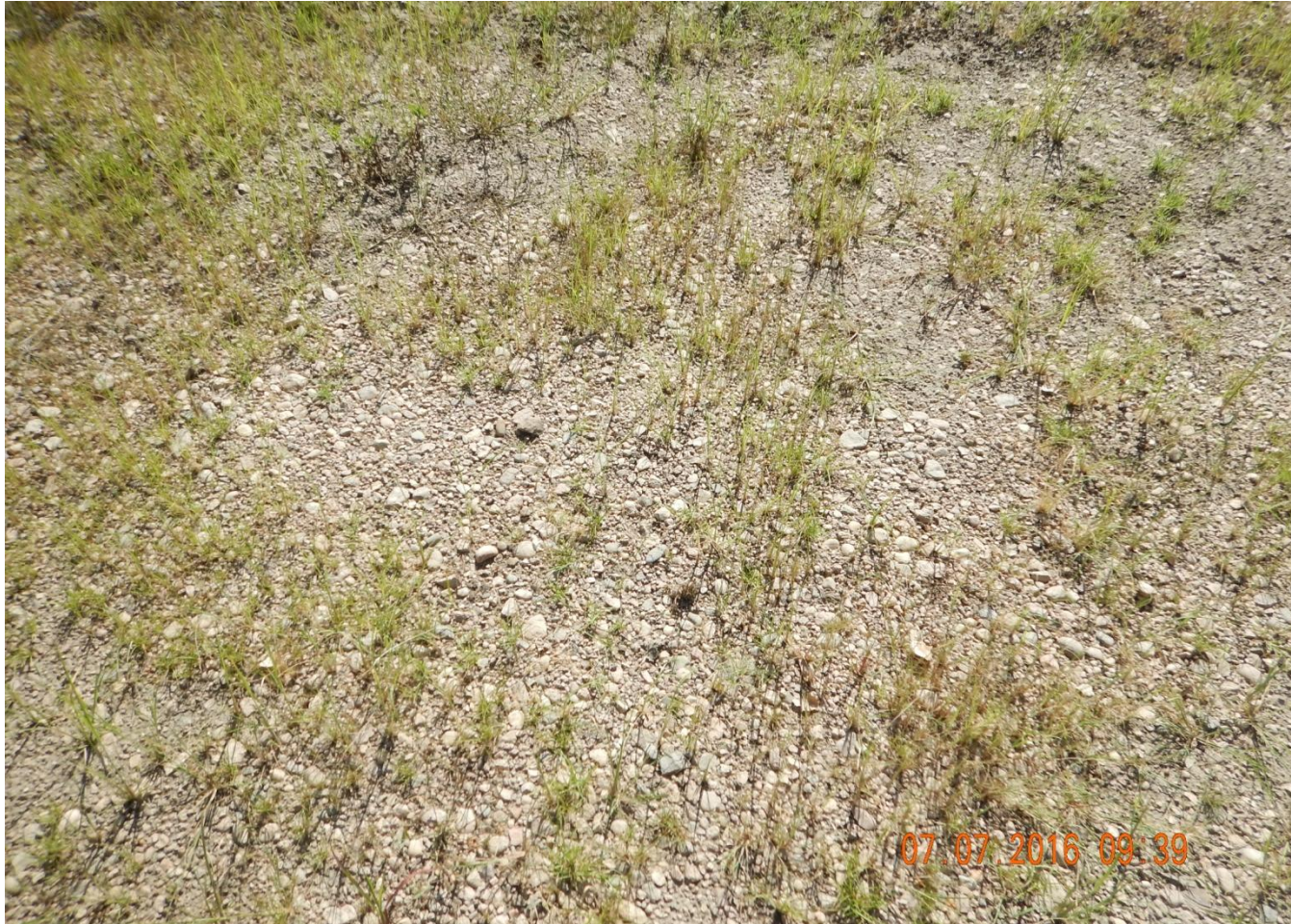
Photo 6. Close up photo taken from the tank battery location, illustrating that gravel has not been removed per Rule 1004.
