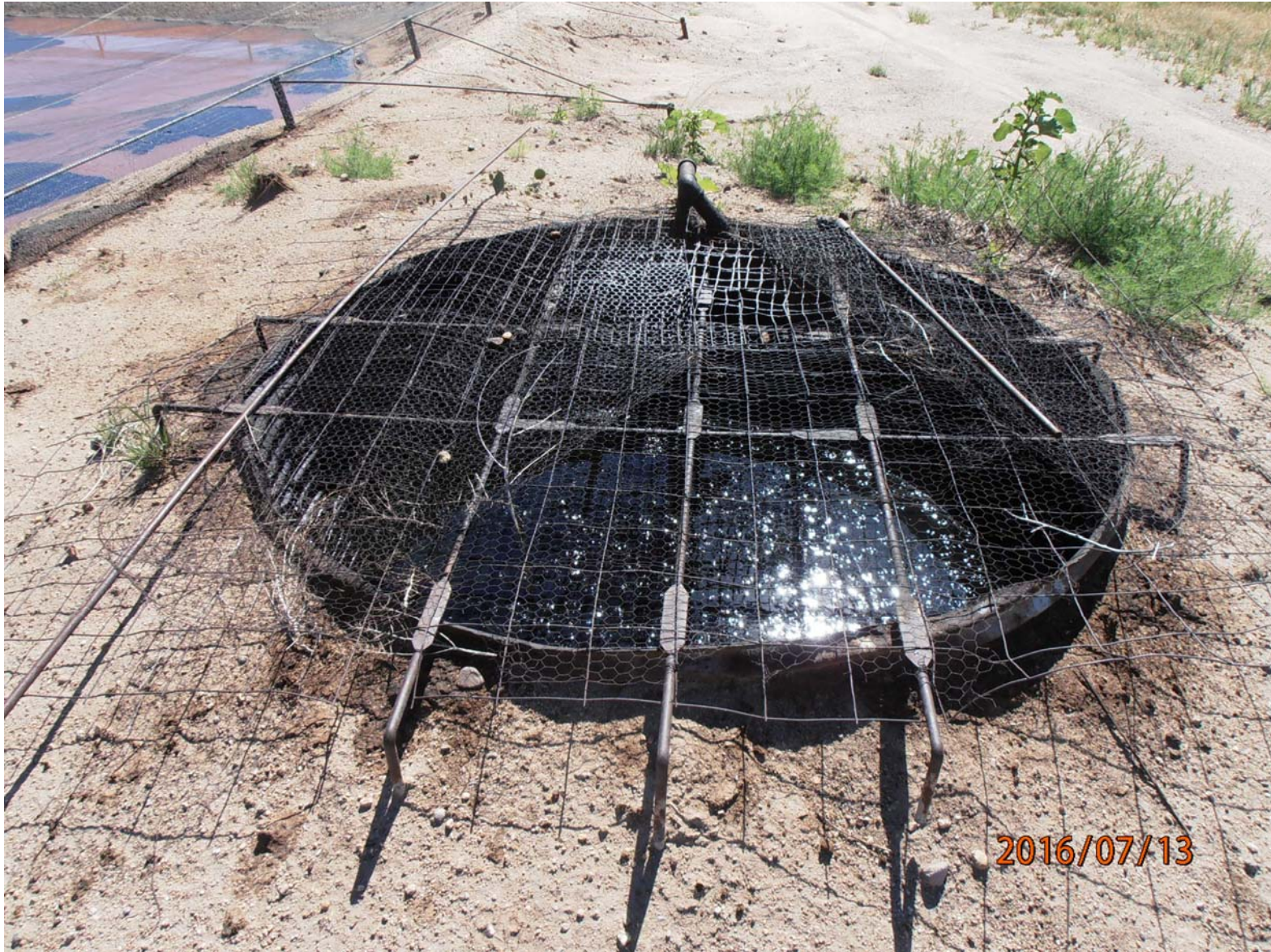
Unlined skim pit (tin horn) located on southwest corner of produced water pit.
