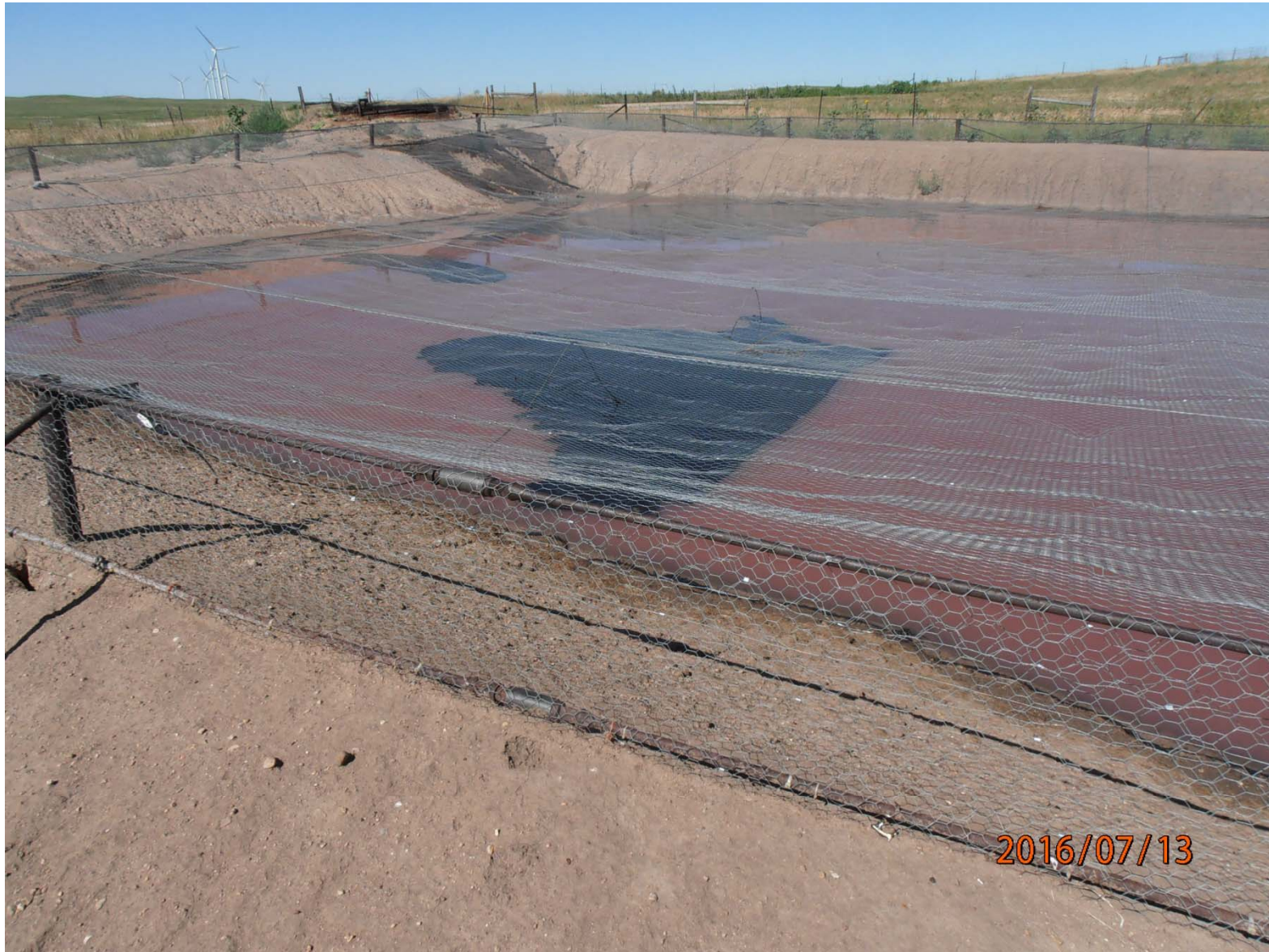
Sag in netting from broken cable is center of picture.
