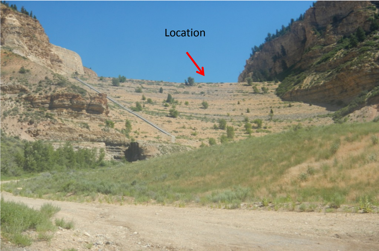
Photo#2: Location site is at top of 300Ft of Fill from Road Construction.
