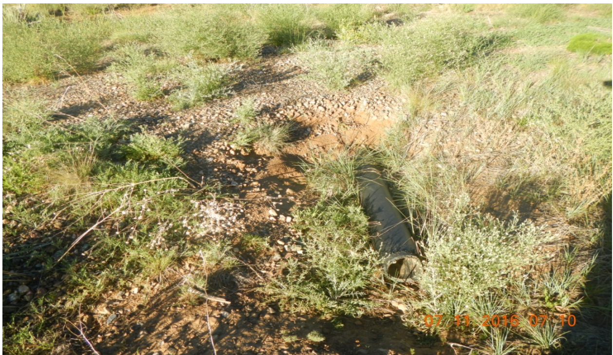
photo 4: A plastic culvert and gravel remains along the access road.
