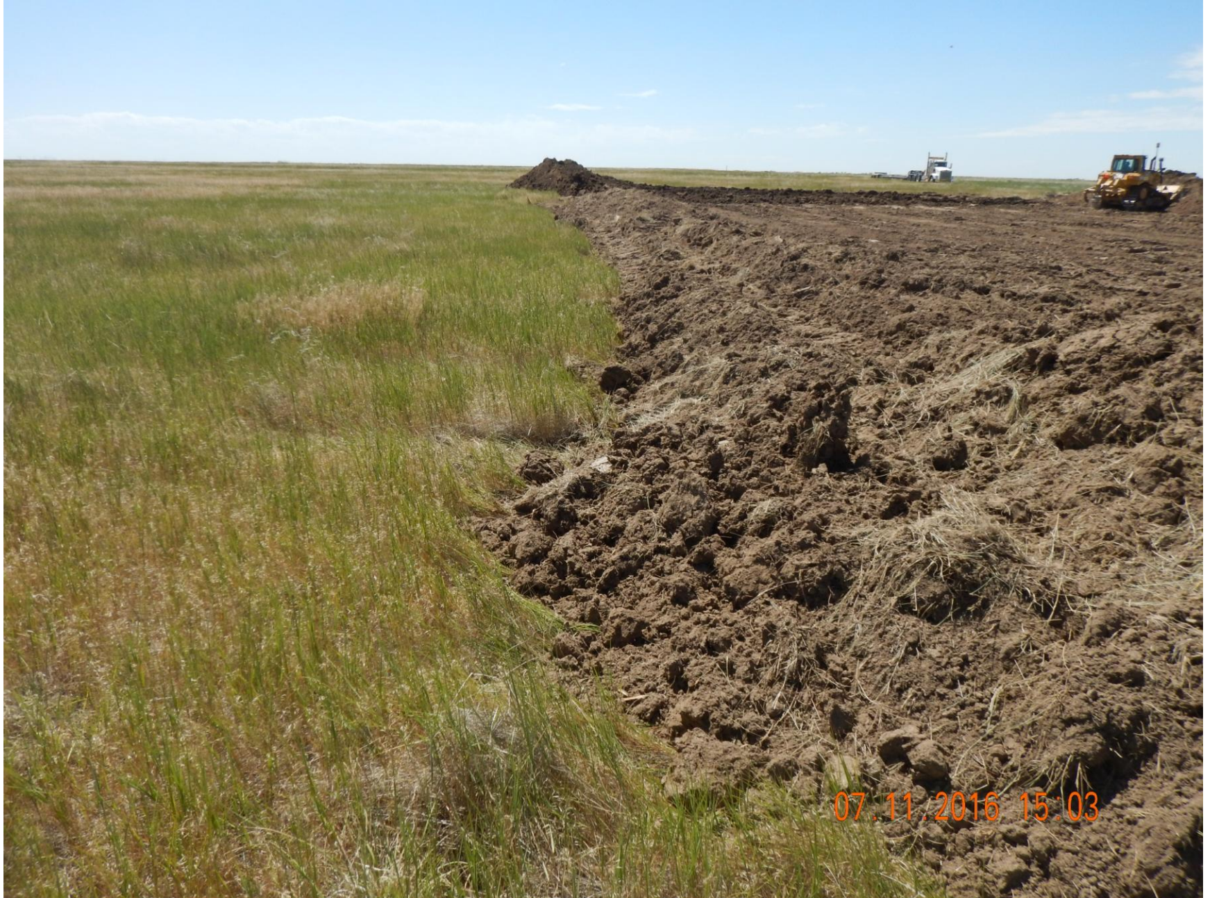
Figure 5: Photo taken from the southeast corner of the location, facing west. Photo shows berms have not been constructed properly; berms along perimeter are not compacted and have either been incorrectly tracked, or not tracked at all.
