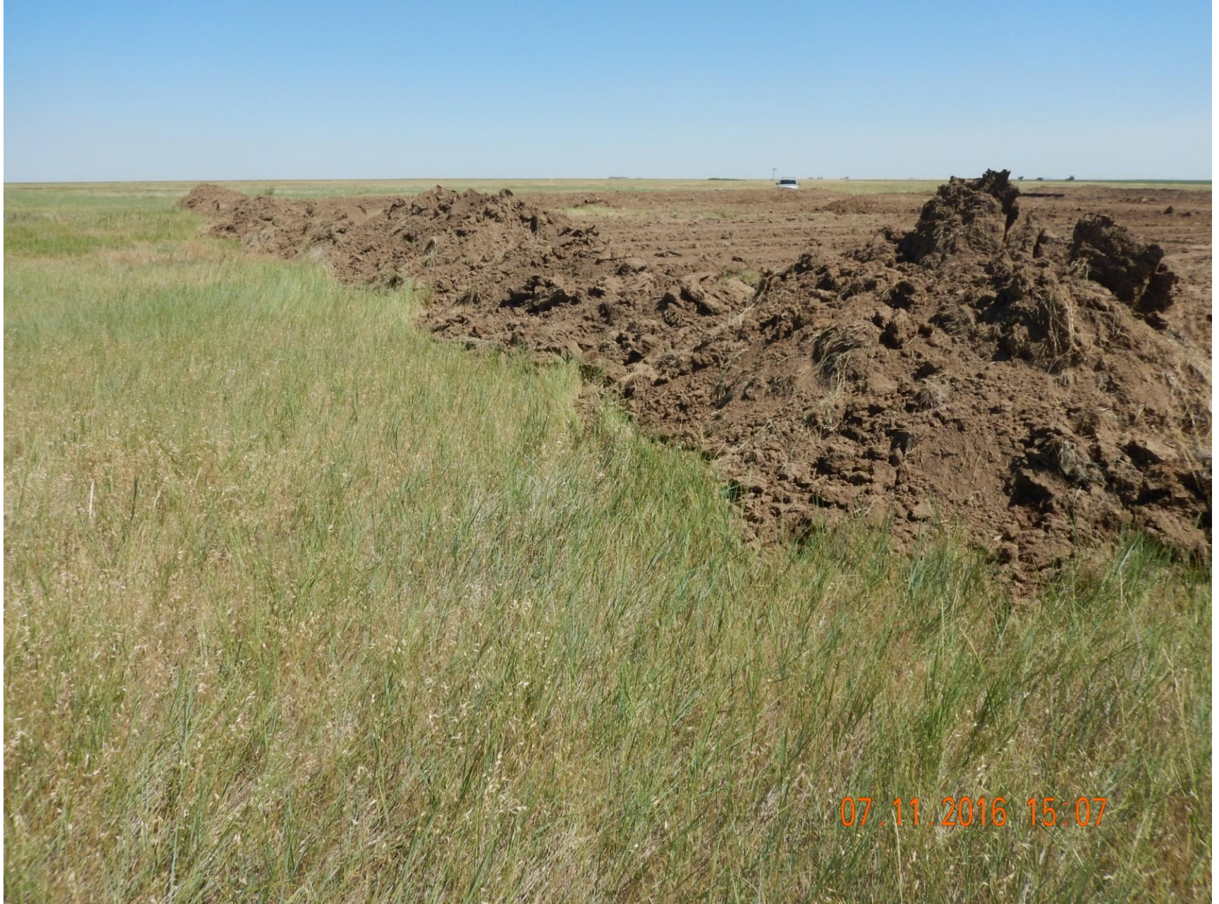
Figure 10: Photo taken from the north end of the location, facing east. Photo shows berms have not been constructed properly; berms along perimeter are not compacted and have either been incorrectly tracked, or not tracked at all.
