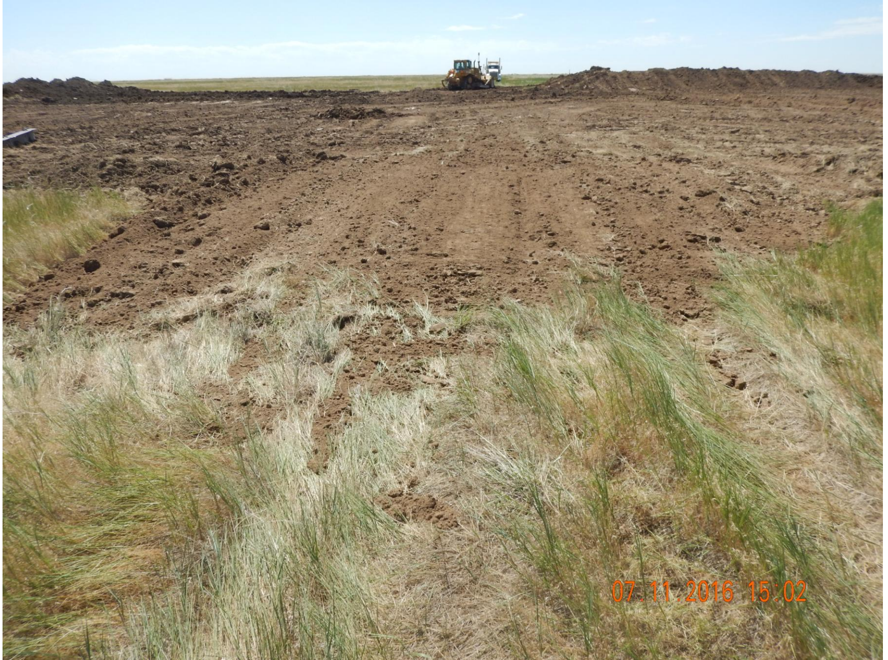
Figure 2: Photo taken from the east end of the location, facing west. Photo shows entrance to location. Note vehicle tracking BMPs absent.
