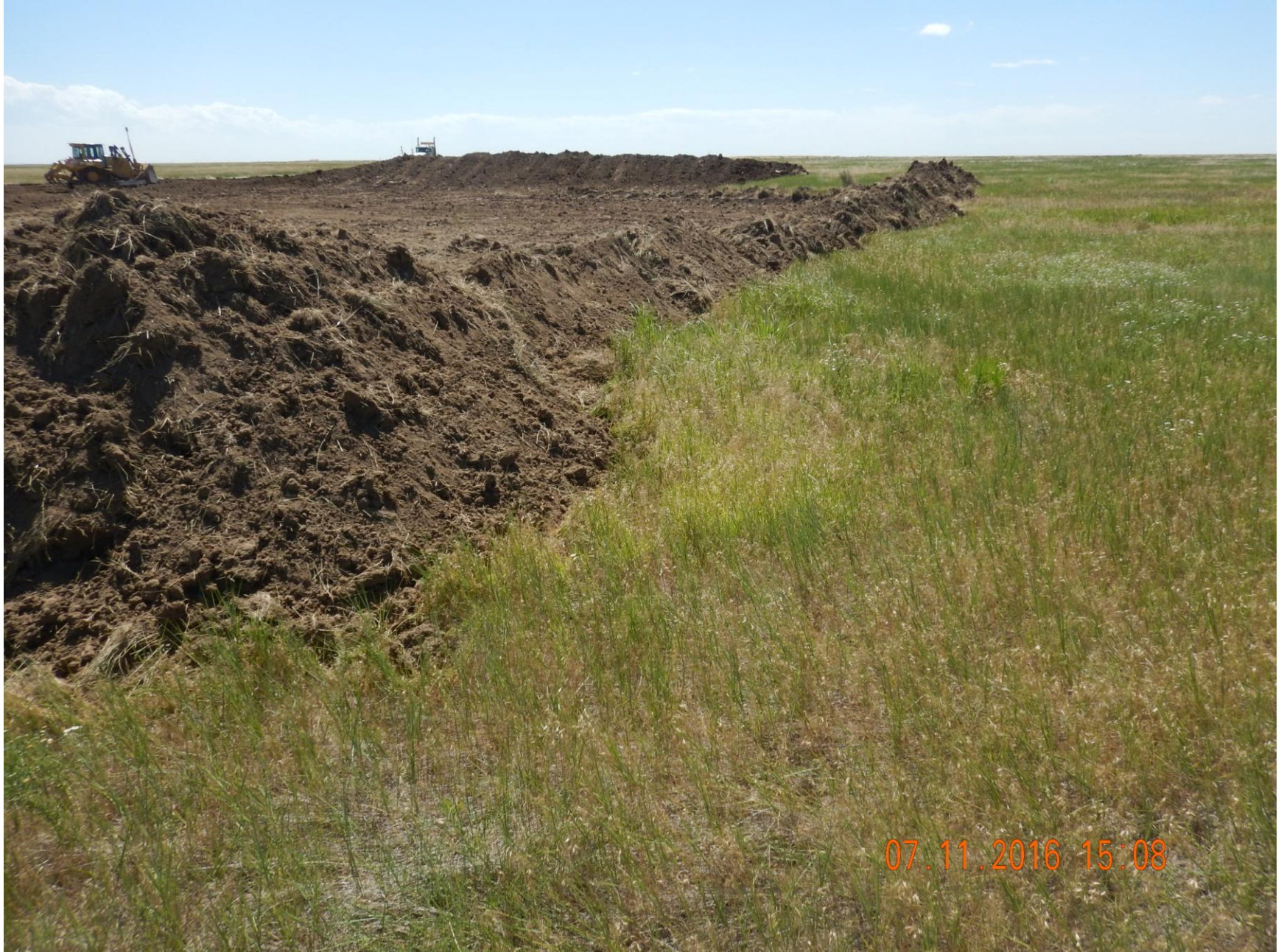
Figure 11: Photo taken from the northeast end of the location, facing west. Photo shows berms have not been constructed properly; berms along perimeter are not compacted and have either been incorrectly tracked, or not tracked at all.
