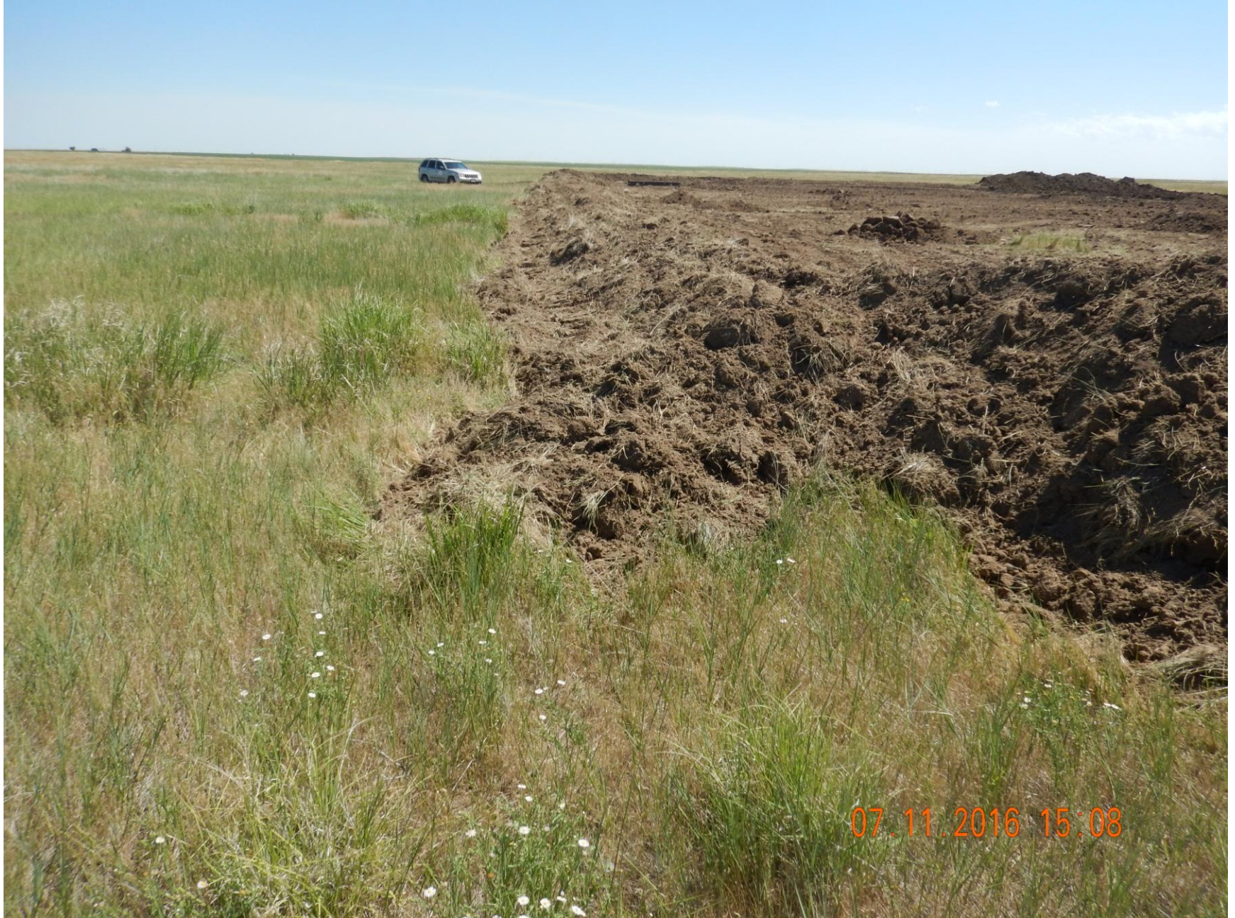
Figure 12: Photo taken from the northeast end of the location, facing south. Photo shows berms have not been constructed properly; berms along perimeter are not compacted and have either been incorrectly tracked, or not tracked at all.
