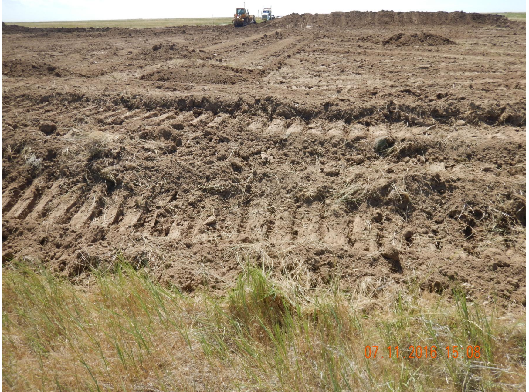
Figure 13: Photo shows perimeter berms have been constructed improperly; berm has been improperly tracked.
