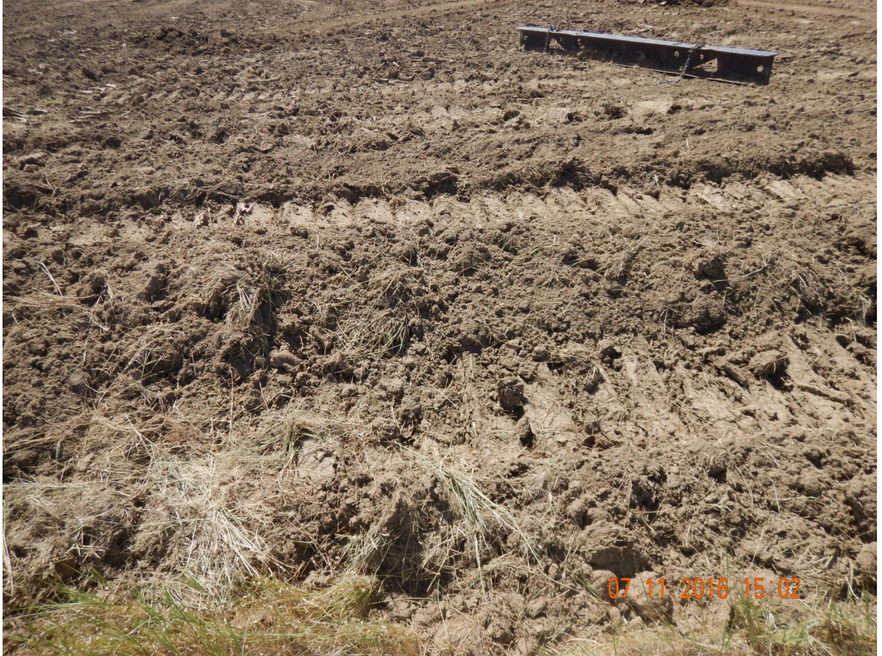
Figure 3: Photo taken from the east end of the location. Photo shows perimeter berms have been constructed improperly; berms along perimeter are not compacted and have either been incorrectly tracked, or not tracked at all.
