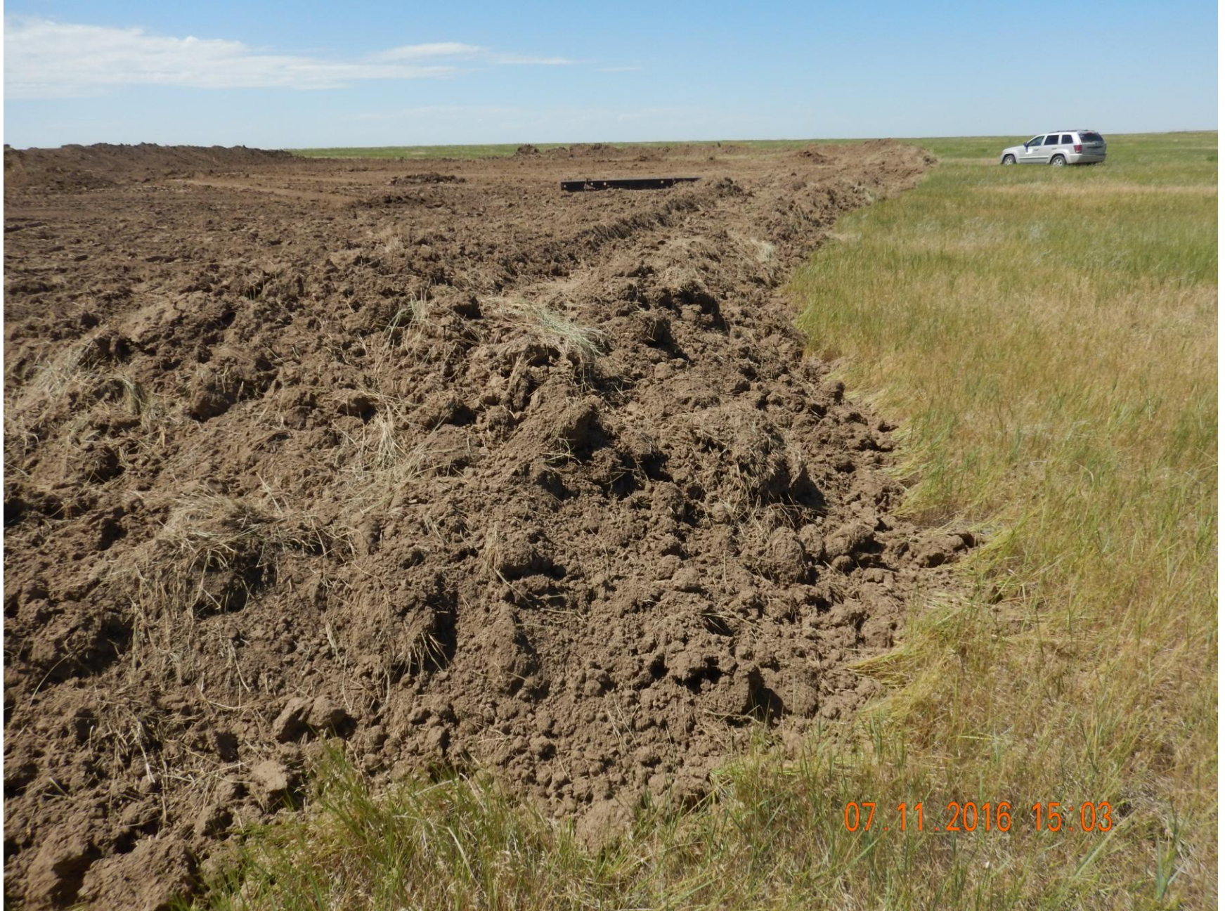
Figure 4: Photo taken from the southeast corner of the location, facing north. Photo shows berms have not been constructed properly; berms along perimeter are not compacted and have either been incorrectly tracked, or not tracked at all.
