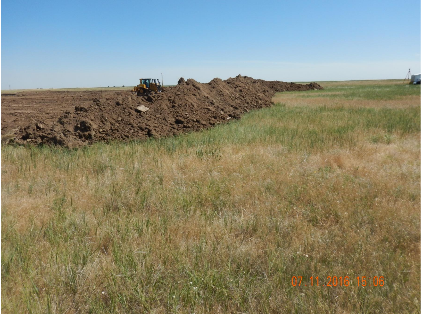
Figure 8: Photo taken from the northwest corner of the location, facing south. Photo shows portion of the topsoil pile. No stormwater or sediment control BMPs in place.
