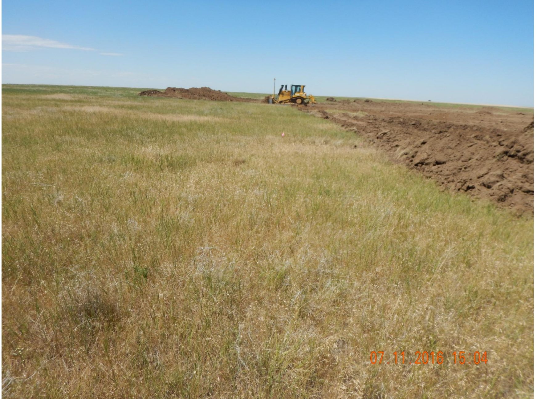
Figure 7: Photo taken from the southwest corner of the location, facing north. Photo shows portion of the topsoil pile. No stormwater or sediment control BMPs in place.
