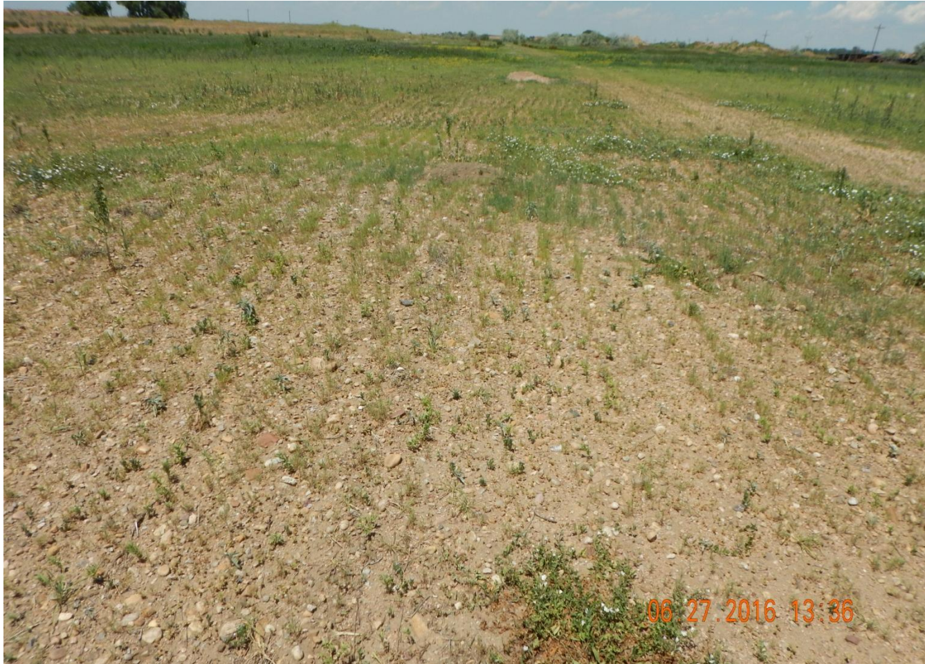
Photo 4. Photo taken from well location, facing North. Need to reclaim location per Rule 1004. A seeding attempt was made but gravel was not removed preventing proper vegetative establishment.
