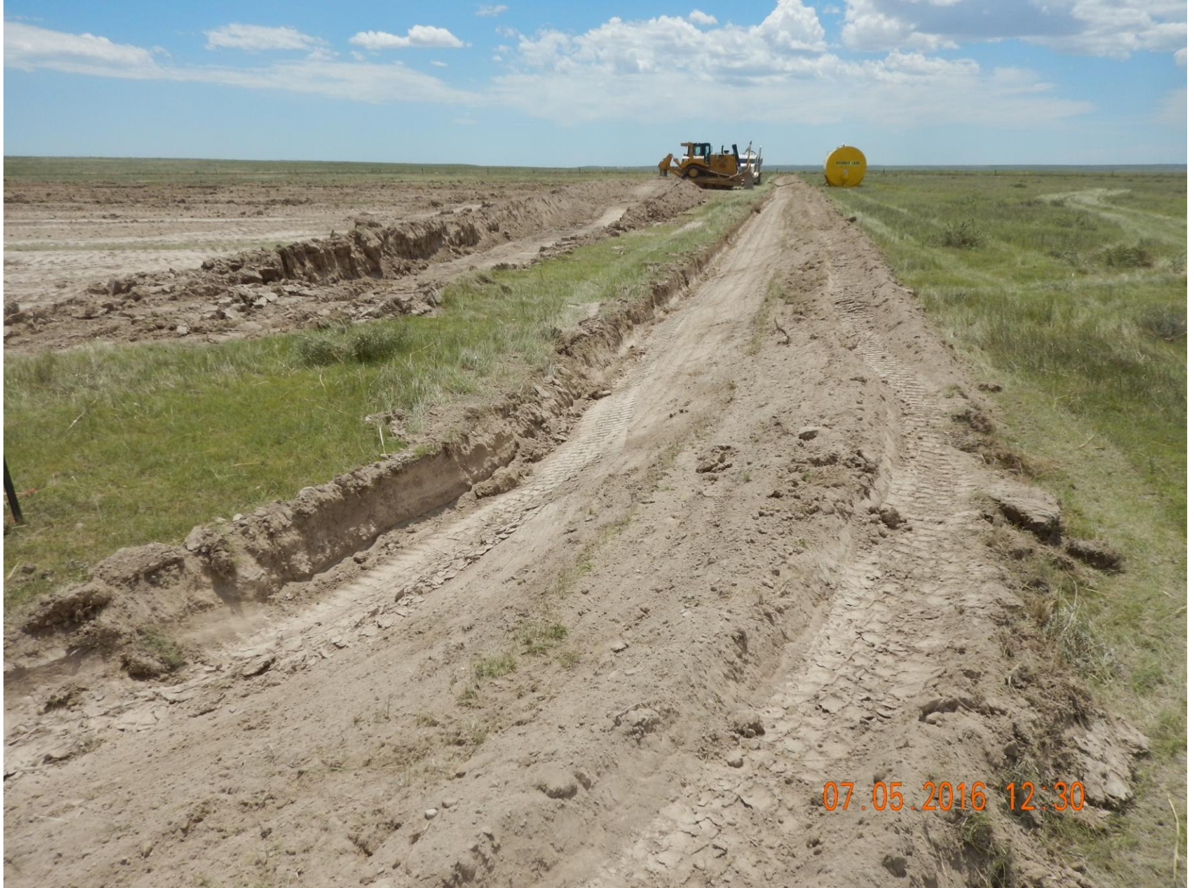
Figure 8: Photo taken from the northwest end of the location, facing south. Photo shows stormwater control ditch around perimeter of the location.
