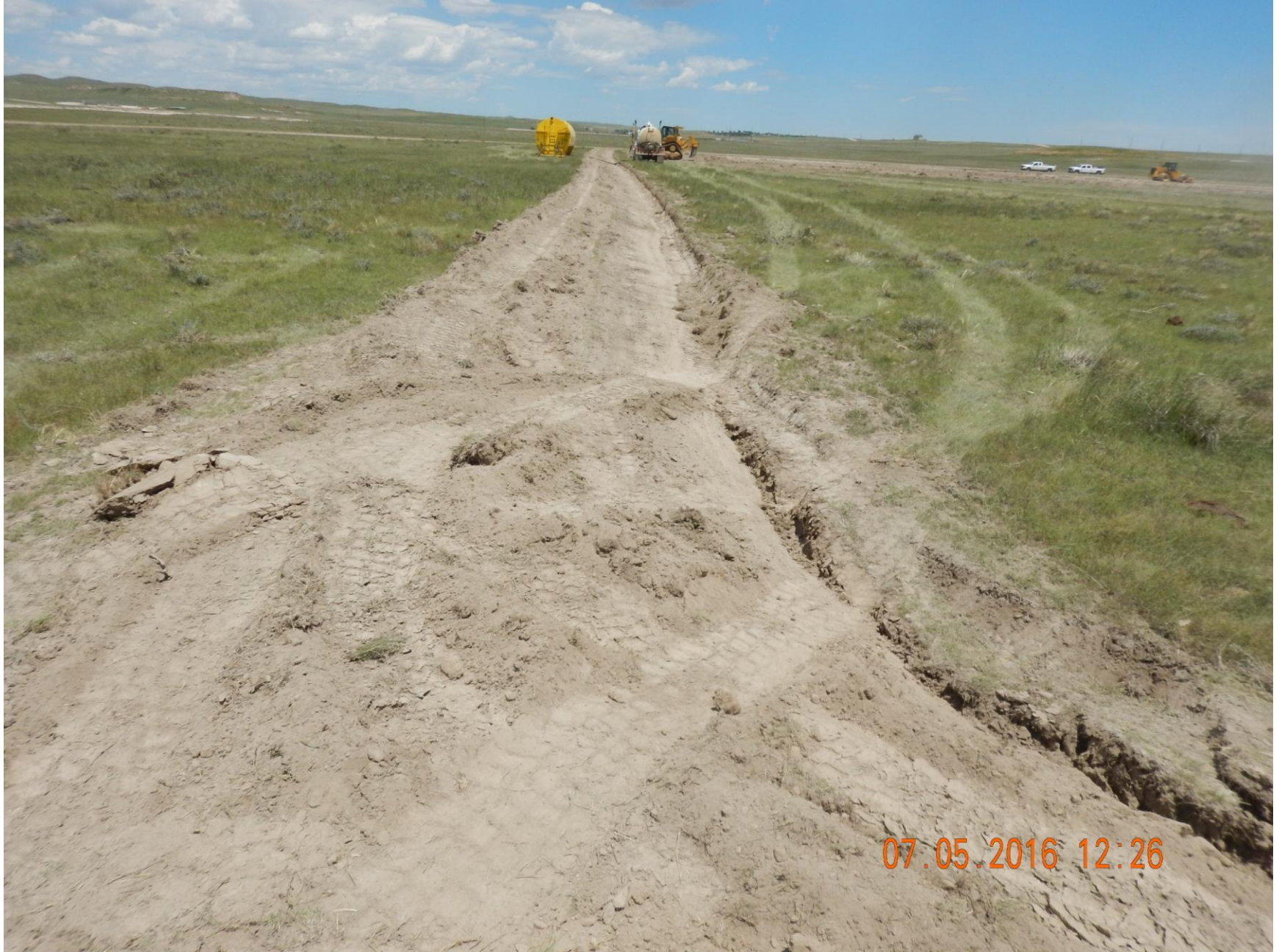
Figure 7: Photo taken from the southwest end of the location, facing north. Photo shows stormwater control ditch around perimeter of the location.
