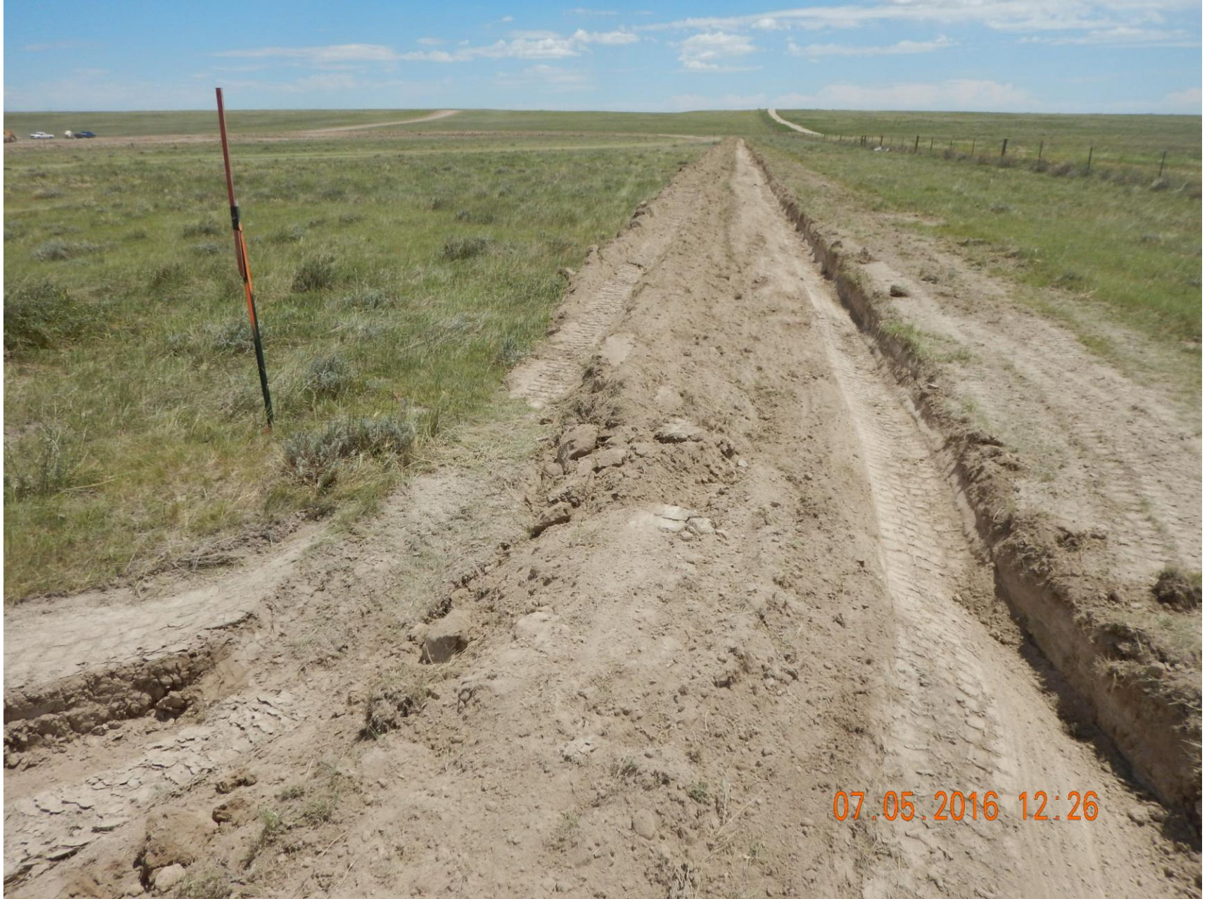
Figure 6: Photo taken from the southwest end of the location, facing east. Photo shows stormwater control ditch around perimeter of the location.
