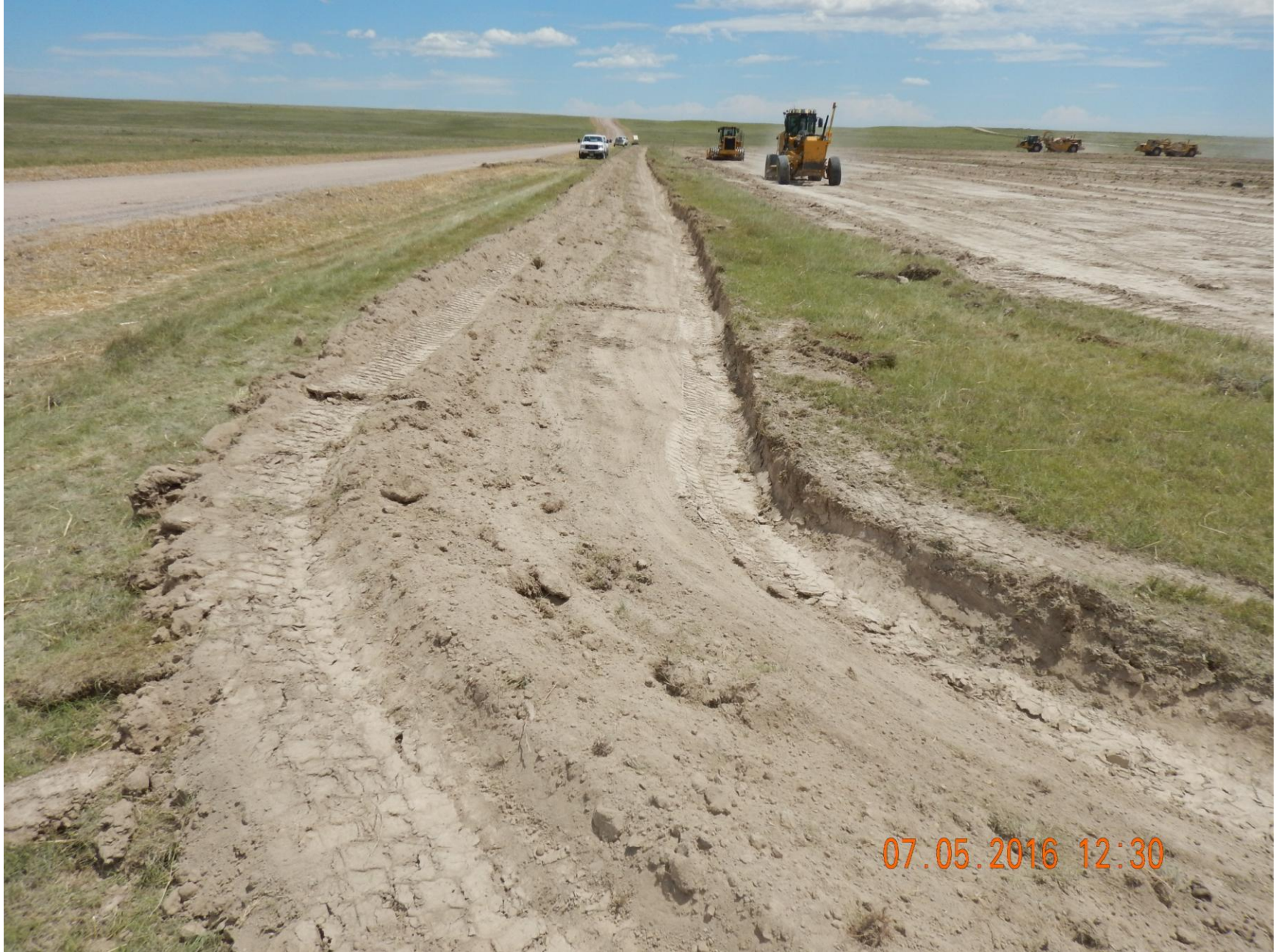
Figure 9: Photo taken from the northwest end of the location, facing east. Photo shows stormwater control ditch around perimeter of the location.
