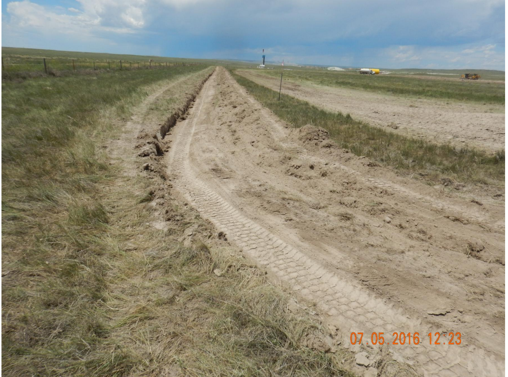
Figure 5: Photo taken from the southeast end of the location, facing west. Photo shows stormwater control ditch around perimeter of the location.
