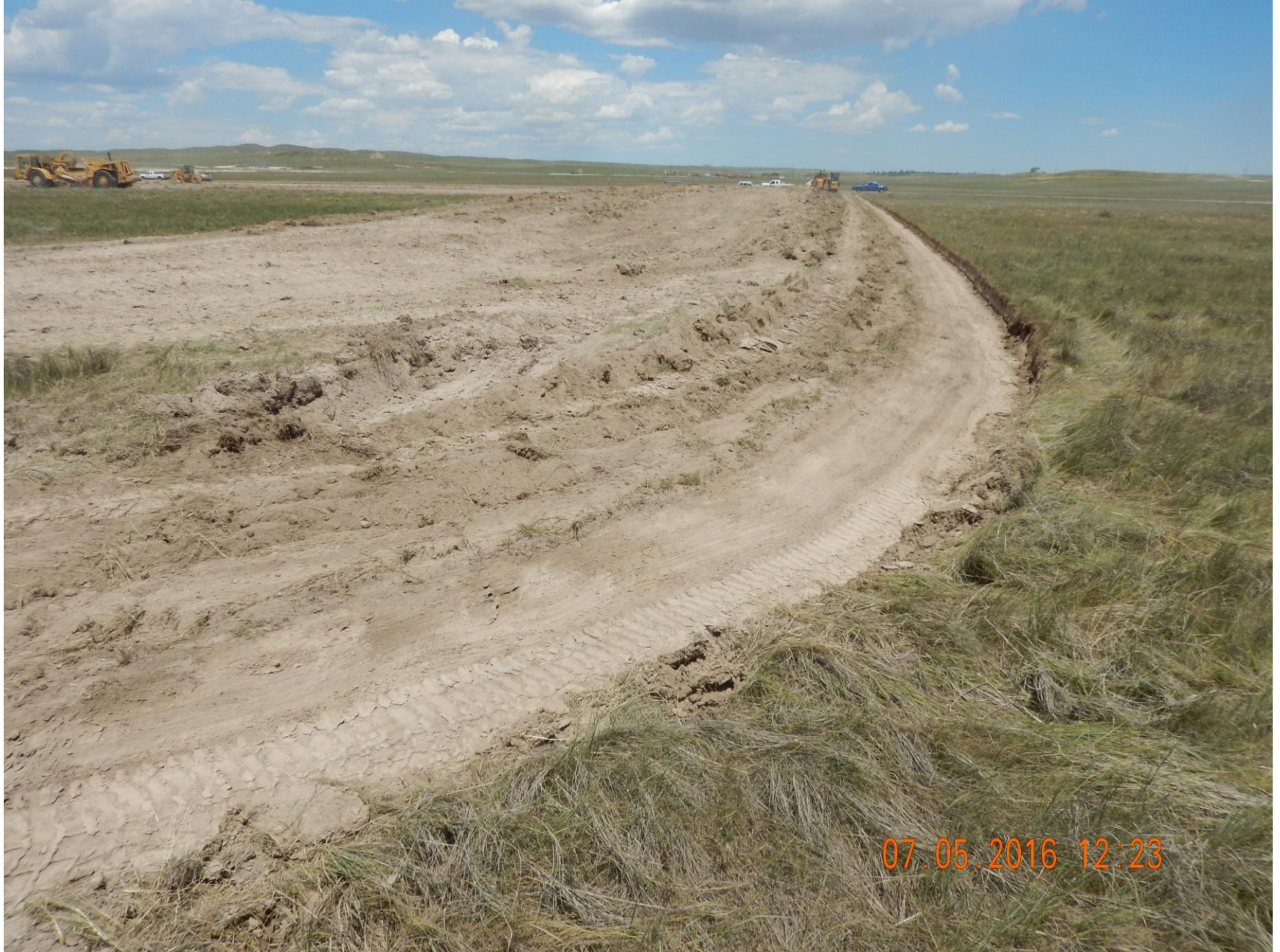
Figure 4: Photo taken from the southeast end of the location, facing north. Photo shows stormwater control ditch around perimeter of the location.
