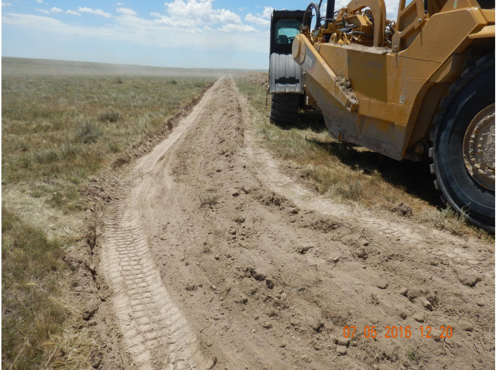
Figure 2: Photo taken from the northeast end of the location, facing south. Photo shows stormwater control ditch around perimeter of the location.
