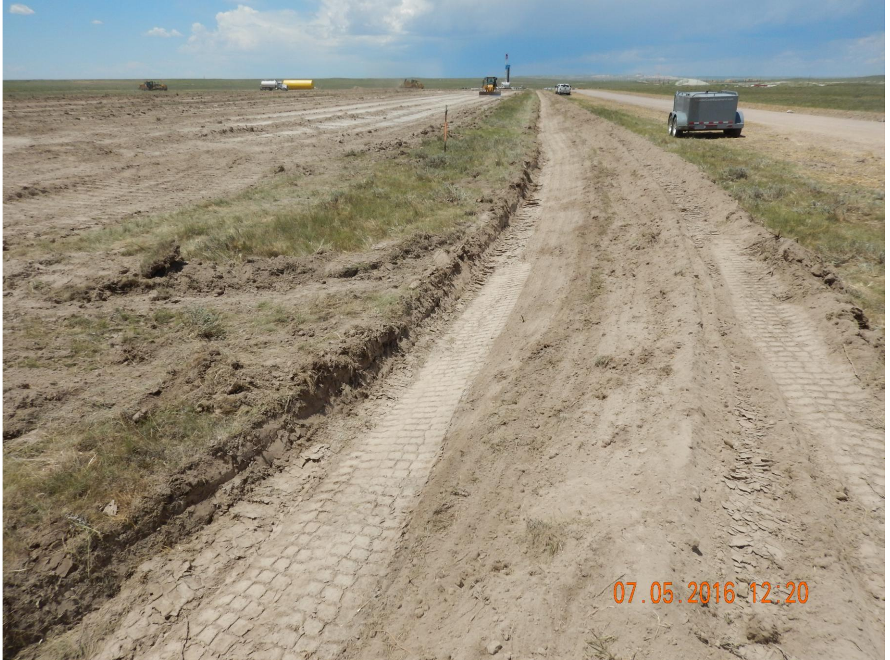
Figure 1: Photo taken from the northeast end of the location, facing west. Photo shows stormwater control ditch around perimeter of the location.
