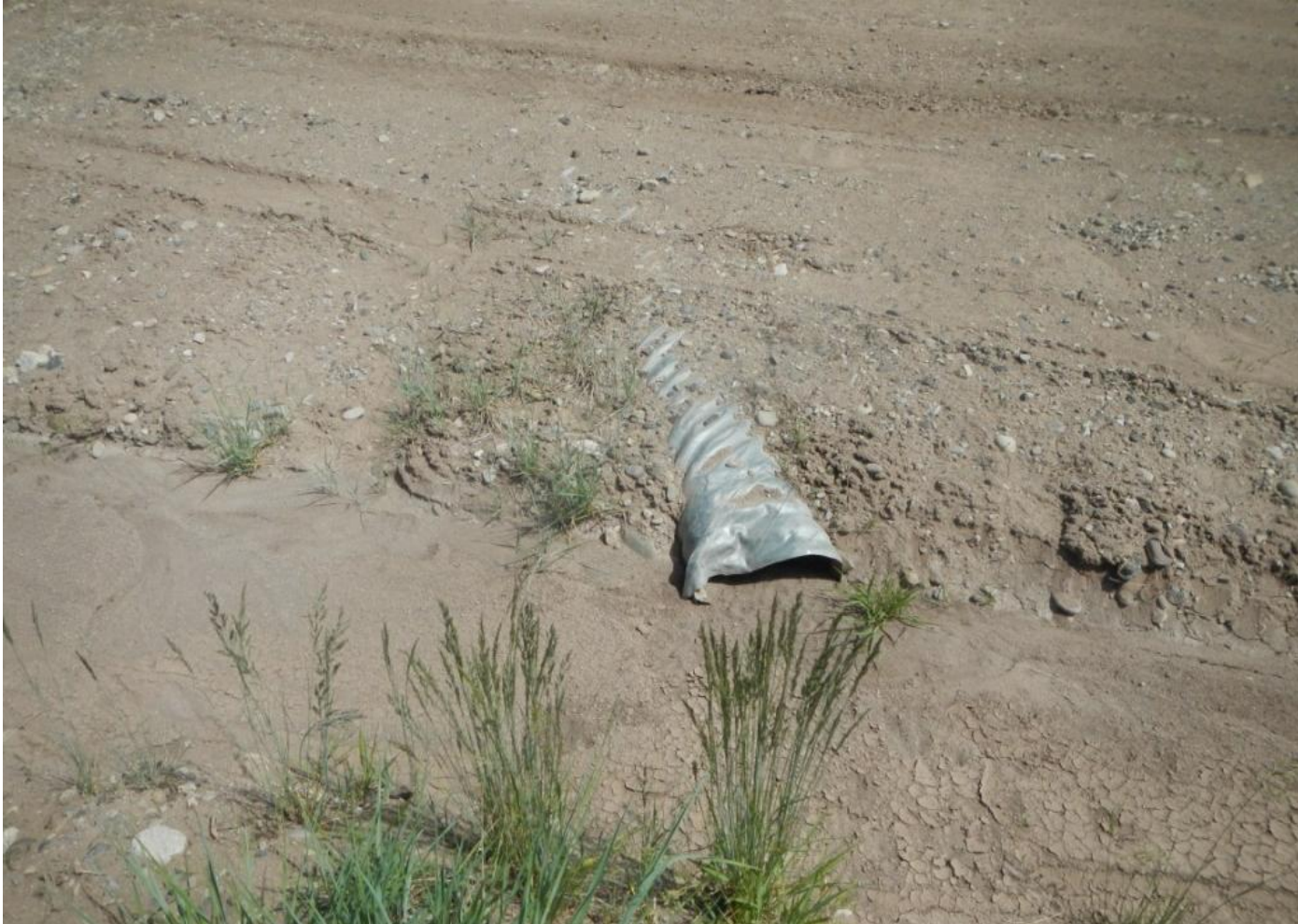
Photo 6. View of culvert at the entrance to the access road that is damaged and full of sediment. Culvert needs maintenance and repair.
