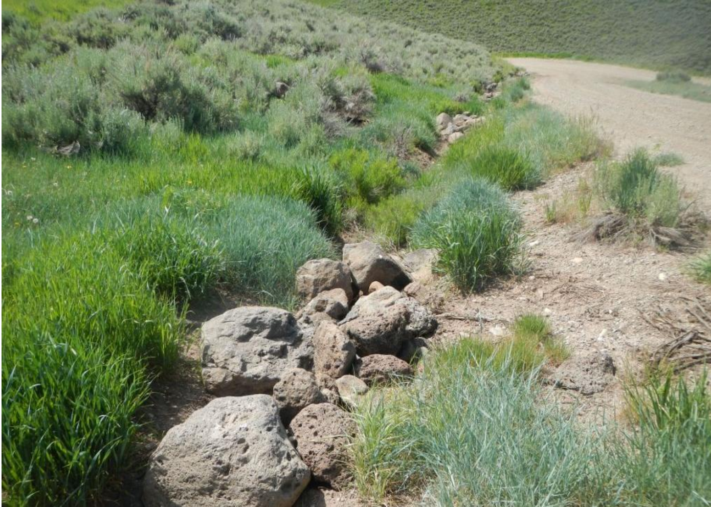
Photo 5. View of roadside ditch along access road from well pad facing toward entrance. Rock check dams are being used to de-energize flows.
