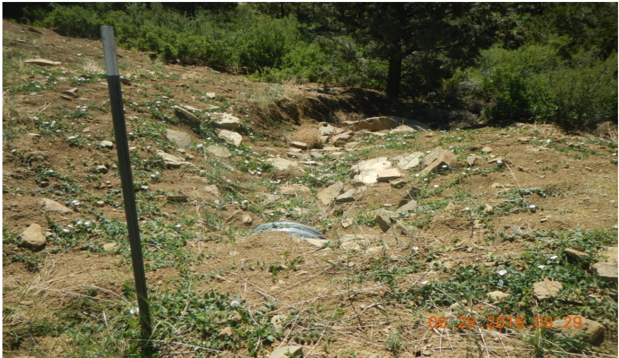
photo 9: There are signs of erosion on the outlet of the culvert. No stormwater outlet protection.
