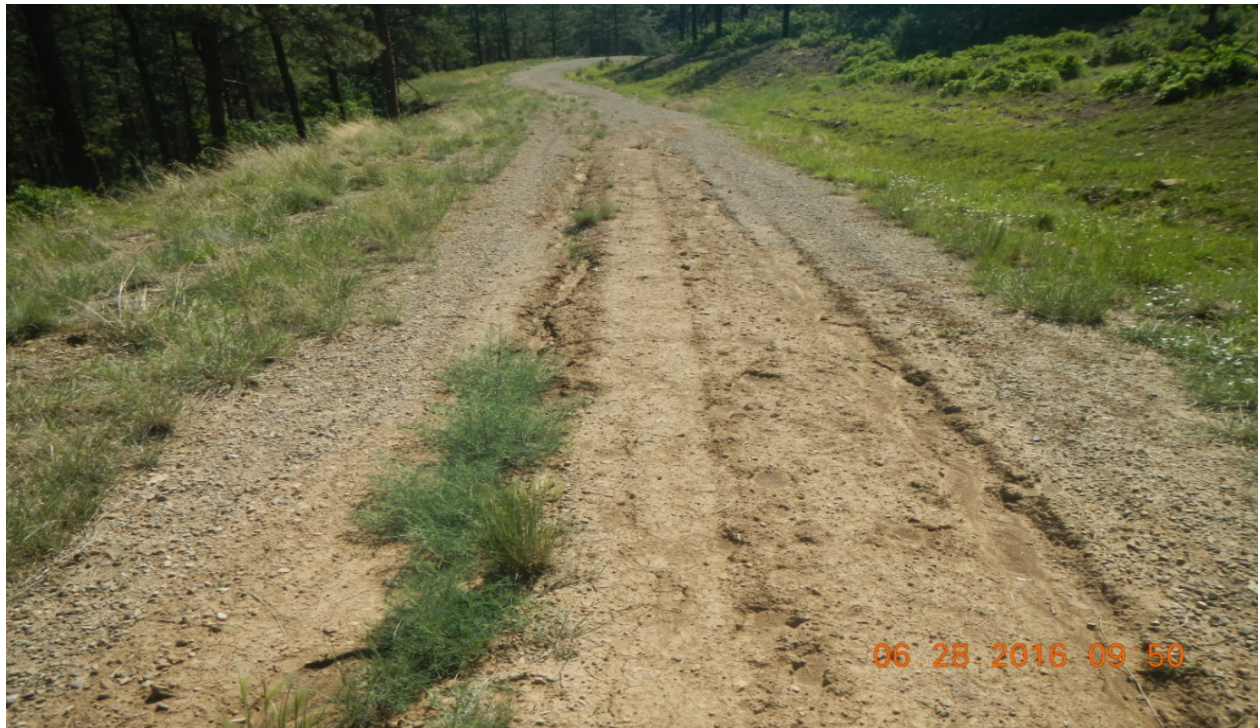
photo 19: Facing northeast along the access road. Signs of erosion can be seen along the access road.
