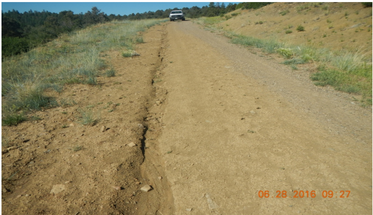
photo 10: Facing back toward the southwest along the access road. Signs of erosion are shown along the road.
