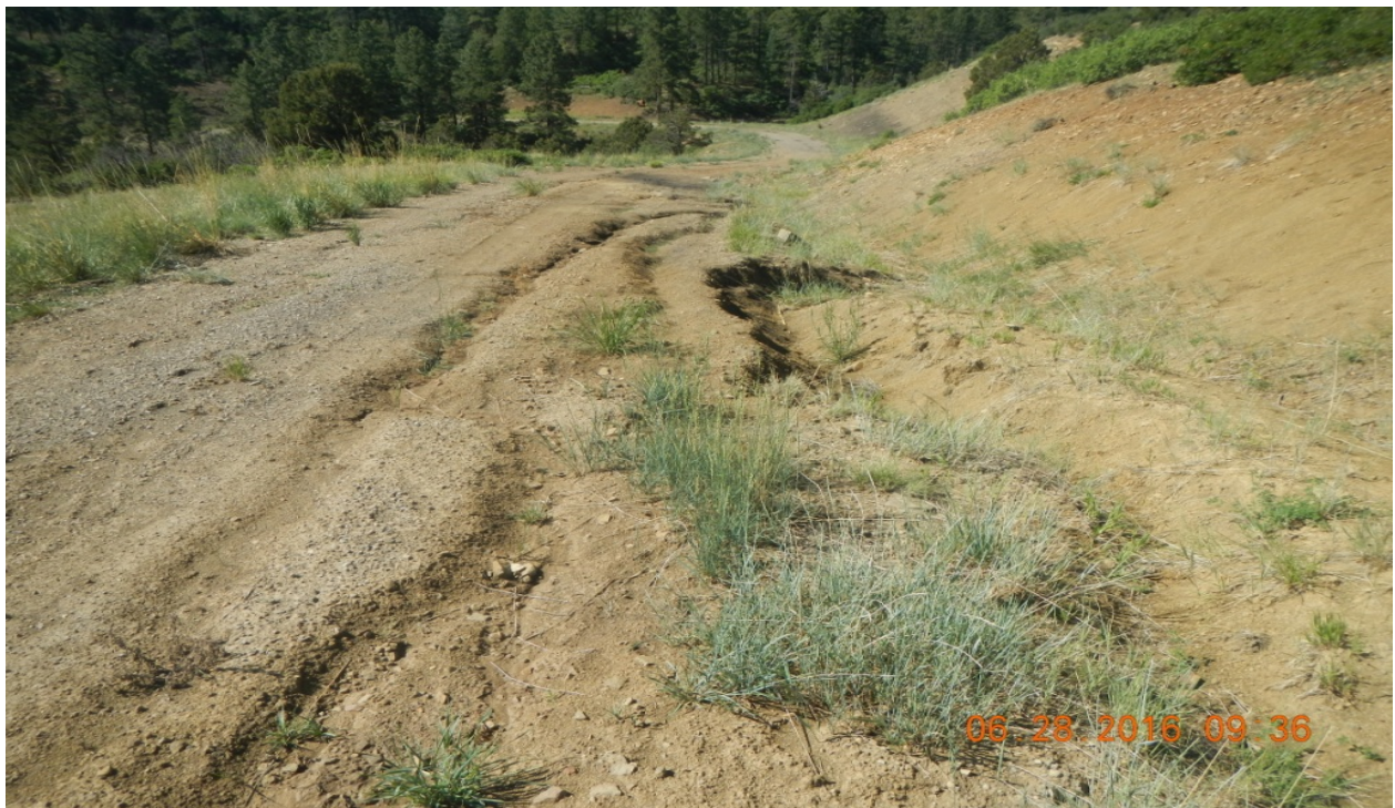
photo 12: Facing southeast along the access road. Erosion channels have developed along the road.
