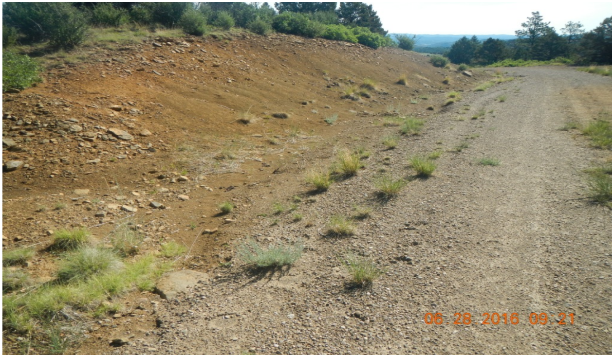
photo 5: The cut side along the access road does not have vegetation establishment.
