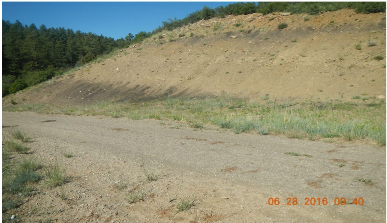
photo 14: Facing toward the cut side along the access road which is not adequately stabilized with vegetation.
