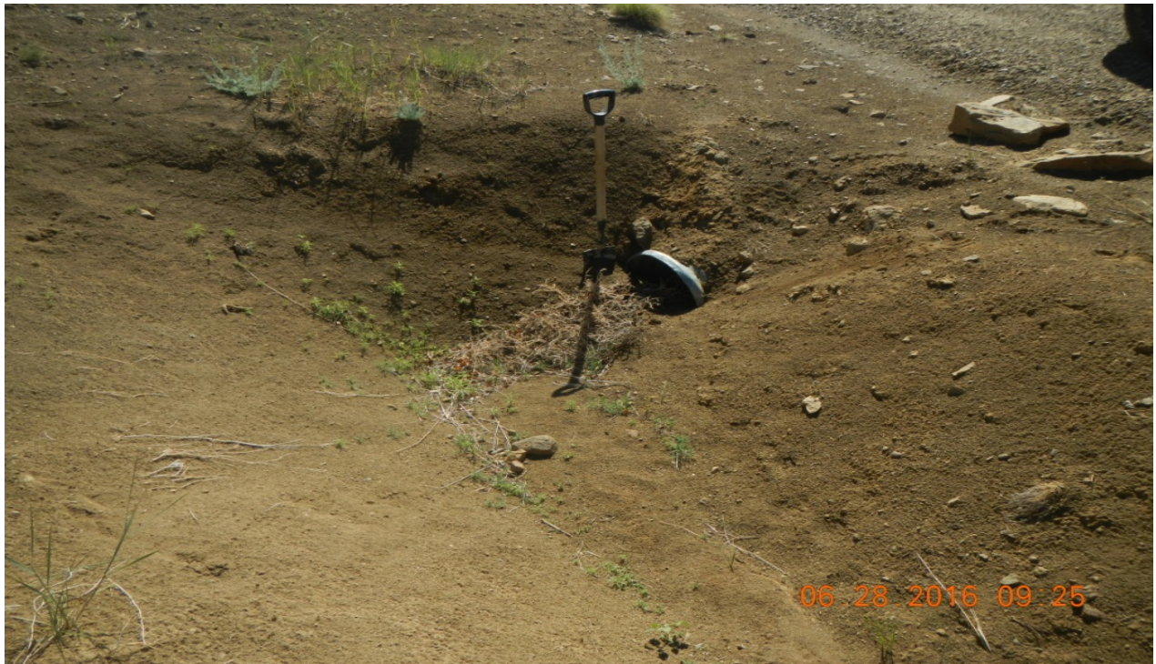
photo 7: A culvert is approximately half full of sediment. (Lat/Long: 37.089,-104.83053)
