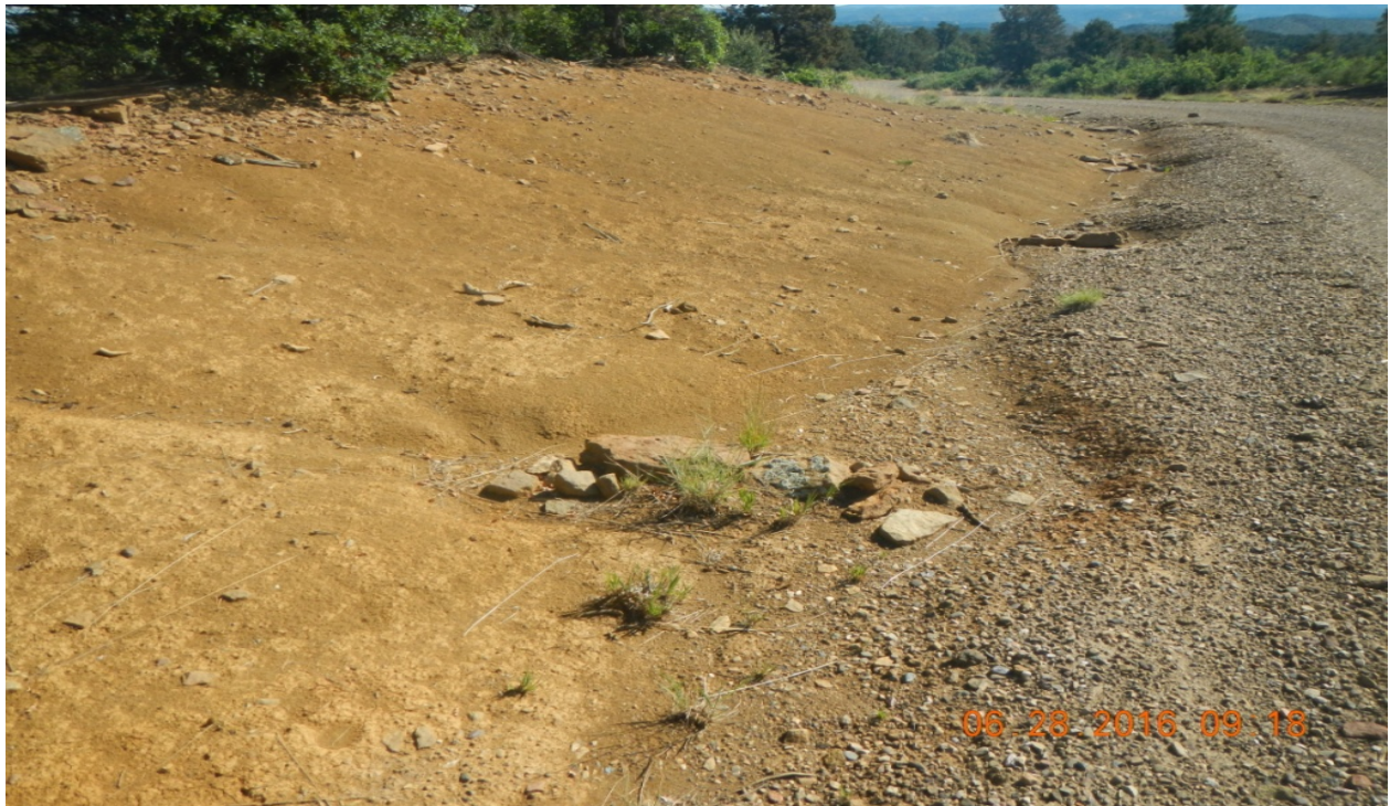
photo 3: Facing toward the side of the access road which is not stabilized with vegetation. What appears to be rock check dams have not been maintained.
