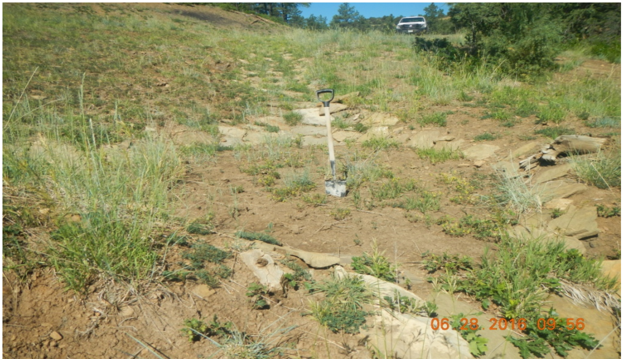
photo 22: There were two sediment traps at the north and northeast side of the location which are full of sediment as shown in this photo.
