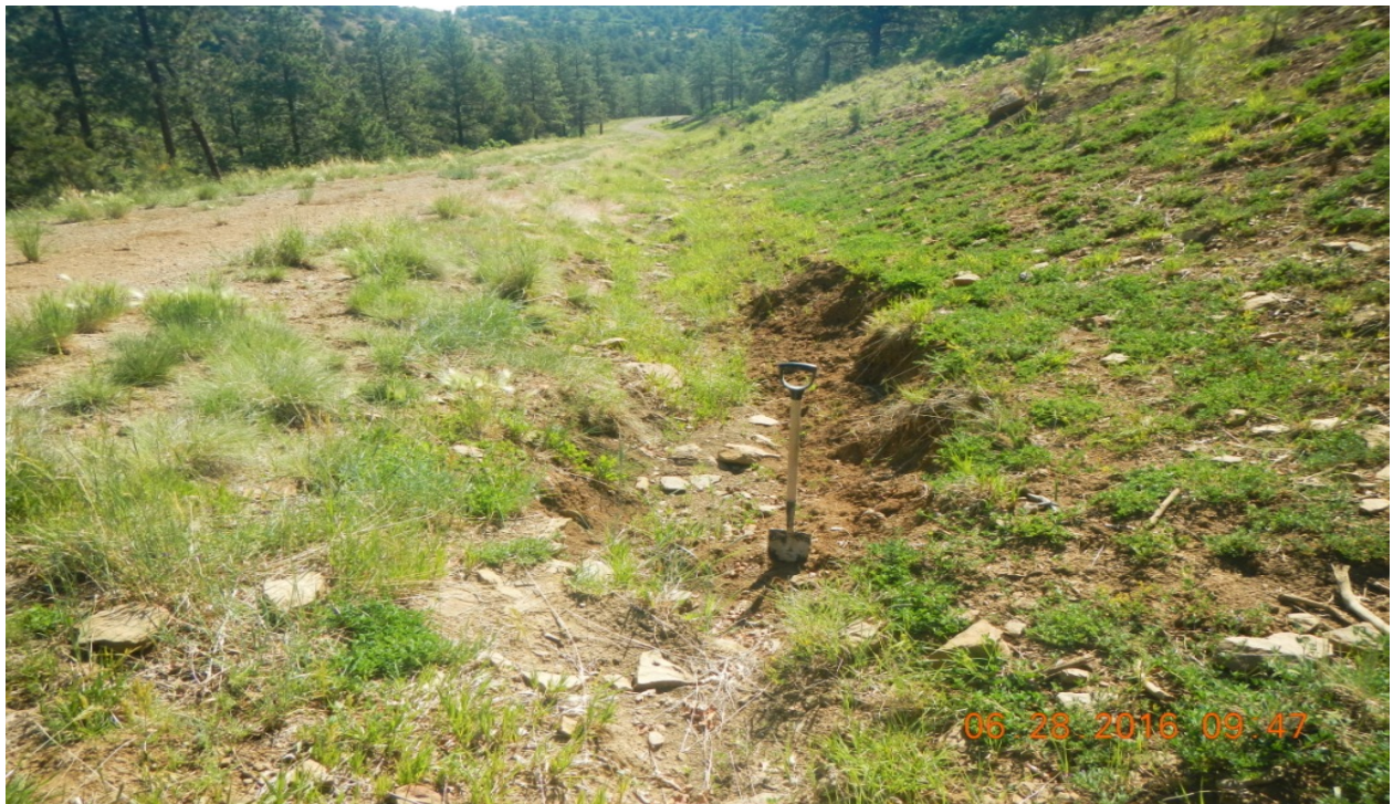
photo 18: Area of erosion noticed along the access road.
