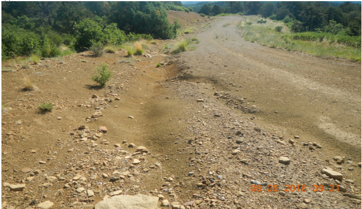
photo 4: Facing northeast along the access road. There are signs of erosion shown in the photo.
