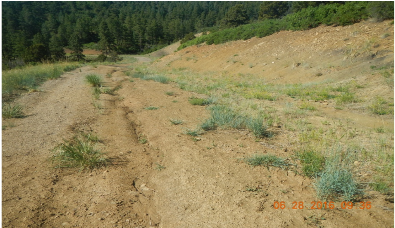
photo 11: Facing southeast along the access road. Vegetation is not established along the cut slope of the road.
