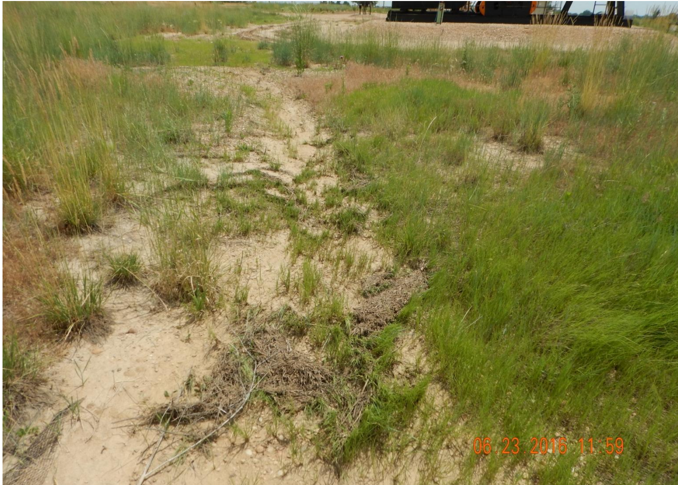
Photo 6. Photo taken from the northwest location, facing East. Need to install sufficient stormwater and sediment control BMPs.
