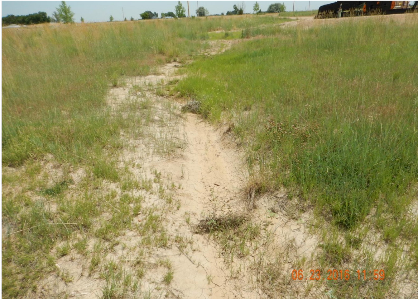
Photo 7. Photo illustrating gulley forming off location and transporting sediment offsite. Need to install sufficient stormwater and sediment control BMPs.
