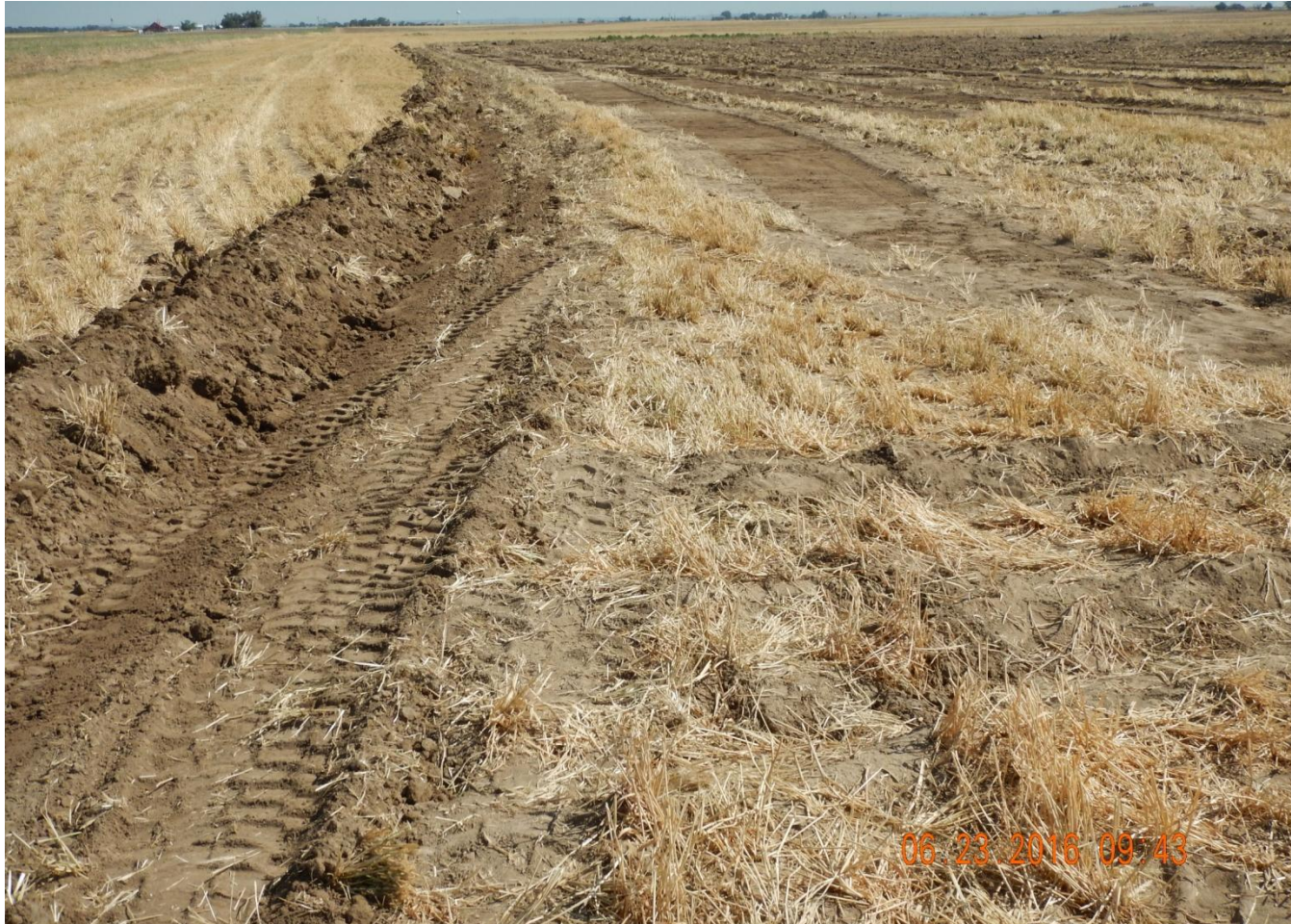
Photo 2. Photo taken from southwest location, facing North. BMP installed around perimeter of location. Operator said berms will be compacted and BMP would be finished on eastern side once landowner moves equipment.
