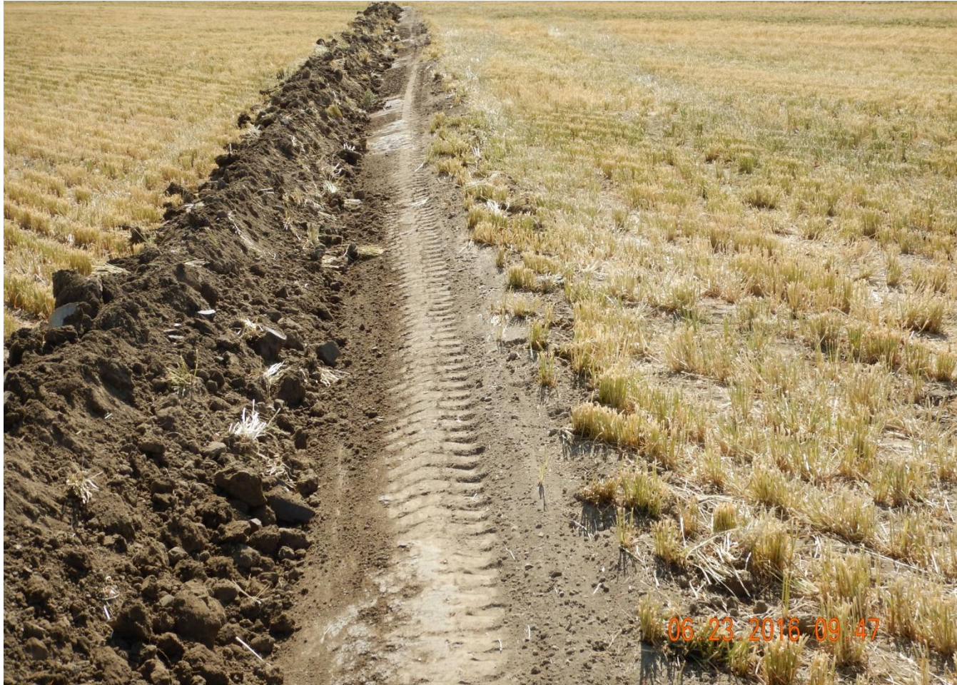
Photo 4. Photo taken from northern location, facing East. BMP installed around perimeter of location. Operator said berms will be compacted and BMP would be finished on eastern side once landowner moves equipment.
