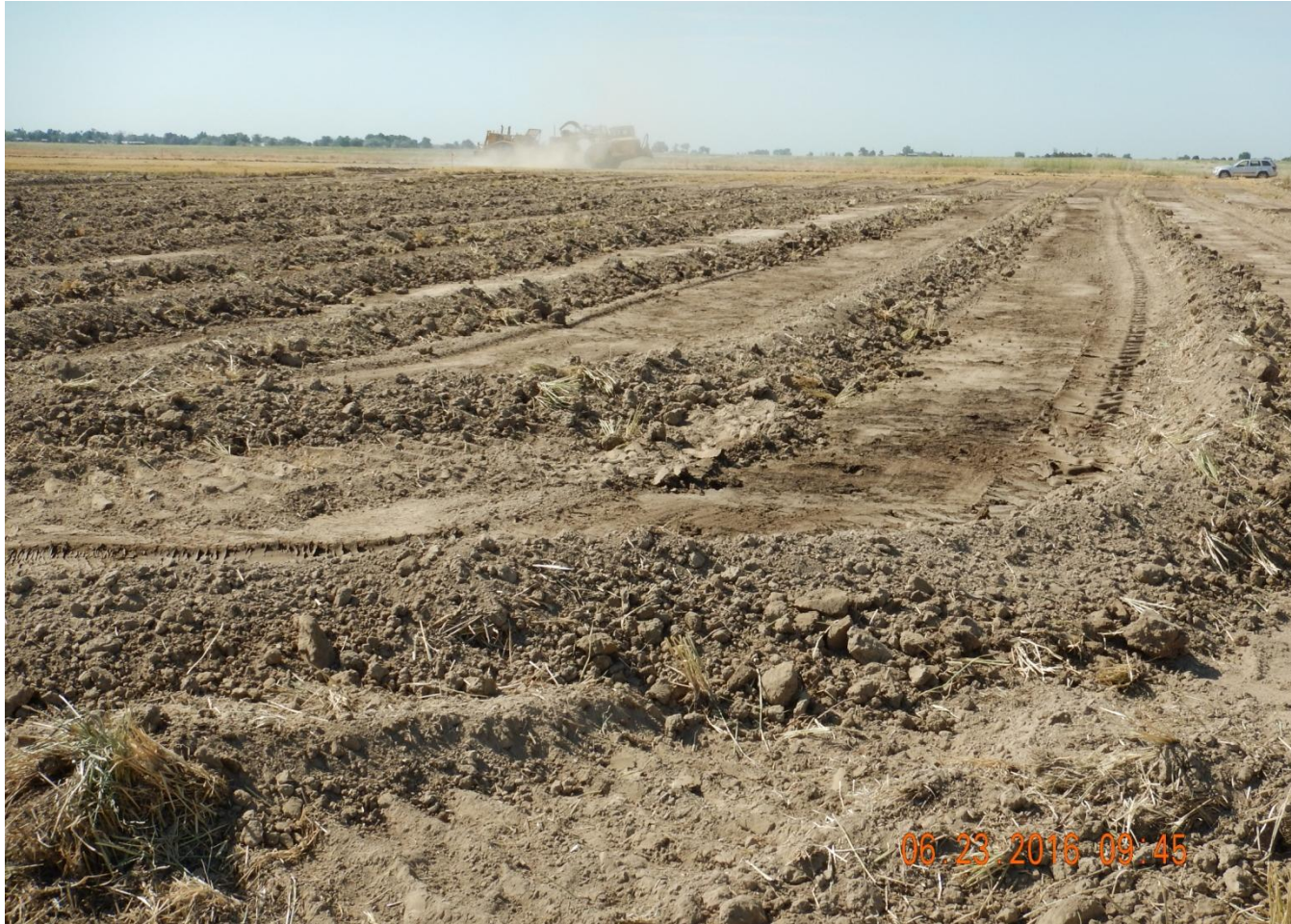
Photo 5. Photo taken from northern location, facing South. Topsoil salvage in process.
