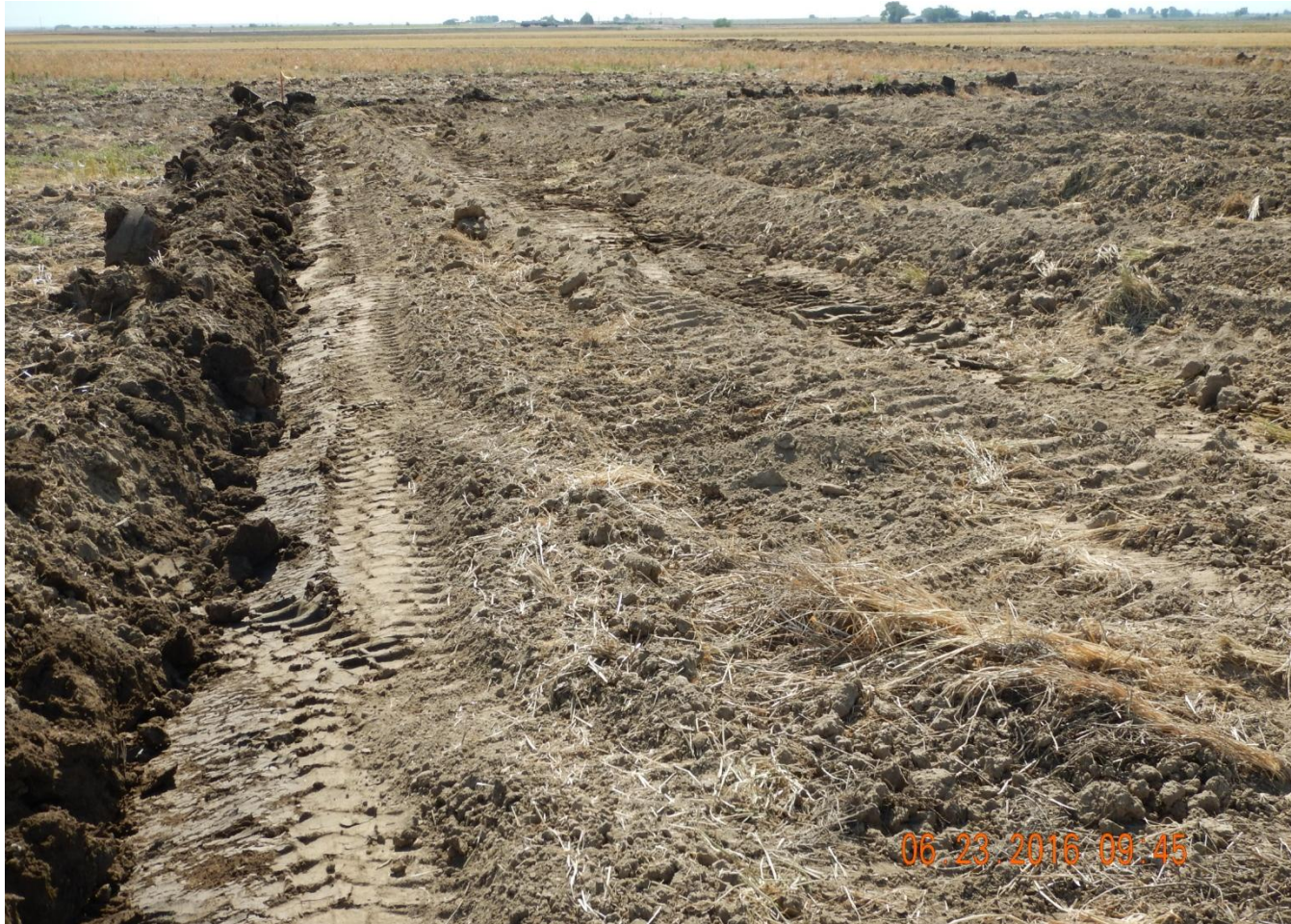
Photo 3. Photo taken from northwest location, facing East. BMP installed around perimeter of location. Operator said berms will be compacted and BMP would be finished on eastern side once landowner moves equipment.
