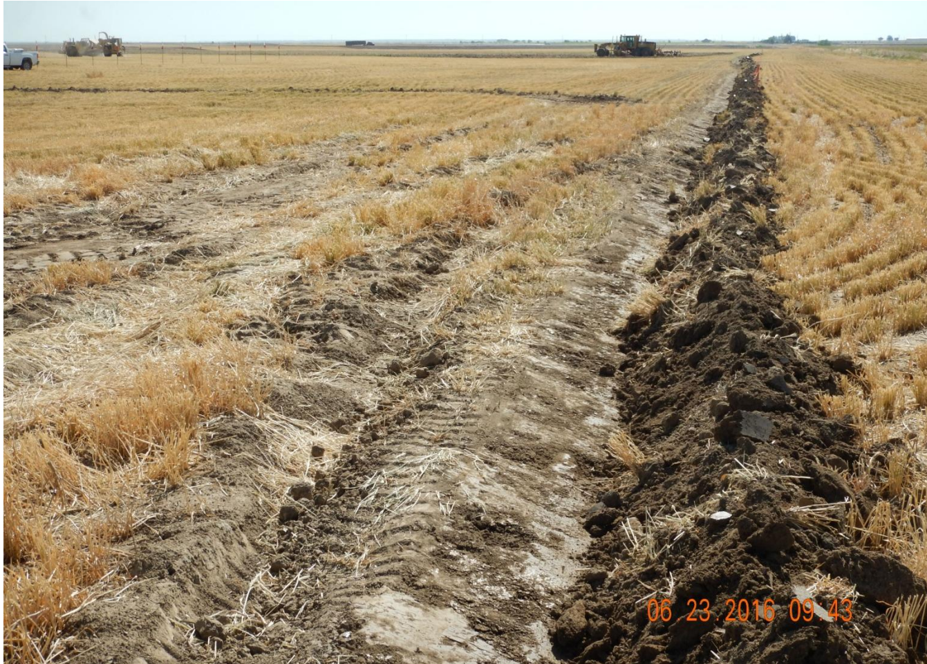
Photo 1. Photo taken from southwest location, facing East. BMP installed around perimeter of location. Operator said berms will be compacted and BMP would be finished on eastern side once landowner moves equipment.
