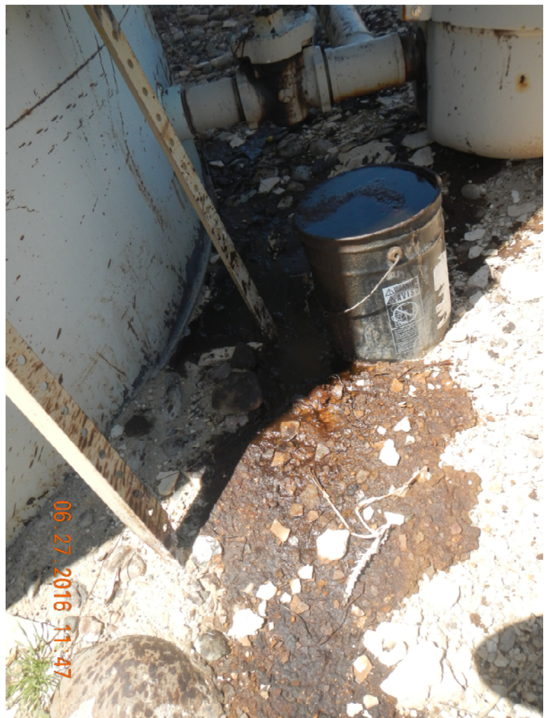
Overflowing bucket of fluid with sheen. Stained soil. Rodent skeleton. Adjacent to crude tank, inside berm.
