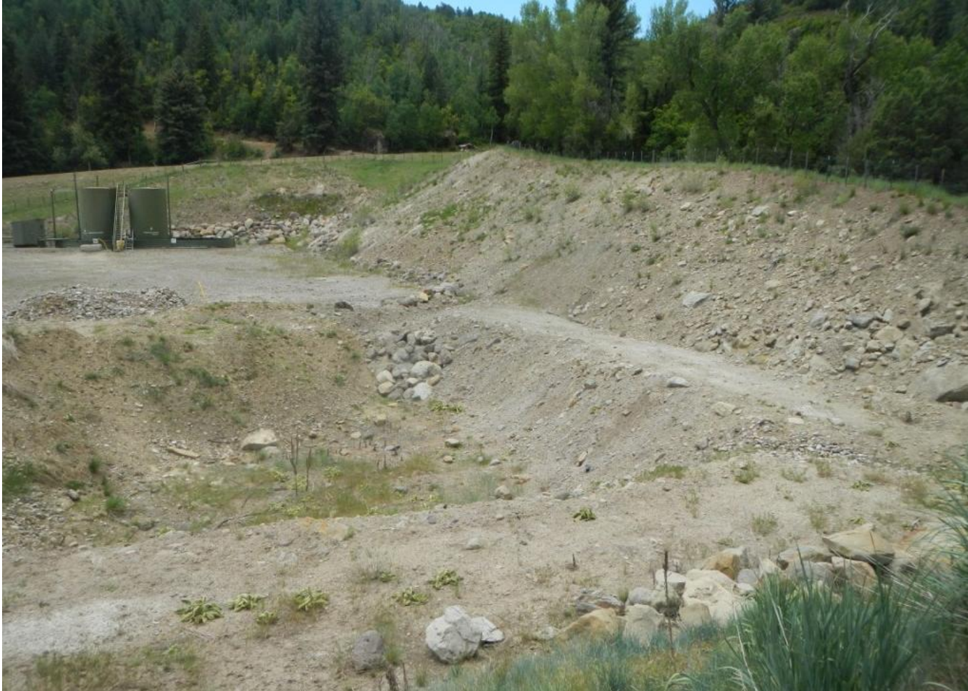
Photo 4. View of the western portion of the project area from the northwestern corner facing southward. It appears that old pit is being used as a large silt trap at this time.
