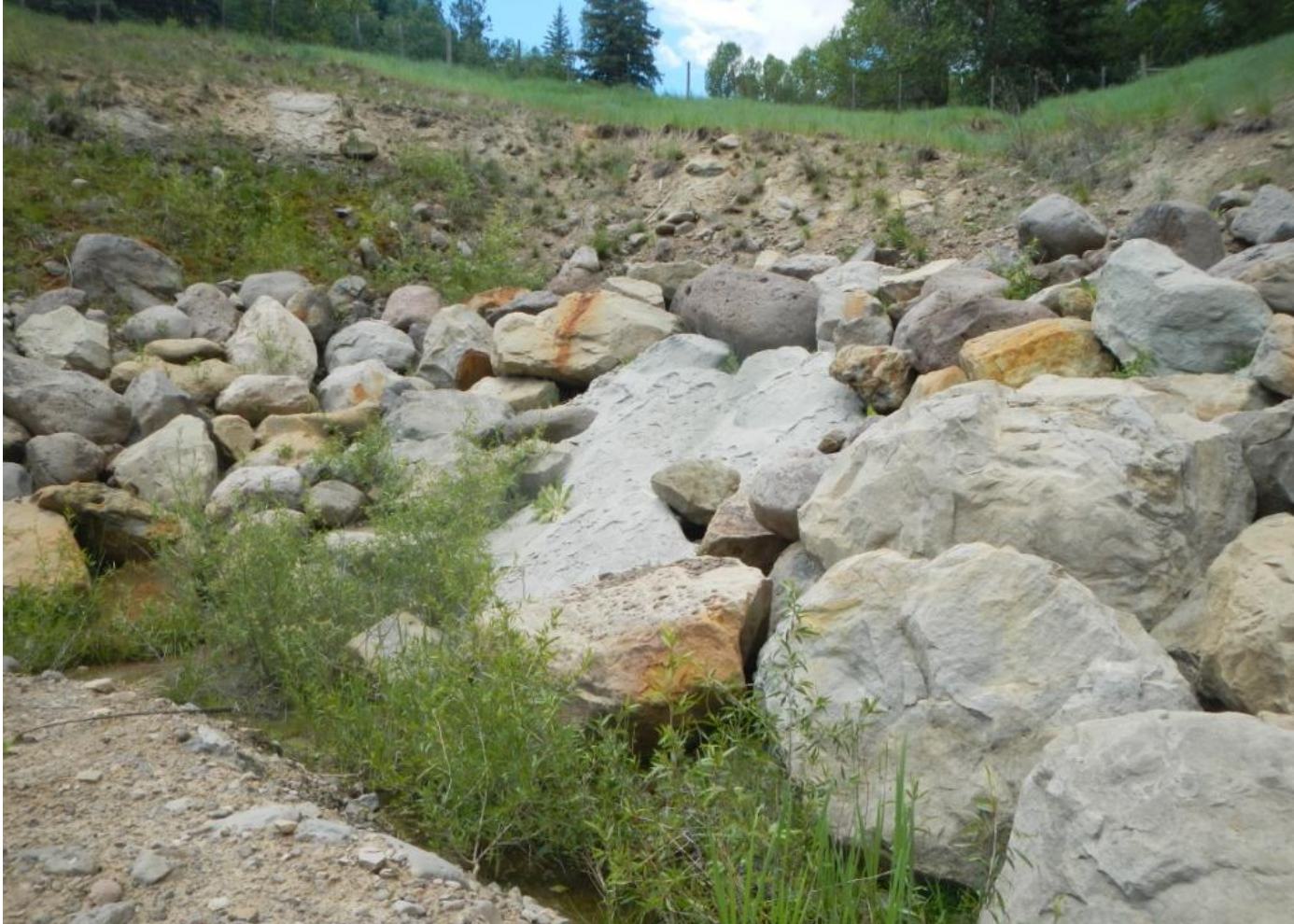
Photo 6. View of the southwestern corner of the project area facing up-slope. Large boulders are being used to stabilize slope. Water is emerging from cut-slope.
