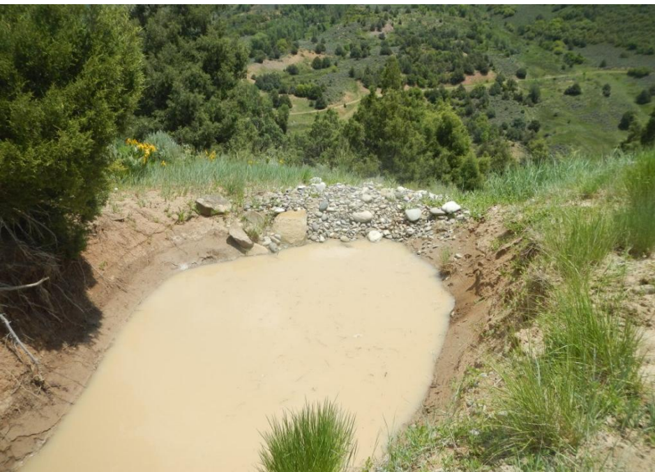
Photos 11 and 12. View of silt trap (on left) at turnout along access road. Photo on right shows silt trap overflow point that is stabilized at this time.
