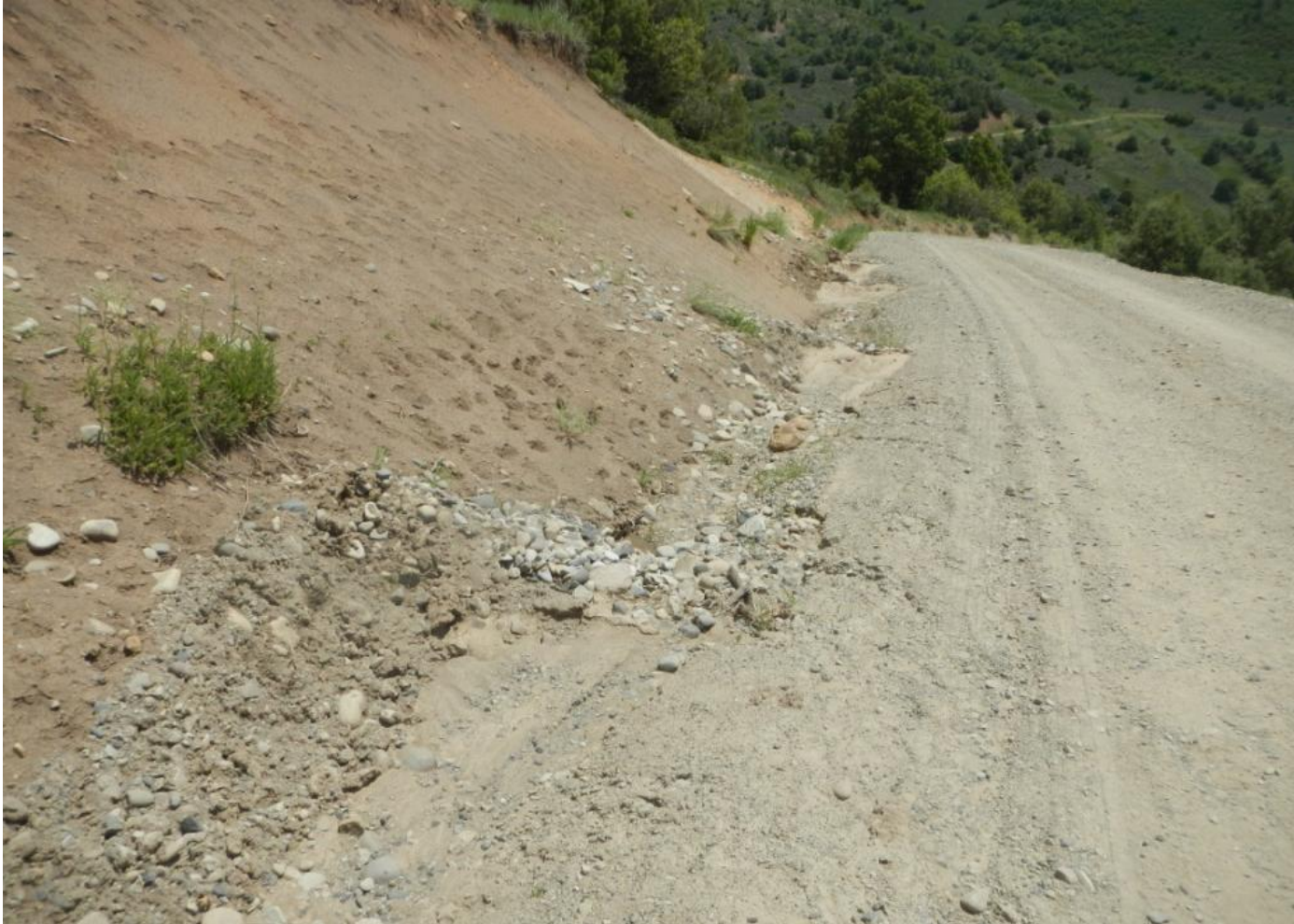
Photo 8. View of cobble check dams along steep section of access road. These appear to be properly sized and spaced. Sediment accumulation needs to be cleaned.
