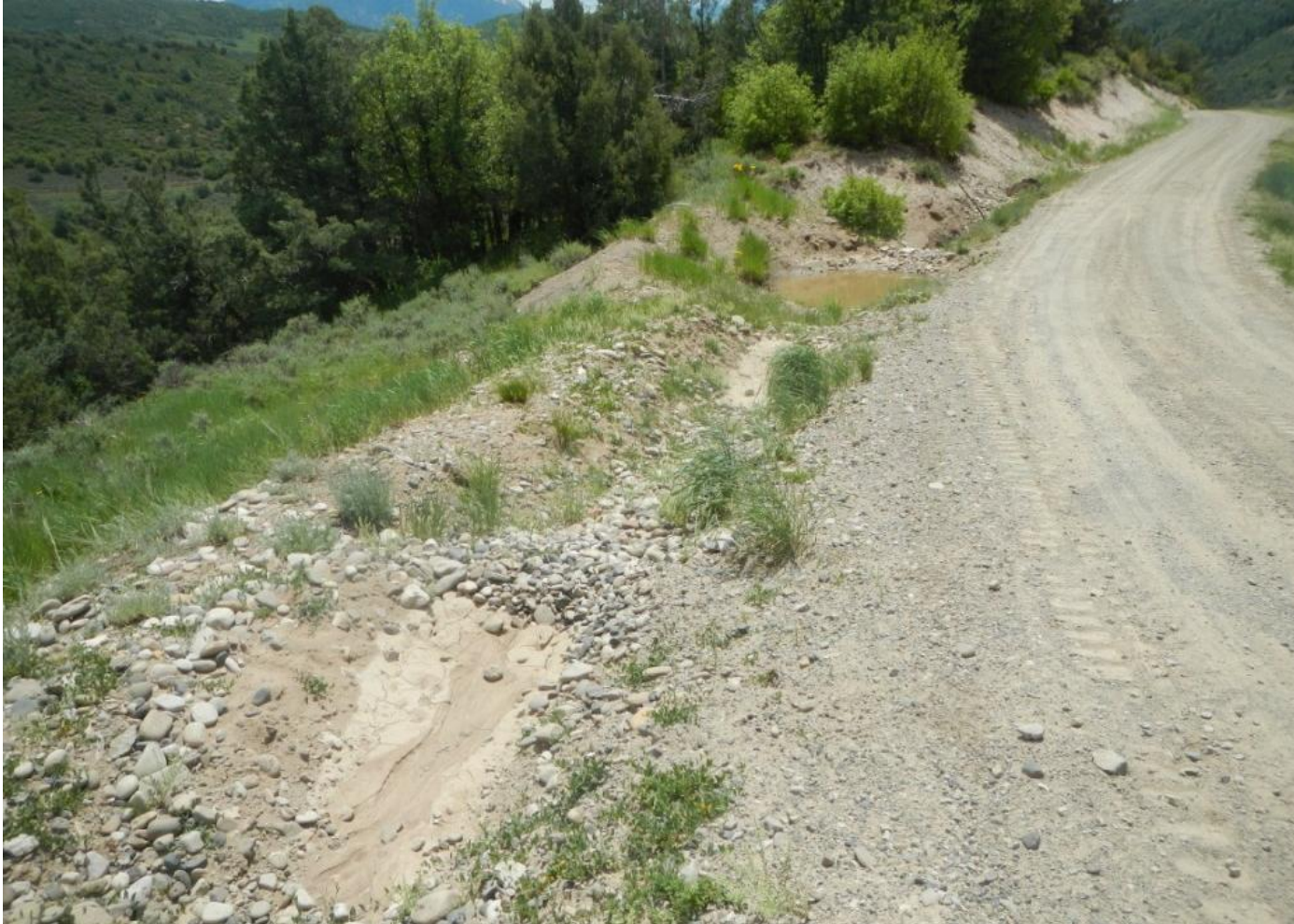
Photo 9. View of silt traps and culvert entrance along access road that appear to be functioning.
