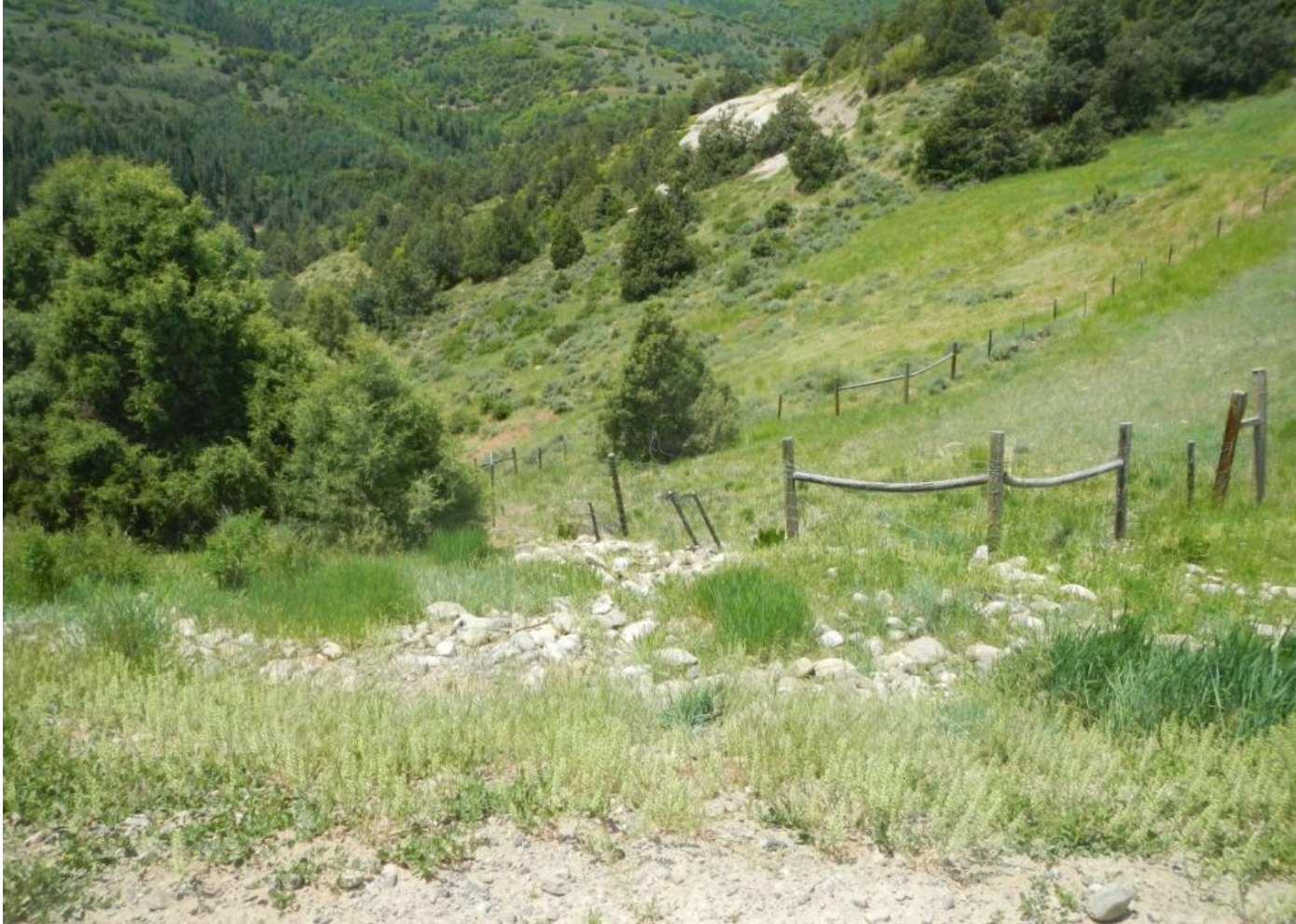
Photo 10. View of culvert outlet along access road draining westward. Outlet drain is armored and is stabilized at this time.
