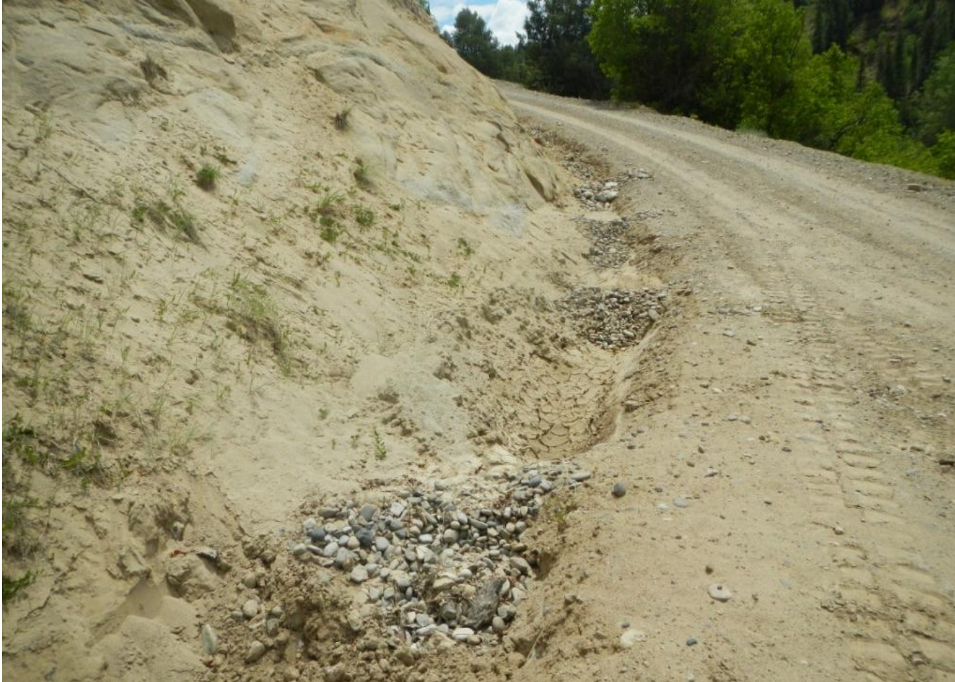
Photo 13. View of more cobble check dams near the bottom of the access road. These appear to be properly sized and spaced and will require frequent maintenance for silt accumulation.
