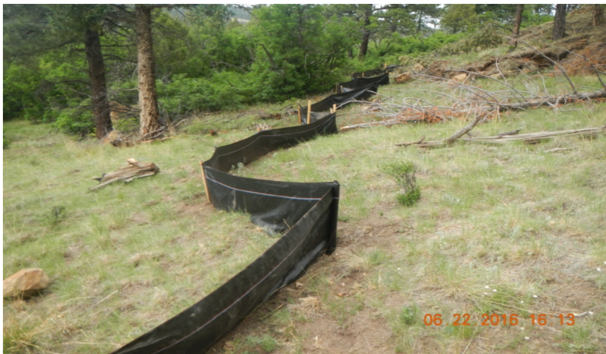
photo 5: A silt fence is installed at the west perimeter of the location.
