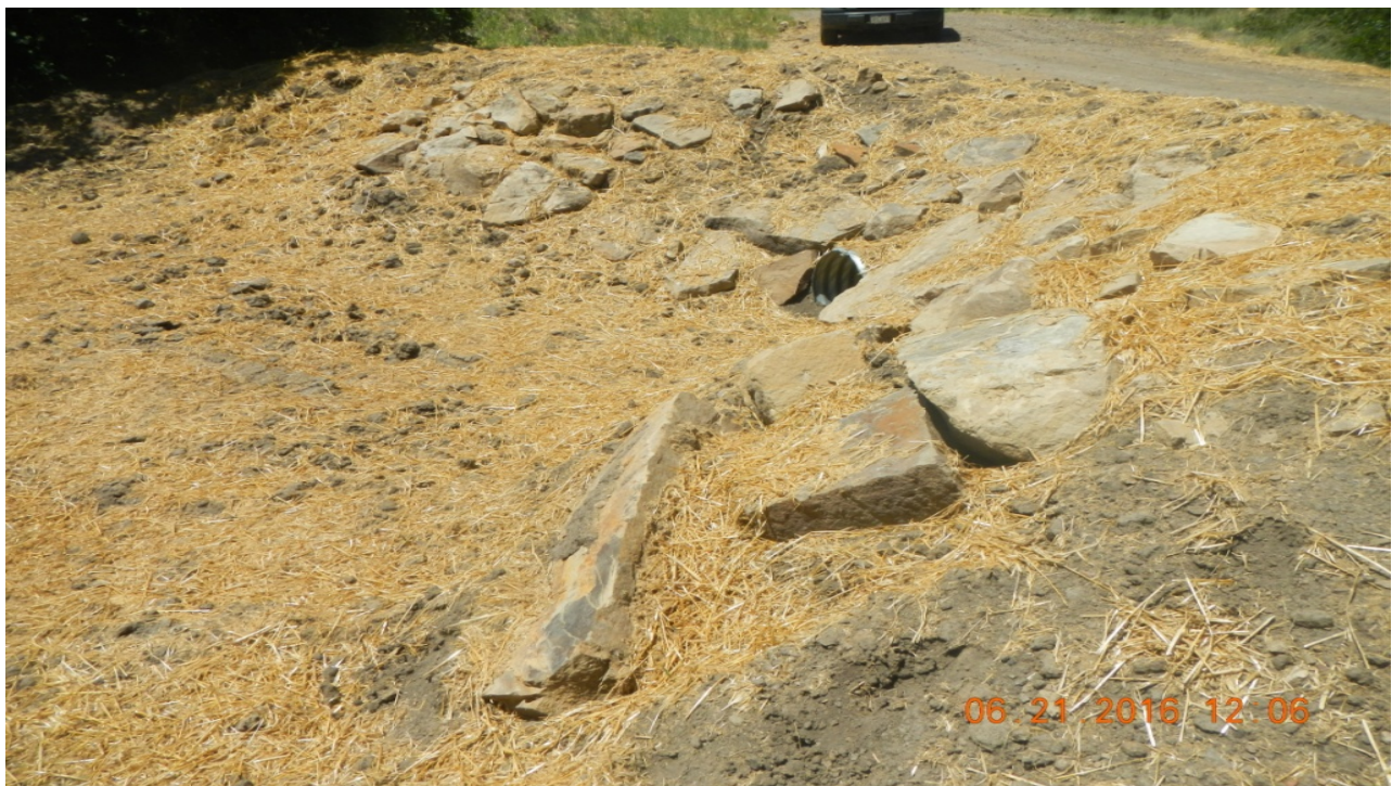
photo 2: Sediment has been cleaned out of culvert along the access road.
