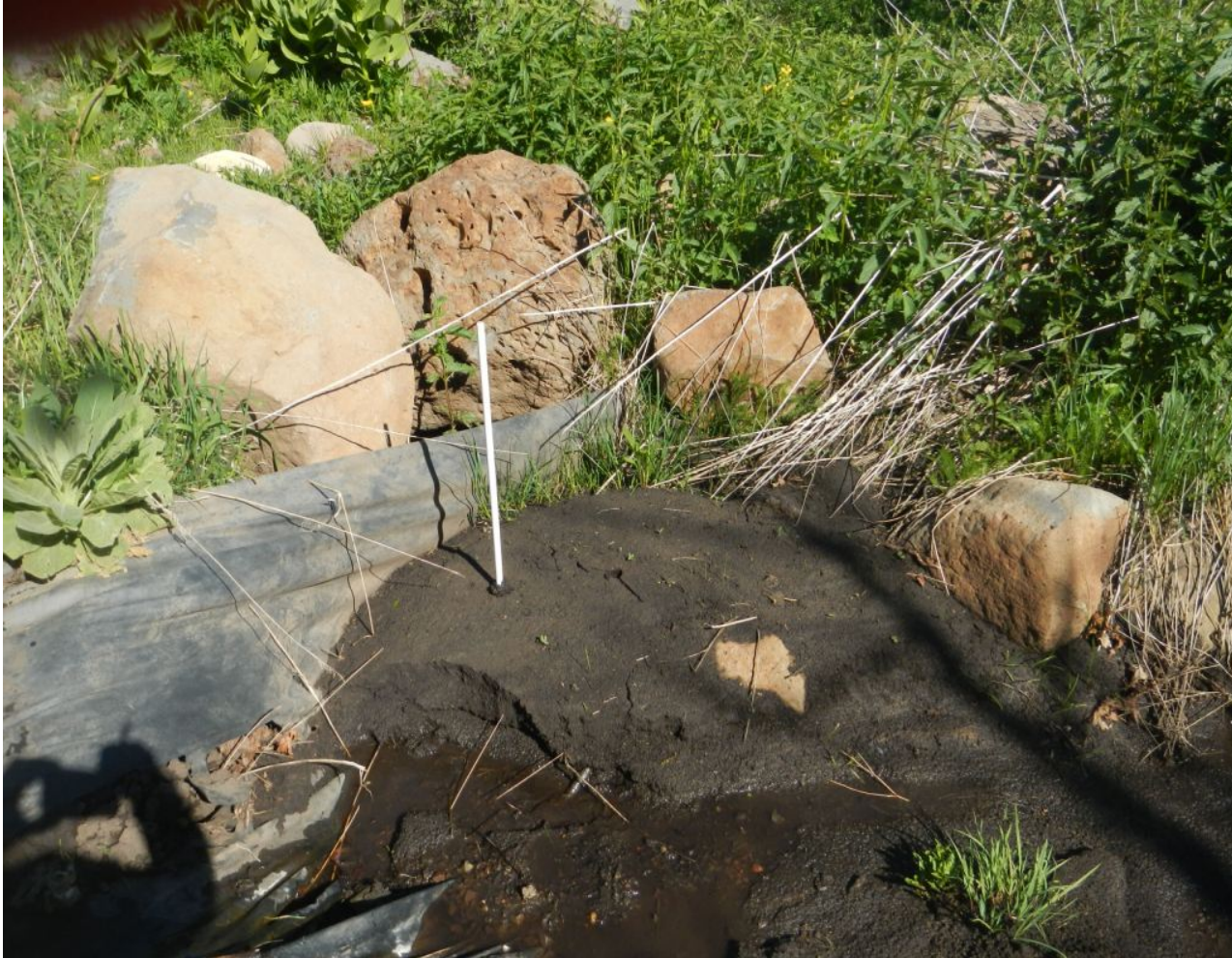
Photo#11: Sediment is Built up and allowing water to overwhelm ditch banks and flow to Cut Slope.
