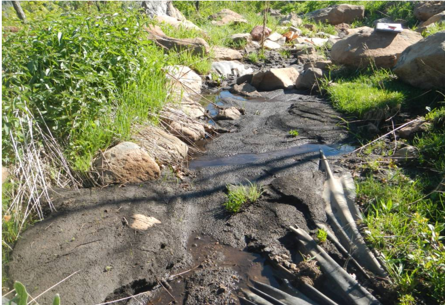
Photo#10: Sediment Build- Up is allowing water to overwhelm ditch banks and flow to Cut Slope.
