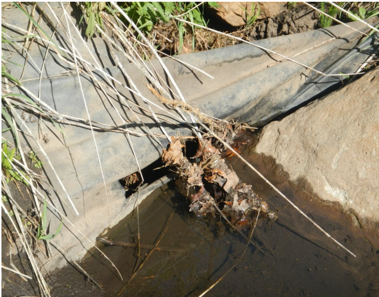
Photo#9: : Liner is failed at points & water undercuts ditch and drains to Cut Slope.
