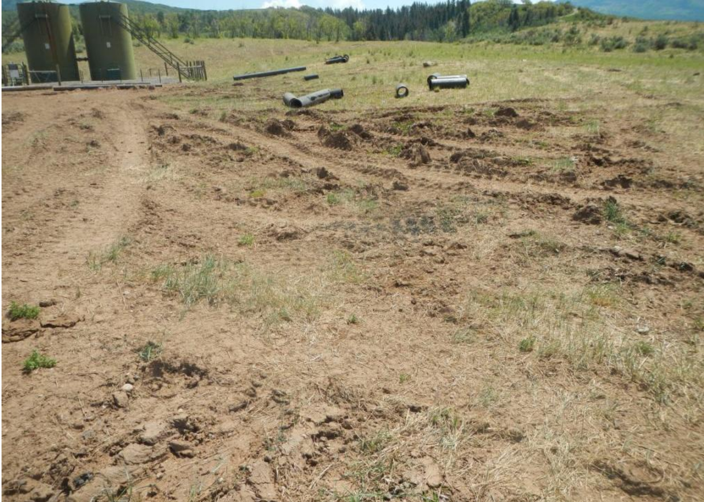
Photo 4. View of tire tracks, disturbed vegetation, and pipe debris in the southern portion of the project area. Tracked portions of the interim reclamation need to be seeded and reclaimed. Pipe and other debris needs to be removed.
