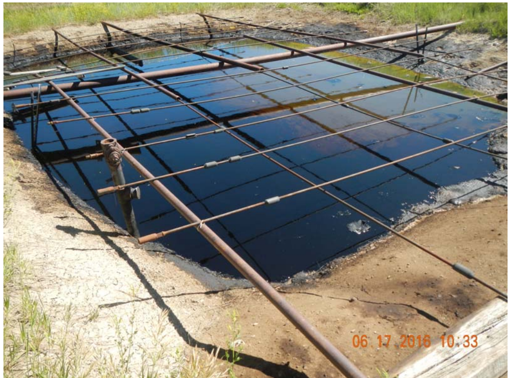
Pit without net. Water and product present in pit. 2 feet of freeboard not present.
