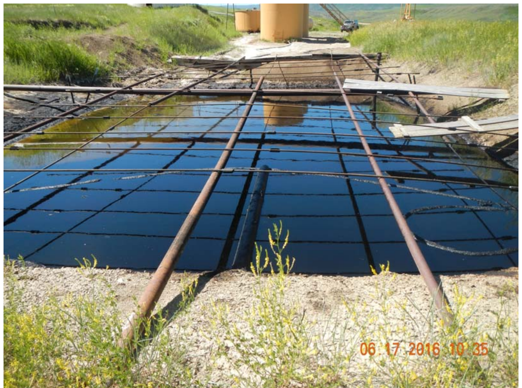
View of pit looking uphill towards wellhead and tanks.
