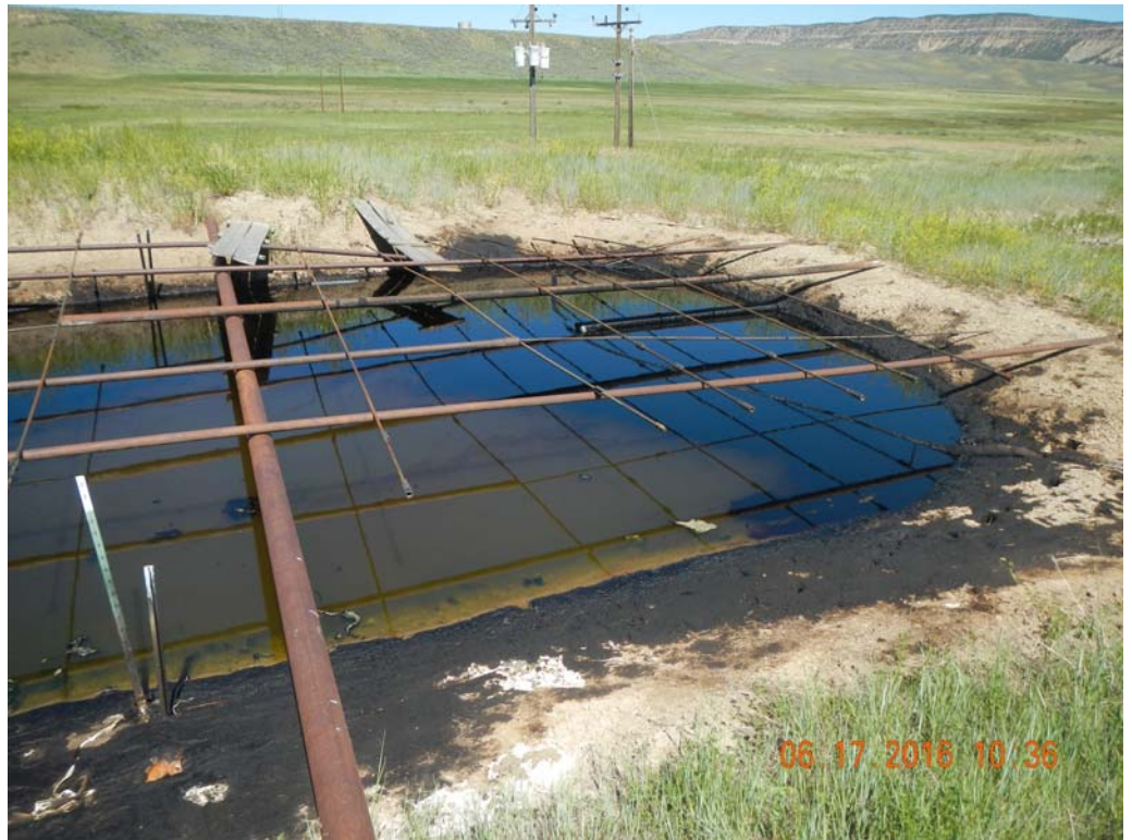
Pit without netting and without 2 feet of freeboard. Drainage ditch and stream visible in background.
