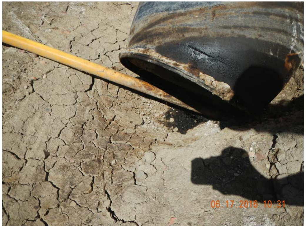
Stained soil below bucket below leak at tank loadout.
