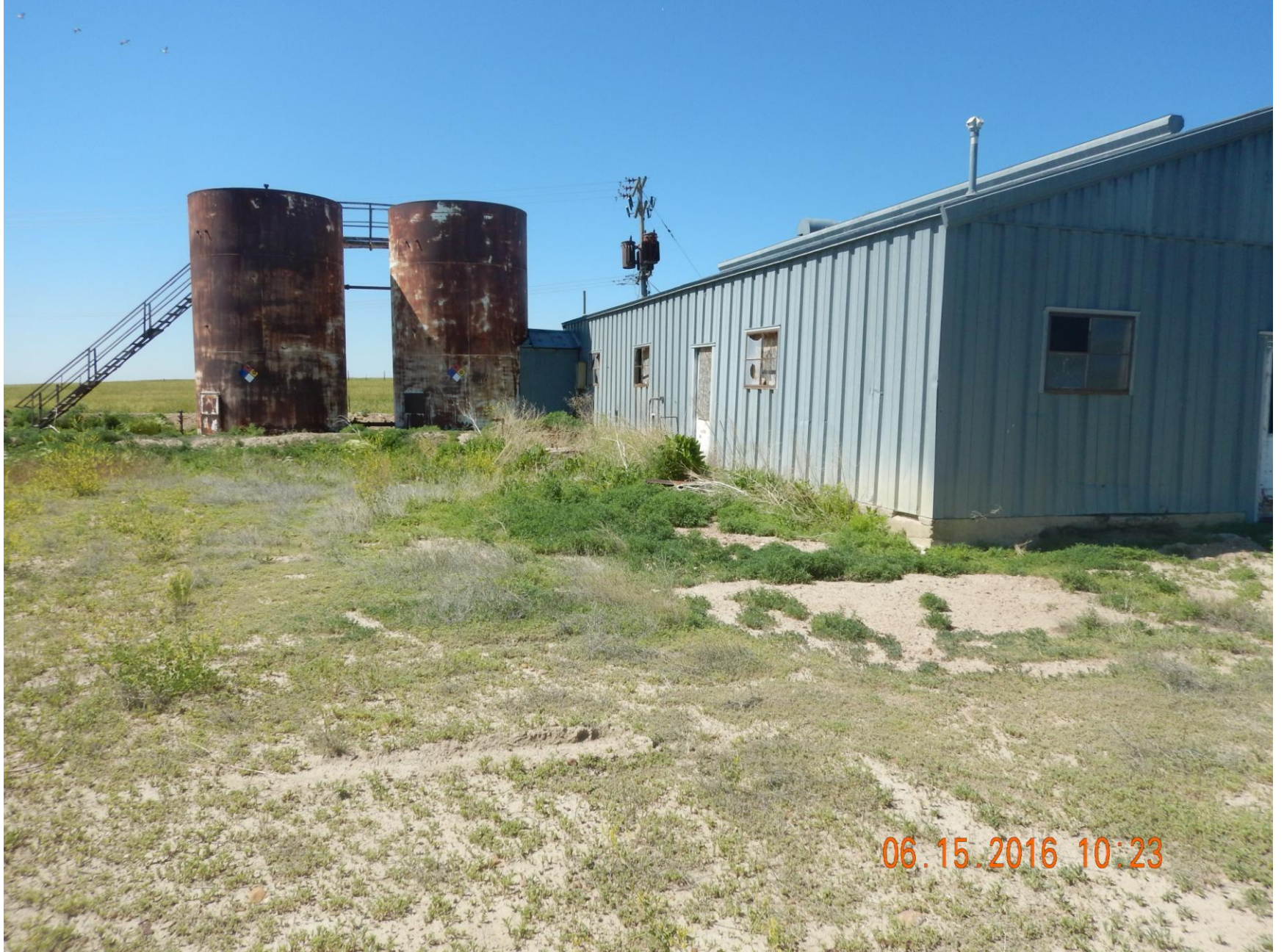
Figure 1: Photo taken from the southwest end of the location, facing south. Photo shows facilities on active location.
