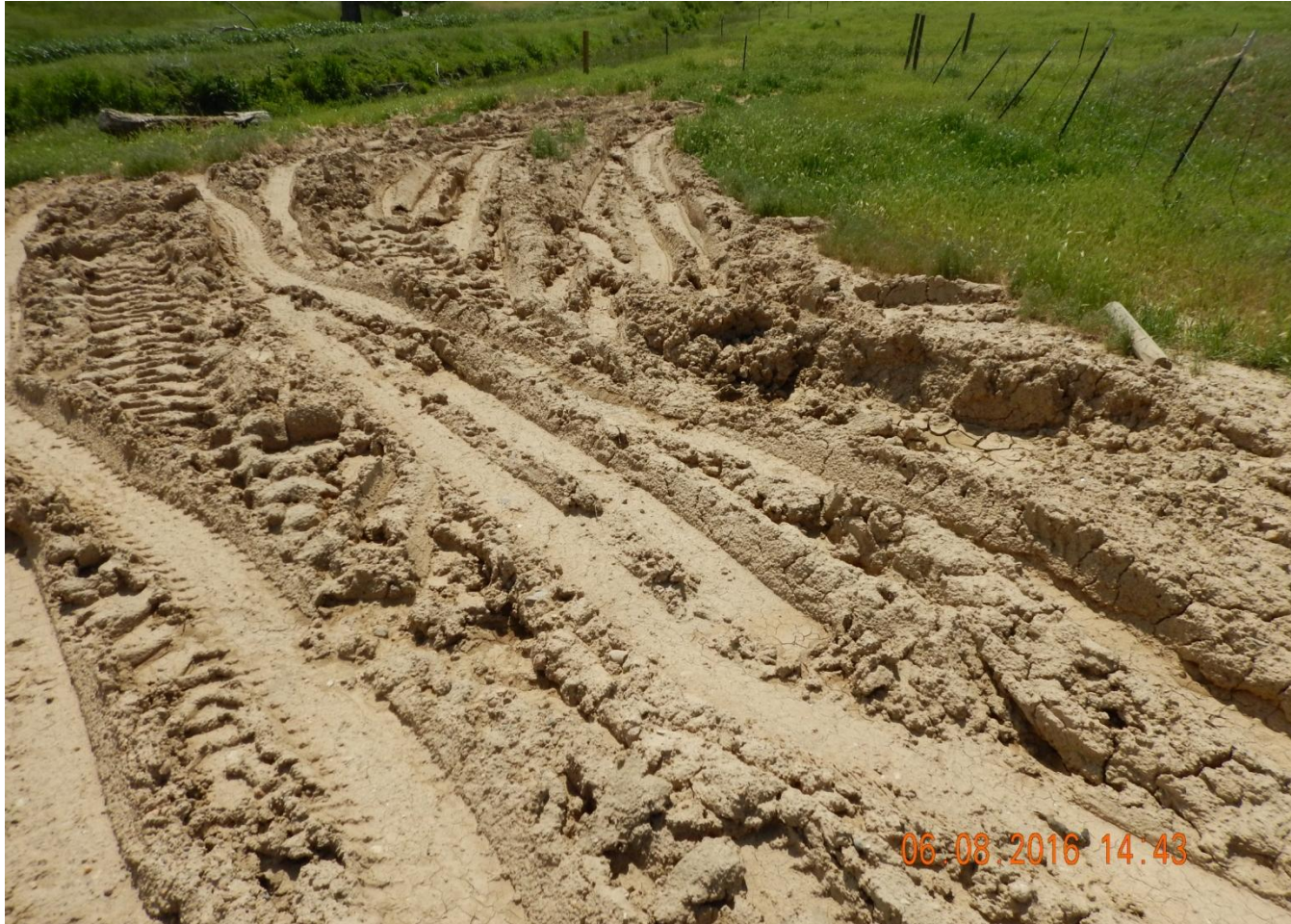
Photo 3. Photo taken from southwest of tank batteries, facing West. Need to maintain access road to prevent vehicle tracking and rutting.
