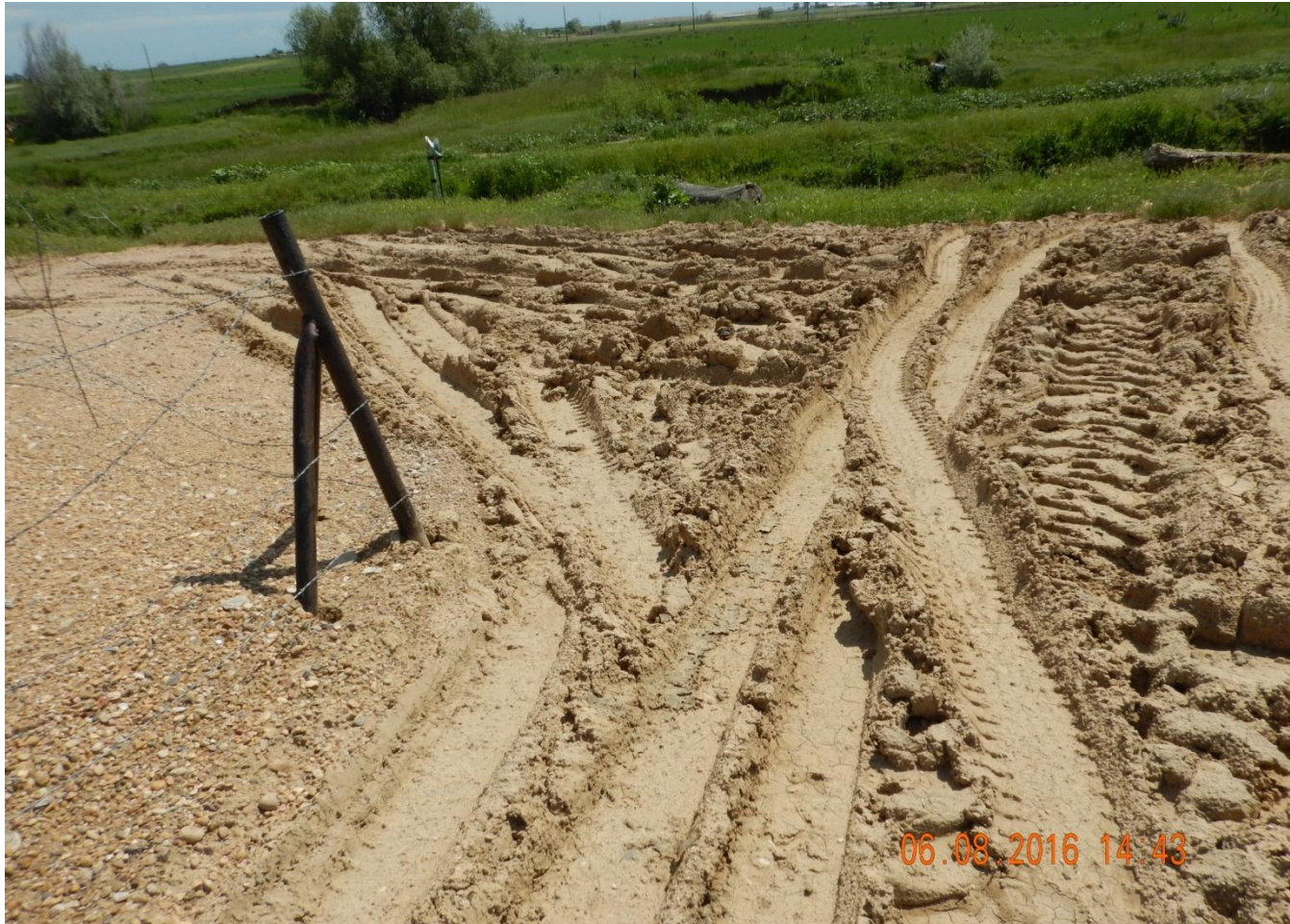
Photo 4. Photo taken from southwest of tank batteries, facing East. Need to maintain access road to prevent vehicle tracking and rutting.
