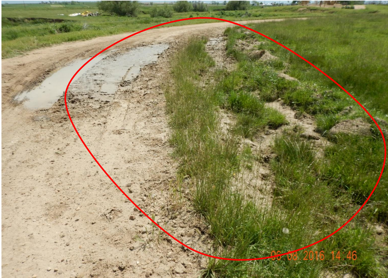
Photo 5. Photo taken north of tank batteries, facing South. Access road was widened. Need to repair access road and reseed portions that will be disturbed. Reseeding may have to wait until the Fall when more favorable conditions are permitted.
