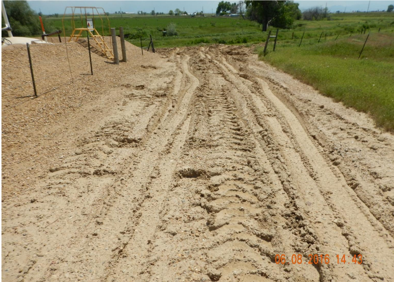
Photo 2. Photo taken from west of tank batteries, facing South. Need to maintain access road to prevent vehicle tracking and rutting.
